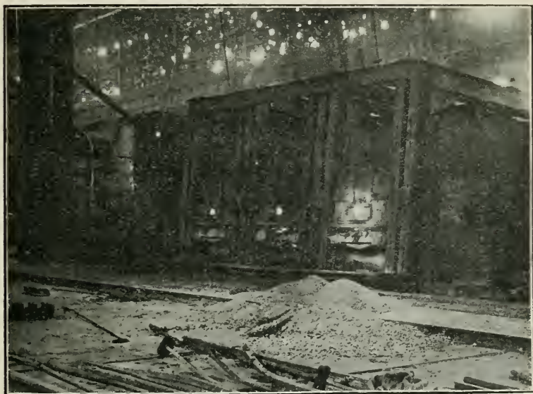
FRONT VIEW OF FURNACE.
