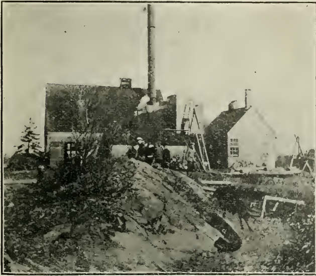
STERLING SHAFT HOUSE.
