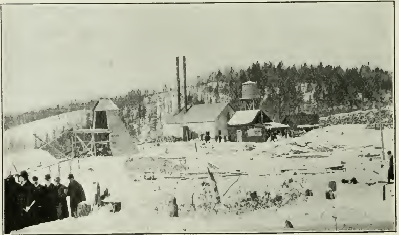
Shaft House and Buildings at the Foster.
