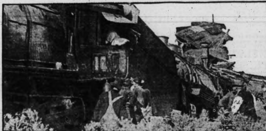
WHAT ONE SMALL BOY CAN DO. —When a small boy took a rock and broke a switch lock on a Montana railroad he caused this smashup, in which five persons were killed. Photo shows rescuers trying to extricate the engineer, who died shortly after being freed.
