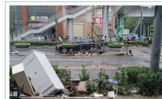
Songshan Road in Zhengzhou, damaged by the floods.
