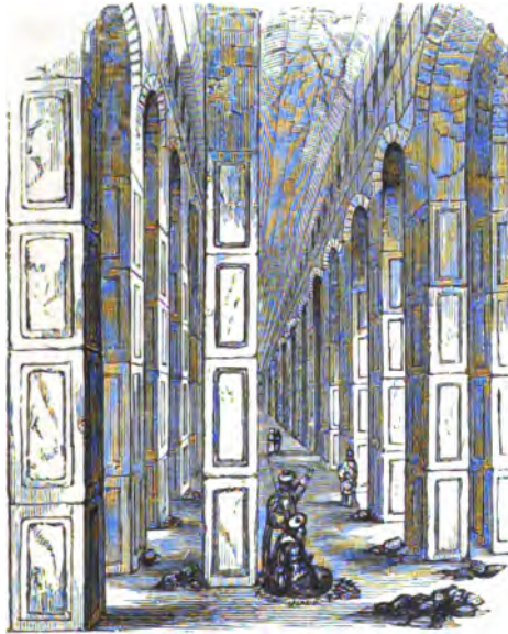
Underground Buildings in the south-east corner of the Haram es Sherif.
