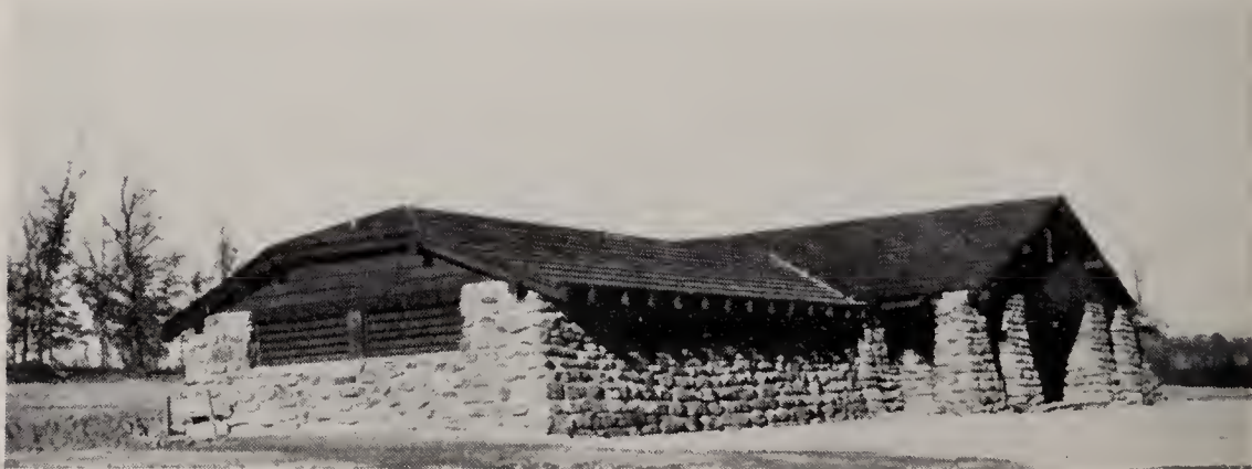
The bathhouse on Wedington Lake, built entirely of native materials from the project area. The boat house, administration building, and other structures are similar in design and construction
