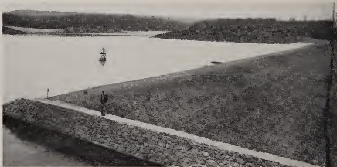
Wedington Lake, looking northwest from the dam and spillway. At the foot of the dam is the 5-acre tree nursery of the project, irrigated from the lake. Planting and other development was not complete when this picture was made
