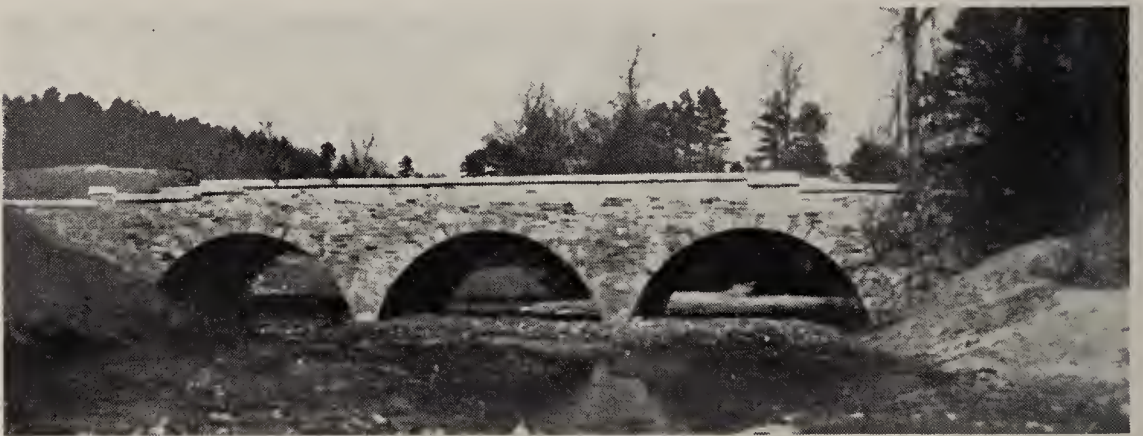
Spanning Six Mile Creek, this triple-arched bridge on the Park Road was constructed entirely by relief labor, and largely with native materials
