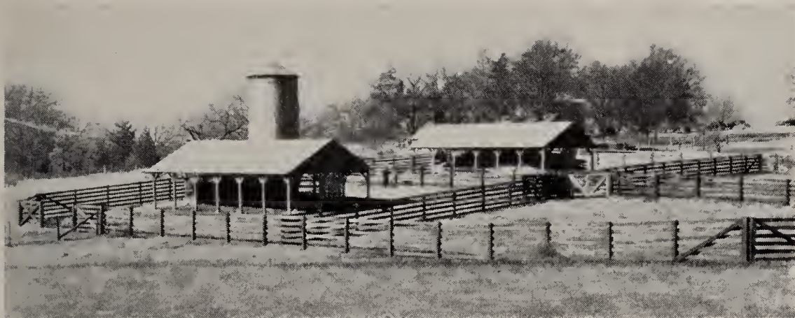
These corrals have been built for the sheltering, feeding, and examination of the cattle that will be run on the project's 2,200-acre improved pasture
