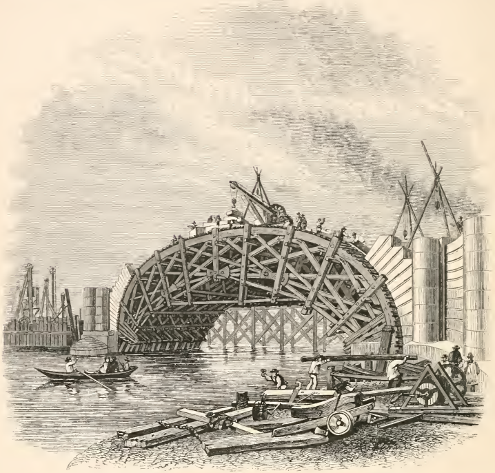
CENTERING OF ARCH, WATERLOO BRIDGE. [After E. Blore.]
