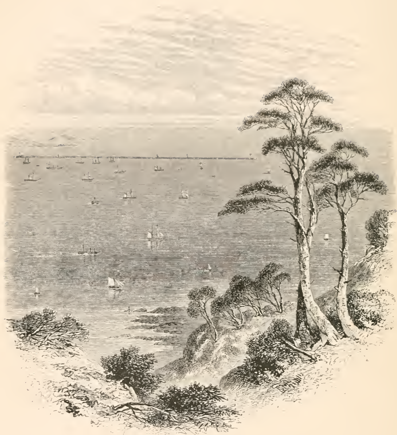
VIEW OF THE BREAKWATER FROM MOUNT EDGCUMBE.
