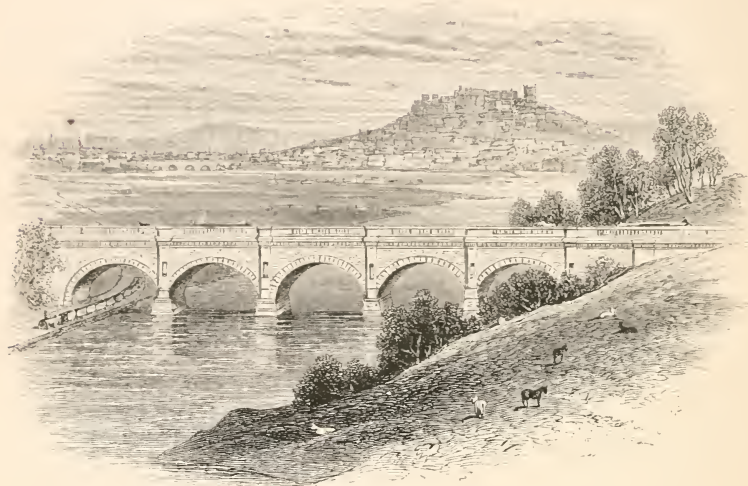
LUNE AQUEDUCT, NEAR LANCASTER.
