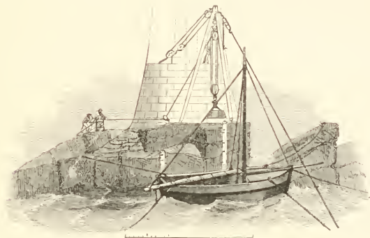
PROGRESS OF THE WORKS TO THE 15TH COURSE.
