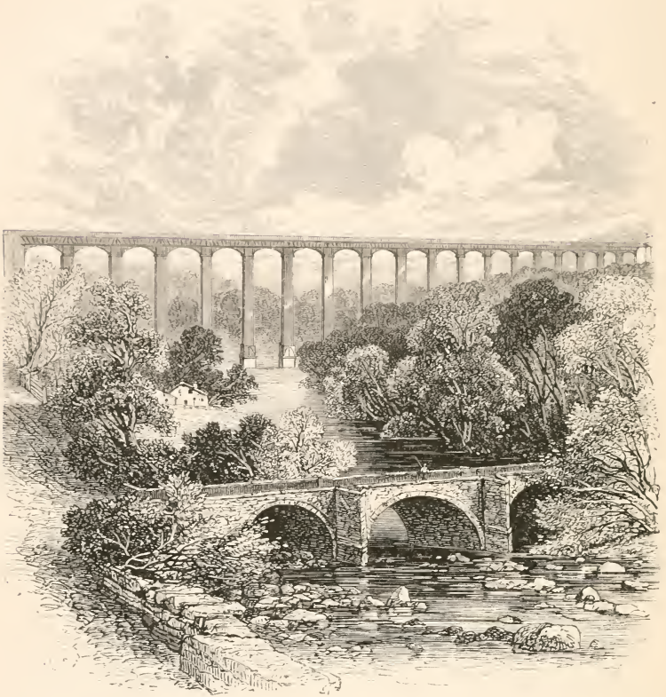
VIEW OF PONT-CYSTLLEN AQUEDUCT.
