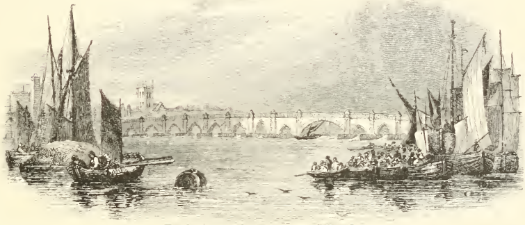
OLD LONDON BRIDGE AFTER THE REMOVAL OF THE PIER.
