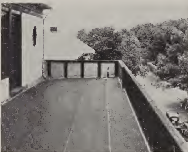
Cotton used as a decking material on porches.
