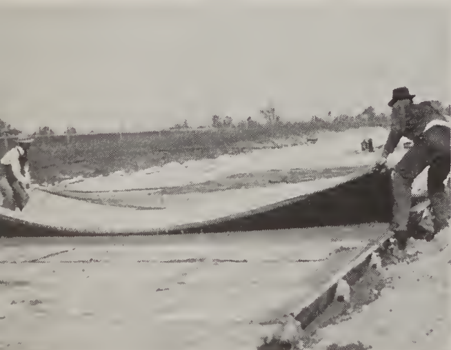
Cotton-curing mats aid in the curing process of concrete-highway construction.
