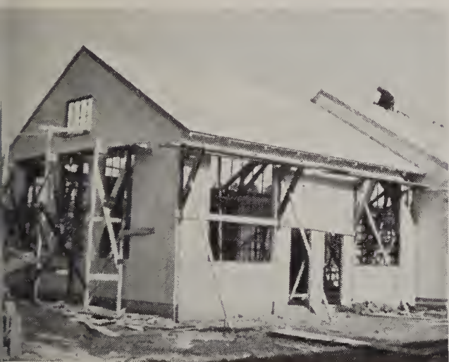
Durable and lasting cotton fabric used as side wall and roof material.
