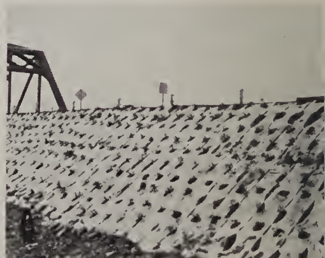
Cotton fabric keeps shrubs in place until firmly rooted along highways.
