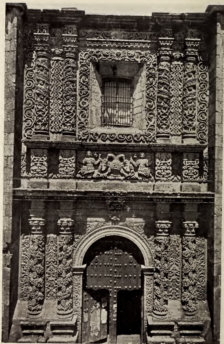
Plateresque Façade of the old convent church of Santa Monica at Guadalajara.
