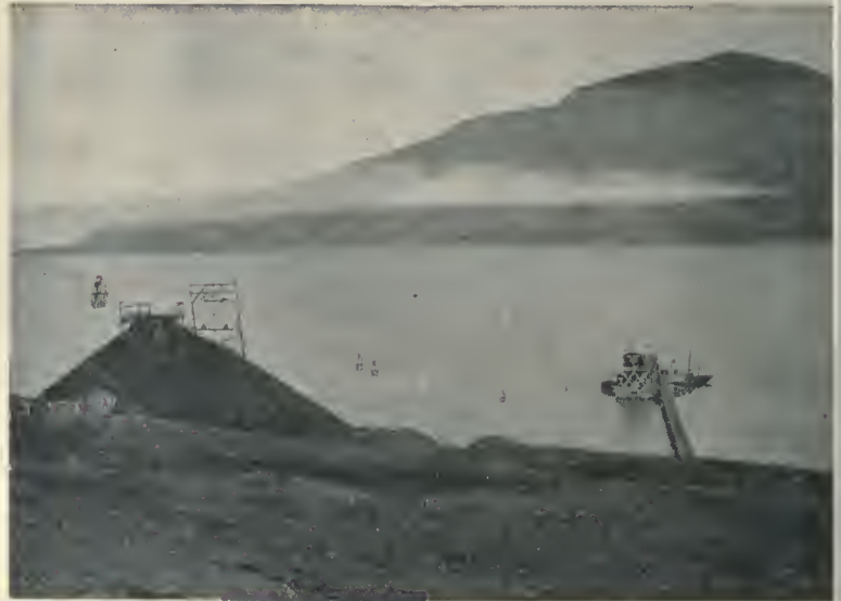
FIG. 2.—Longyear Mine, Advent Bay. Wire ropeway from the mine, coal dump, and jetty with a vessel loading alongside. From "Spitsbergen."
