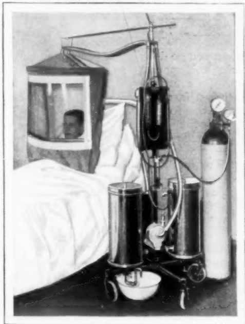
For Beneficial Oxygen Treatments While in Bed: Portable Outfit with Its Tanks, Cooler and Filter
