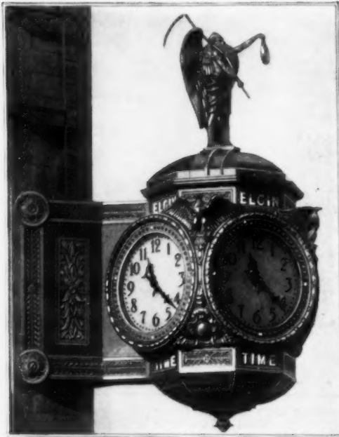
© E. L. Fowler Twenty-Foot Bronze Clock That Is Kept Timed Electrically with Observatory Thirty-Five Miles Away
