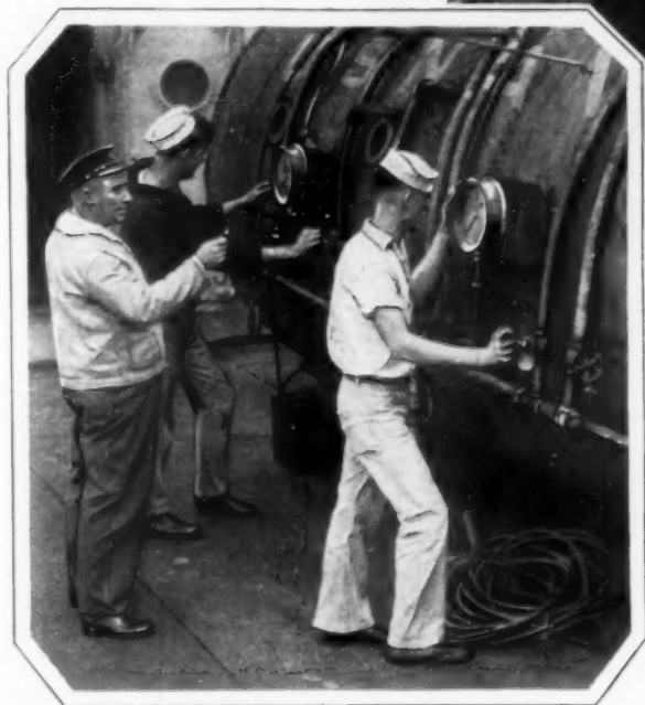
Assisting a Diver from the Pressure Tank after Treatment to Prevent the "Bends," and, at Left, Sailors on Duty at the Tank Controls, Slowly Lowering the Air Pressure in Its Interior
