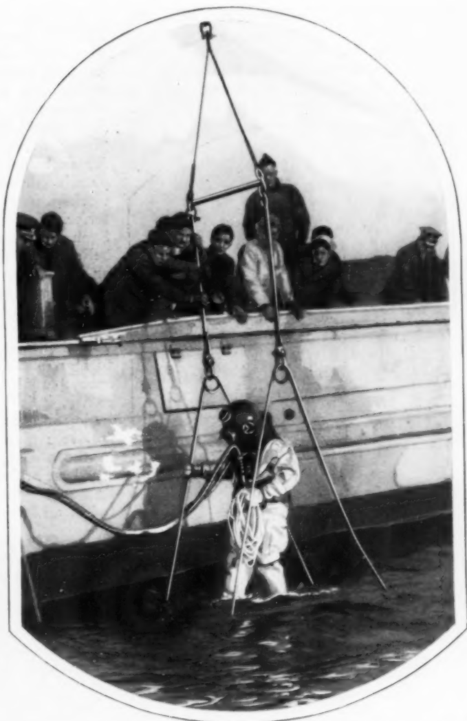
Lowered over the Side on a Platform, a Navy Diver Starts Down to the "S-4," to Attach Air Lines in an Unsuccessful Rescue Attempt
