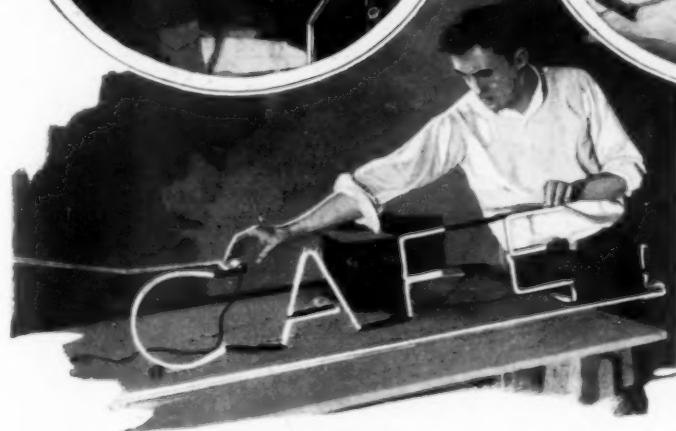
Left, Admitting Gas into the Tube; Above, Bending Tubing into Form of a Letter, and a Finished Word Assembly
