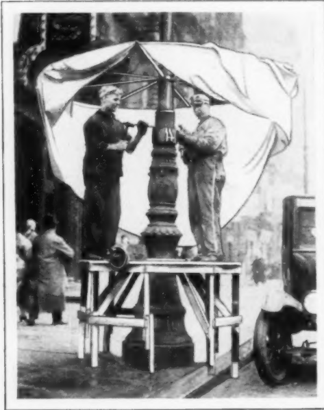
Portable Tent to Shield Pedestrians, with Side Raised to Disclose Workmen
