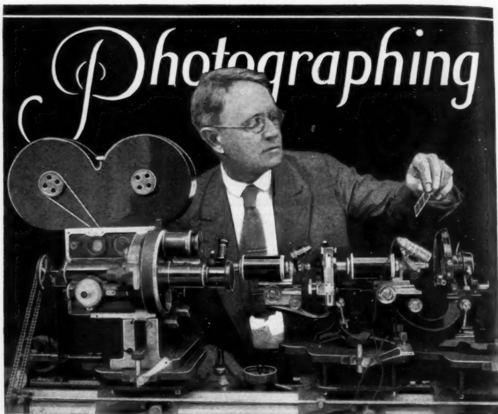
This Slowest of Slow-Motion Cameras Will Take One to Thirty Pictures a Week, Magnifying the Object as Much as 100,000 Times; It Is Geared to a Motor
