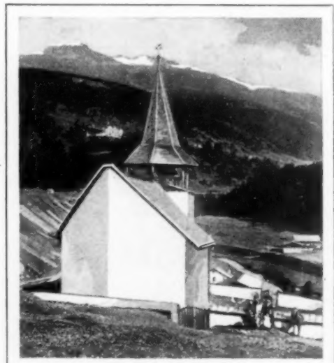
With Its Back to the Hills to Hold Landslides in Check; Swiss Church That Protects Village
