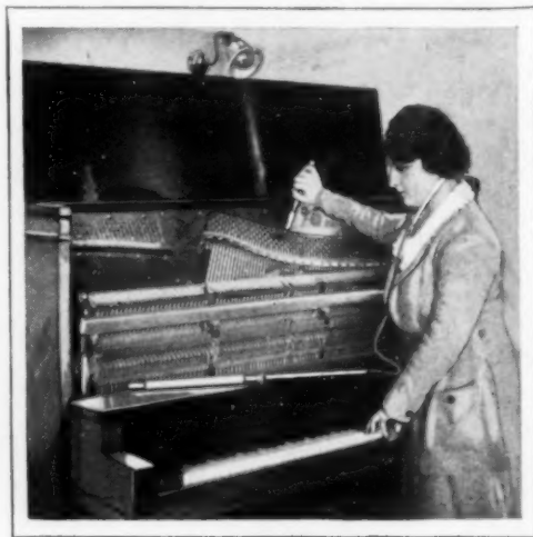
Tuning a Piano with Aid of Gauge. Seen on Shelf above the Keys; It Accurately Measures Sound
