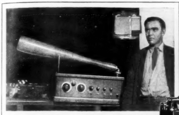
Joe Sullivan, of Toledo, with His Home-Grown Loud Speaker; He Collects Gourds, Removes the Seeds and Then Thoroughly Dries the Gourd, after Which a Loud-Speaker Unit Is Fastened to the Small End
