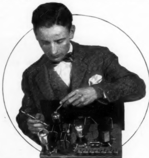
This View Indicates the Position of the Added Transformer and Tube
