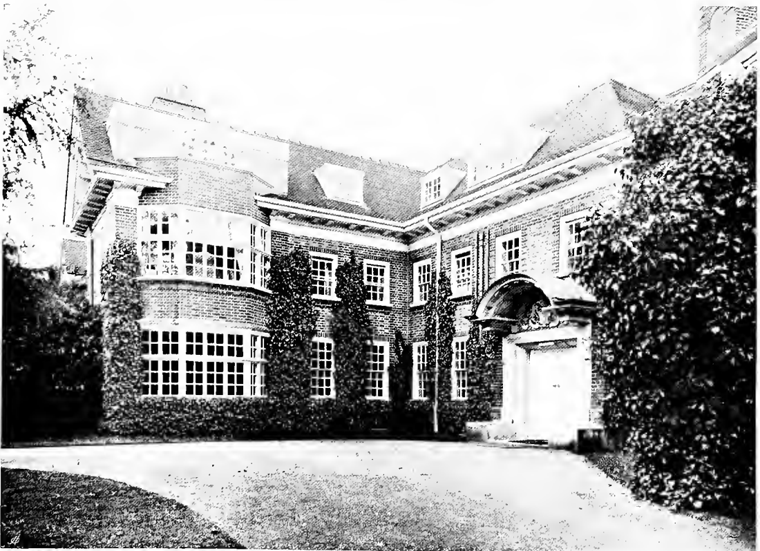
SHOOTER'S HILL HOUSE, PANGBOURNE, BUILT OF GREY BRICKS WITH RED BRICK FACINGS. THE HOUSE HAS A TILED ROOF, A STONE DOORWAY, AND A CORNICE OF WOOD B13
