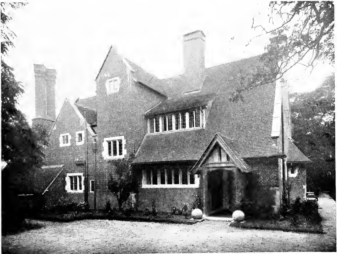
THE GARDEN FRONT, WOODGATE, FOUR OAKS. IT IS ROOFED WITH DARK TILES AND BUILT OF MULTI-COLOURED THIN BRICKS
