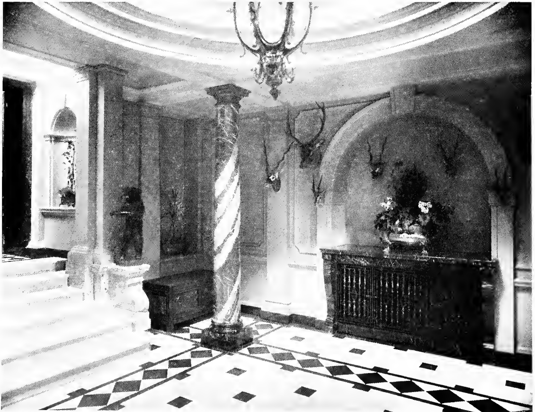
E14 VIEW OF THE LOWER ENTRANCE HALL AT JARDINE HALL, DUMFRIESSHIRE, THE FOUR COLUMNS ARE OF CAMPAN MELANGE MARBLE WITH BLACK BASES AND CAPITALS. THE FLOOR IS OF BLACK AND WHITE MARBLE AND THE WALLS ARE PAINTED
