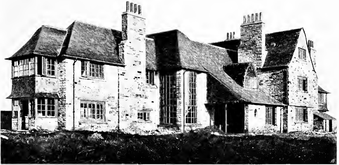
HOUSE AT ST. ANDREWS BELONGING TO CHARLES E. TODD ESQ. IT IS BUILT OF LOCAL STONE AND THE ROOFING IS COMPOSED OF MIXED SLATES FROM EASDALE, CRAIGLEA AND BALLACHULISH
