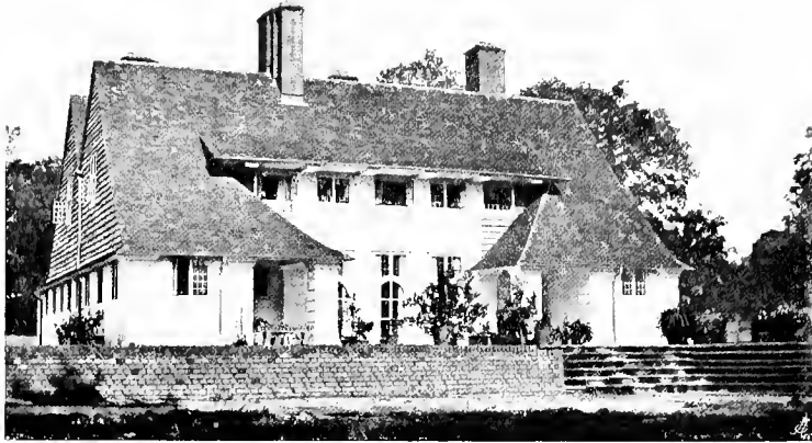
HOMWOOD, KNEBWORTH, HERTFORDSHIRE, THE SEAT OF THE DOWAGER COUNTESS OF LYTON. MATERIALS: TILES FOR THE ROOF AND BRICK AND WOOD FOR THE WALLS. SOUTH-EAST SIDE
