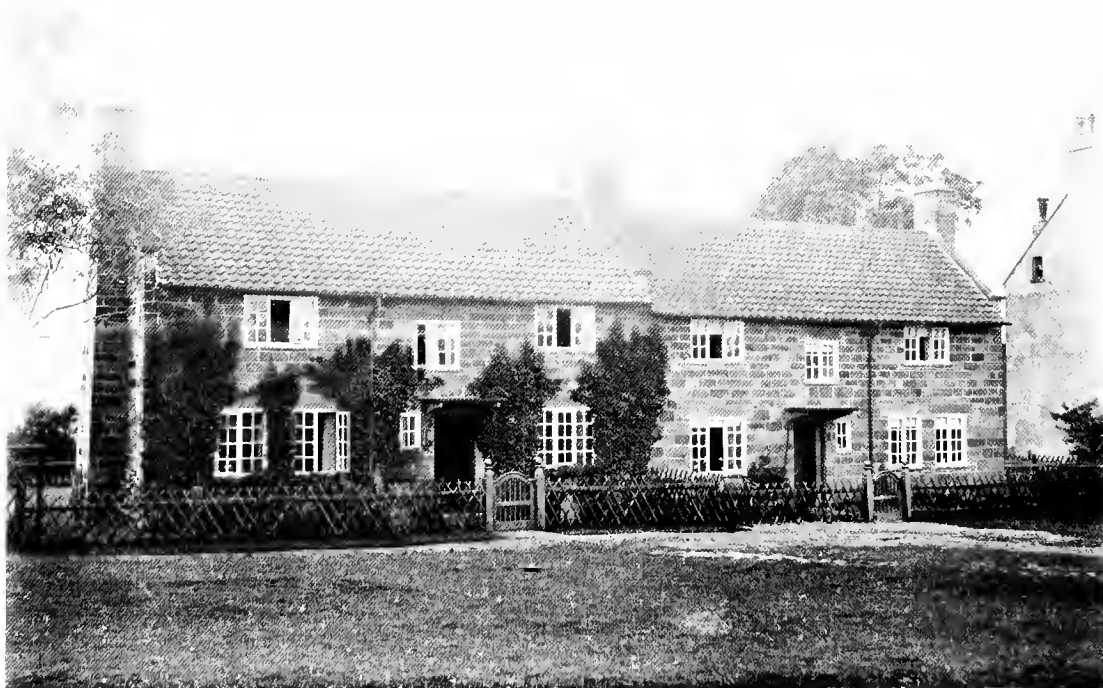
TWO COTTAGES AT GOATHLAND, BUILT OF LOCAL MATERIALS AT A COST OF £650 FOR THE PAIR, EACH COTTAGE HAS TWO SITTING ROOMS AND FOUR GOOD, AIRY BEDROOMS
