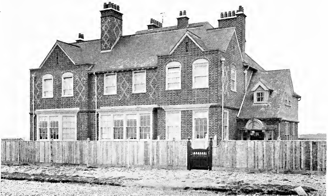
SANDYCROFT, LITTLESTONE-ON-SEA, BUILT FOR THE RIGHT HON. HERBERT J. GLADSTONE, M.P. MATERIALS: DARK RED BRICK FACINGS, BROWN TILE ROOF, THE WINDOW FRAMES AND THE WOODWORK PAINTED WHITE
