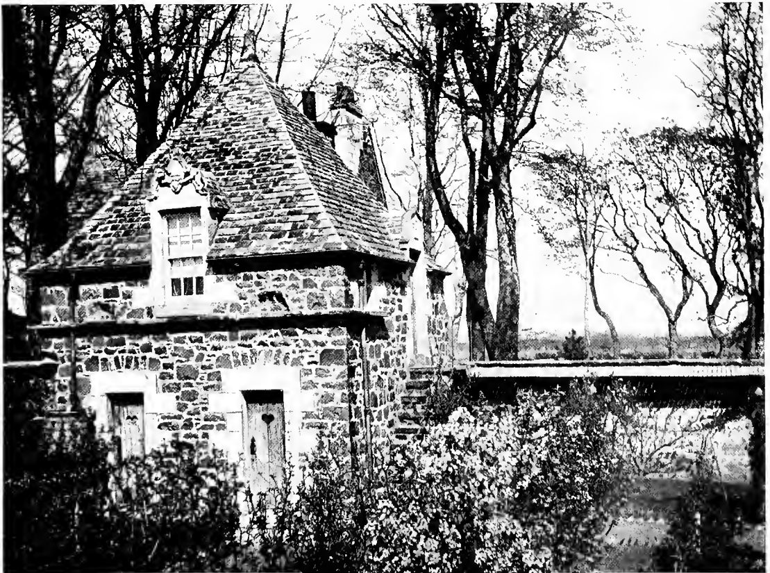
VIEW OF THE GARDEN PAVILION AT EARLSHALL, FIFE. BUILT OF LOCAL RUBBLE-WORK AND ROOFED WITH ARBROATH PAVEMENT SLATES B17
