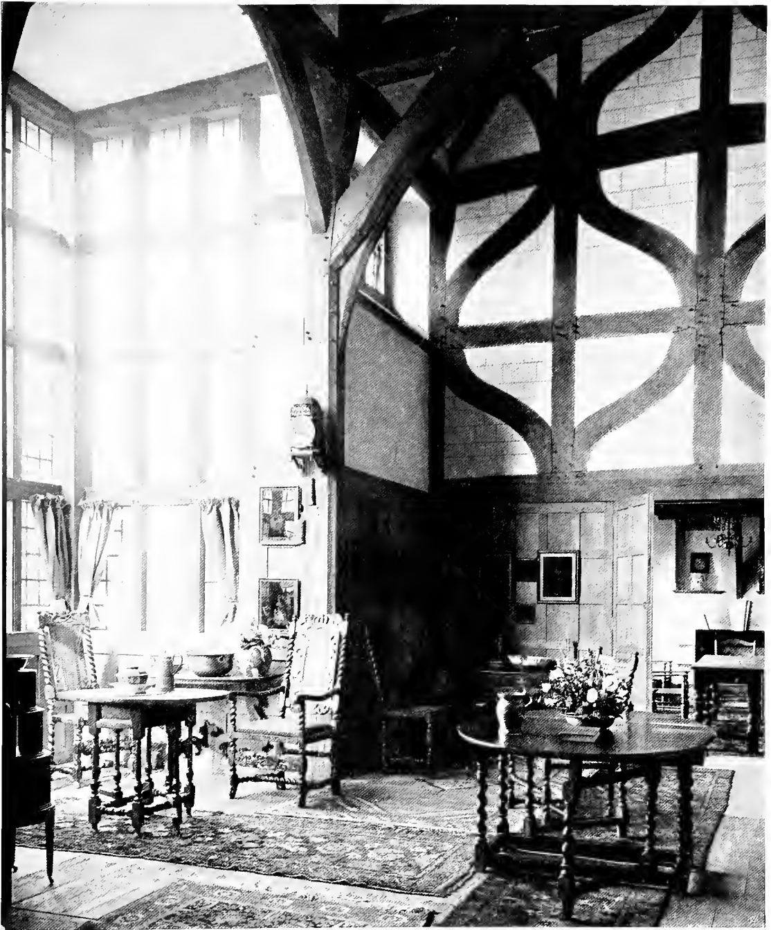
THE HALL IN A HOUSE AT SONNING-ON-THAMES, WITH THE PANELLING AND THE FLOOR OF OAK, AND THE OAK FRAMING FILLED IN WITH CHALK. AFTER A COPYRIGHT PHOTOGRAPH KINDLY LENT BY "COUNTRY LIFE"
