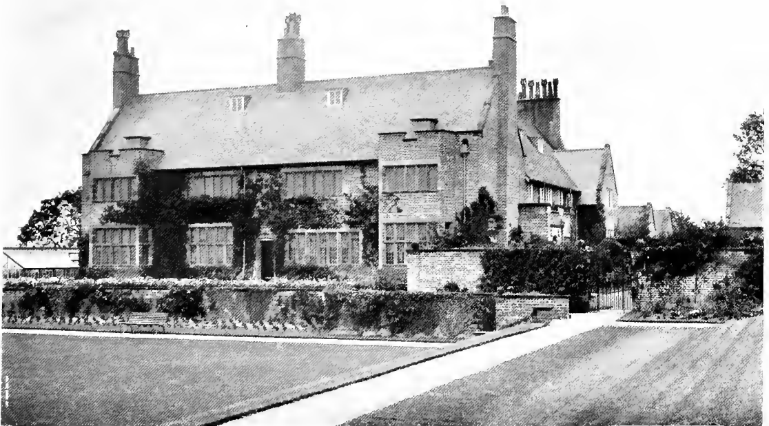
GARDEN FRONT OF A HOUSE AT BROMPTON, NORTHALLERTON, YORKSHIRE, BUILT IN 1895 FOR J. P. YEOMAN, ESQ. MATERIALS: THIN HAND-MADE RED BRICKS, LOCAL CREAMY STONE FOR THE DRESSINGS, RED TILES FOR THE ROOFS
