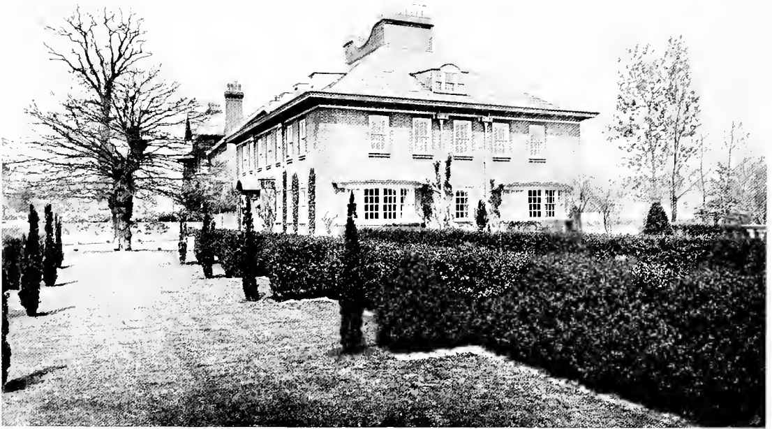
No. 2, WEST DRIVE, STREATHAM PARK
