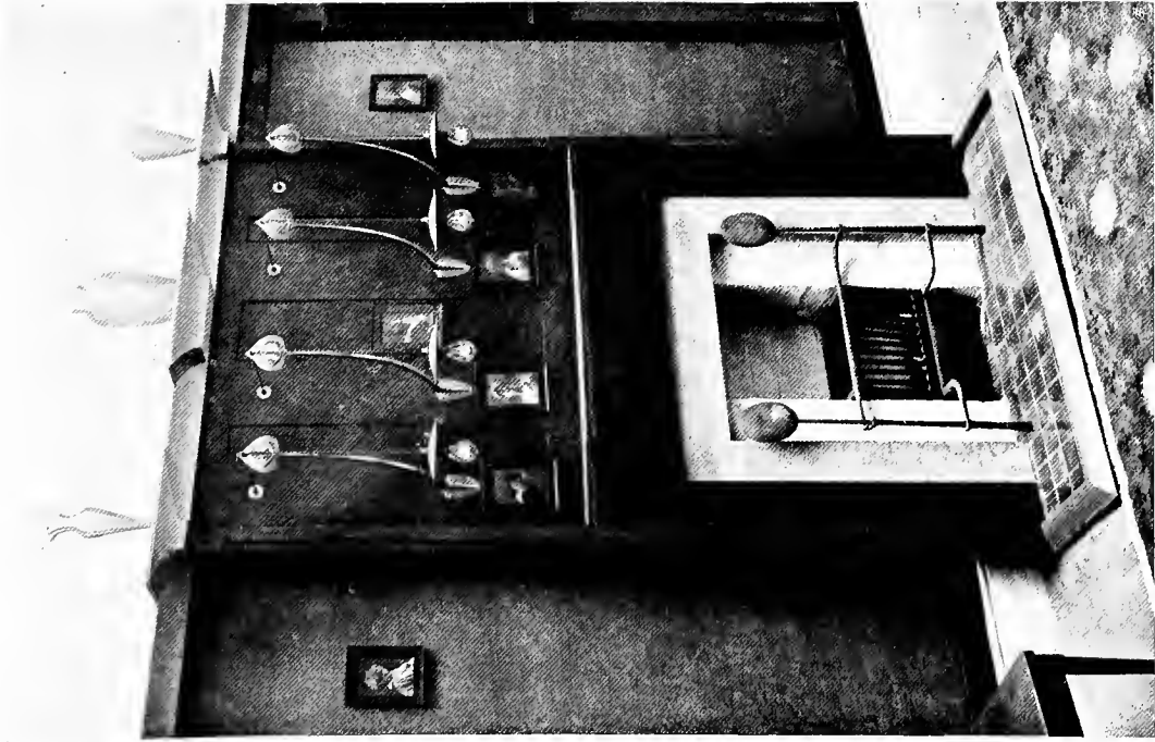
G-25 CHIMNEYPICE IN PINE WOOD, STAINED BLACK, WITH A SHELF OF OAK
