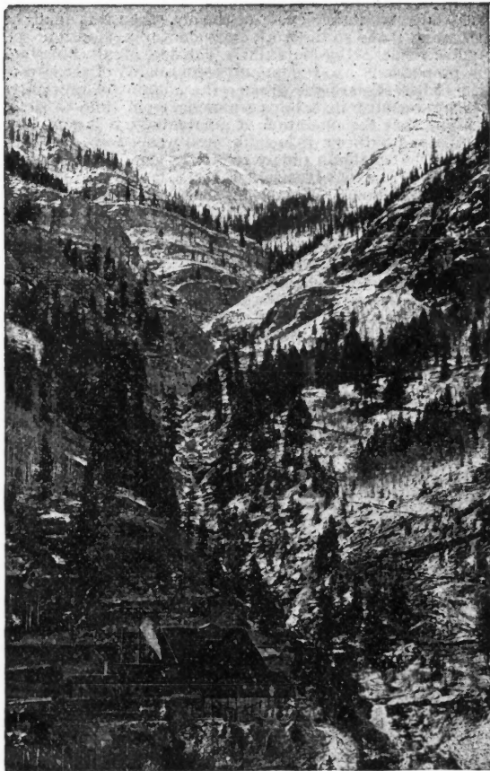
ELECTRIC POWER HOUSE FOR THE BELMONT MINE.
