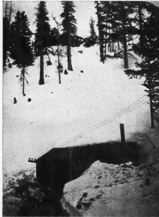
2. ENTRANCE TO TURKEY CREEK TUNNEL.
