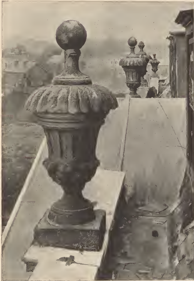
VASES ON PARAPET OF ROOF, ENTRANCE FRONT.
