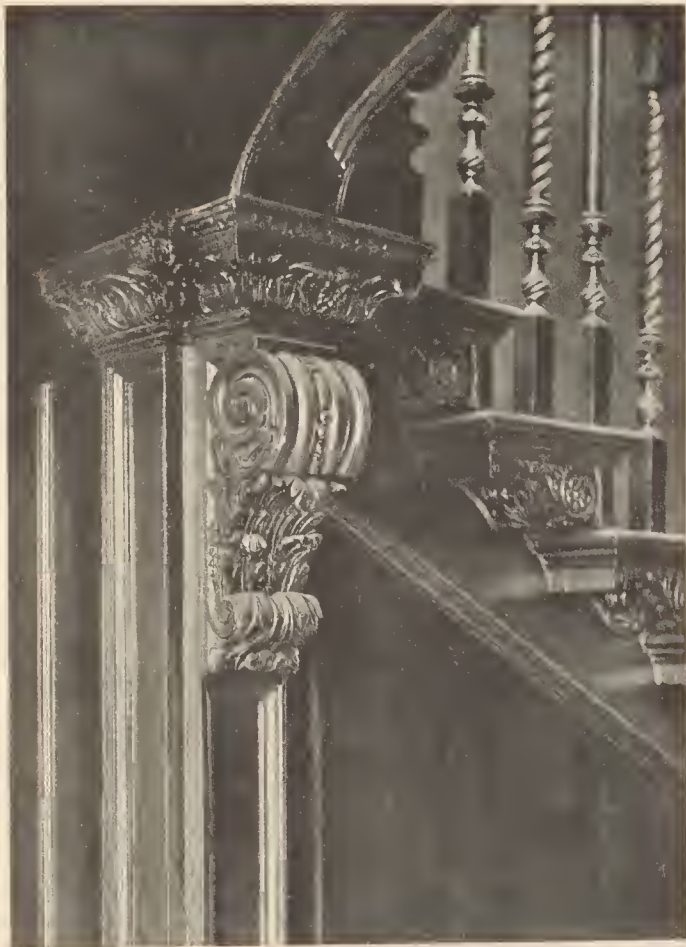
CARVED SPANDRILS AND CORBEL OF STAIRS IN HALL.
