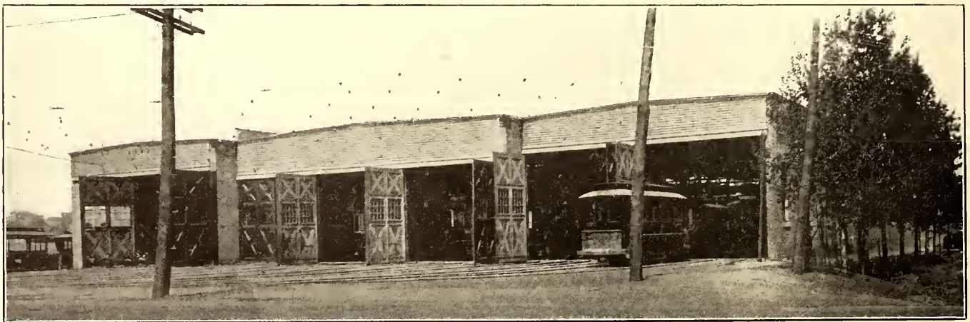
FIG. 26.—CAR HOUSE AND SHOPS ON WABASH AVENUE
