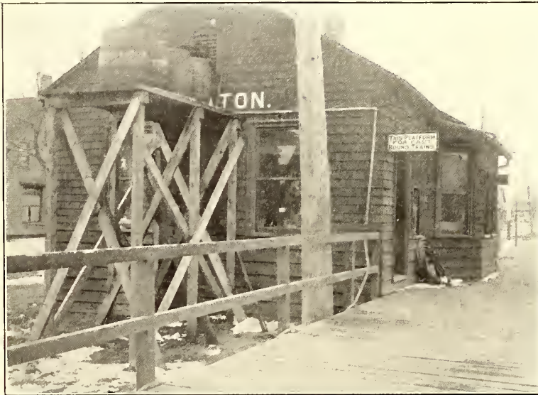
FIG. 3.—ELEVATED BARRELS AT WHEATON FOR FILLING TANKS IN CARS
