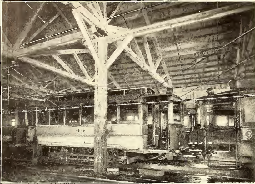
CAR IN TEST NO. 3—BEFORE THE FIRE
