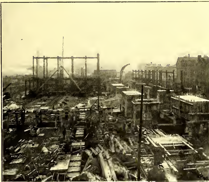
FIG. 6.—ENGINE AND BUILDING FOUNDATIONS, CHELSEA GENERATING STATION, LOOKING WEST
