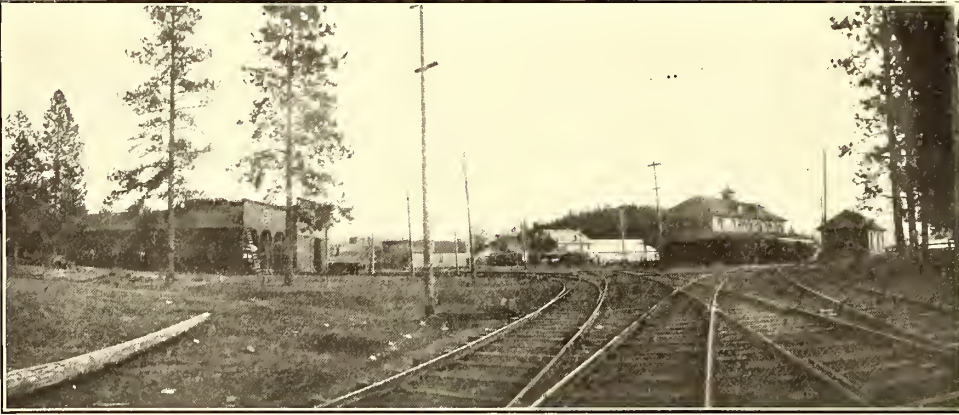
PASSENGER DEPOT, FREIGHT HOUSE, CAR HOUSES AND MACHINE SHOPS AT THE TERMINAL YARD OF THE COEUR D'ALENE & SPOKANE RAILWAY
