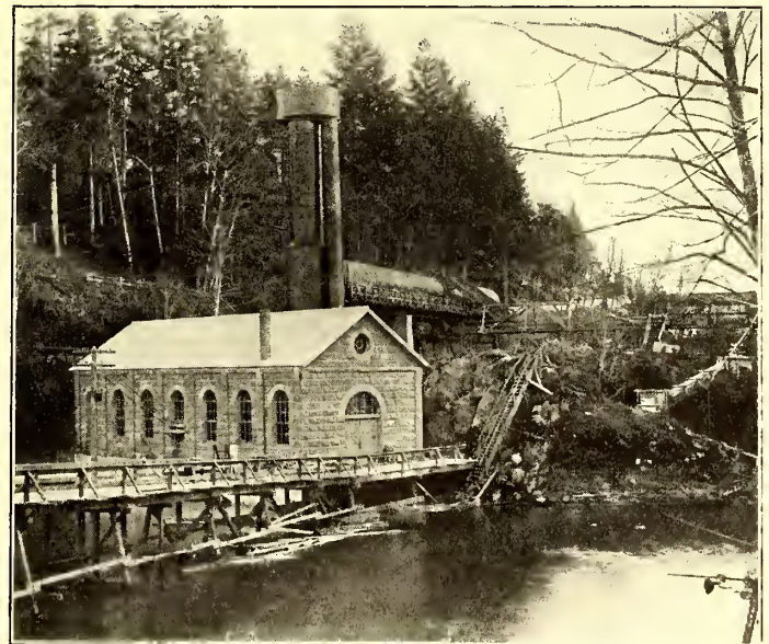
POWER HOUSE, STANDPIPE AND PIPE LINE
