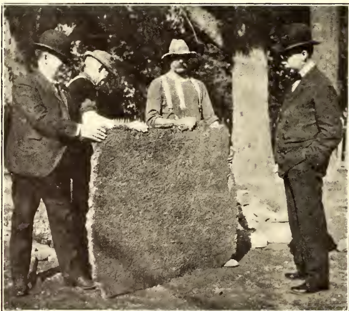
BOSTON ELEVATED RAILWAY, HIGH STREET, MEDFORD. SHOWING THE UPPER SURFACE OF A SECTION OF THE BITULITHIC PAVEMENT CUT FROM BETWEEN THE TRACKS TO INSTALL A CATCH-BASIN OUTLET
