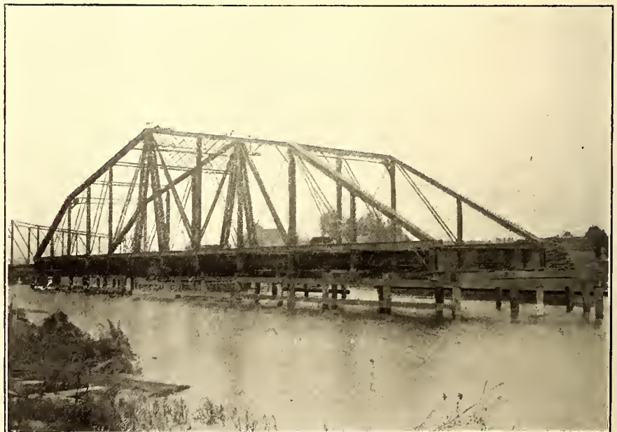
THE DOUBLE-TRACK DRAW-BRIDGE CROSSING THE RIVER ROUGE, NEAR DETROIT
