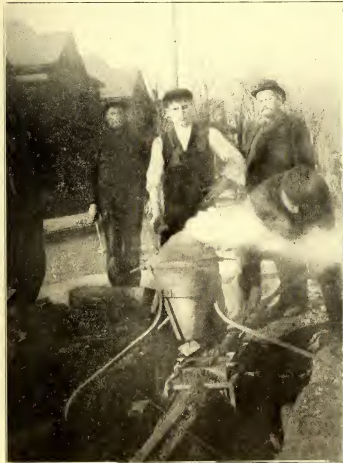
THE FIRST STEP IN THE REACTION, GETTING READY TO DRIVE PIN UP AND MAKE POUR
