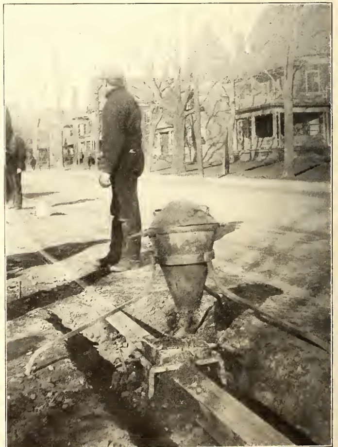
CRUCIBLE AND MOULD IN PLACE READY TO MAKE WELD
