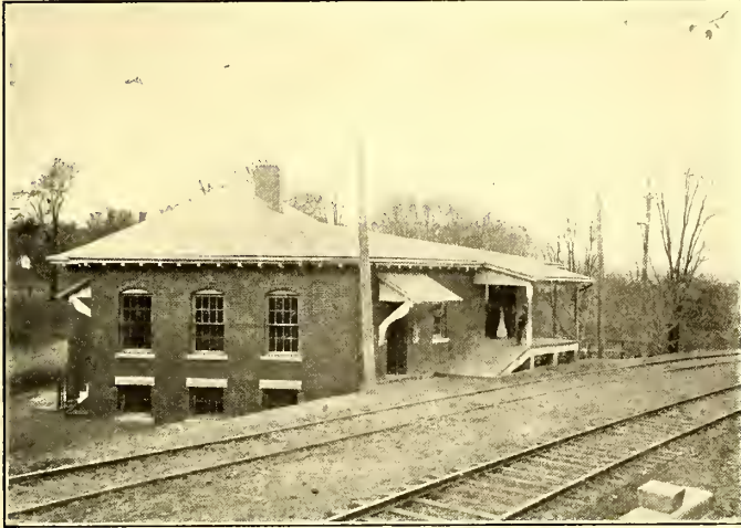
THE DAMASCUS SUB-STATION
