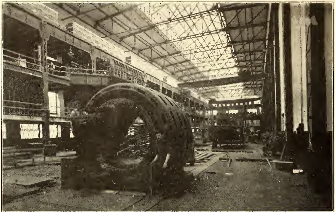
FIG. 28.—ALTERNATOR FIELD DURING ERECTION
