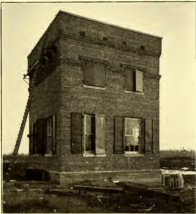
TRANSFORMER STATION AT REEDVILLE, IND.
