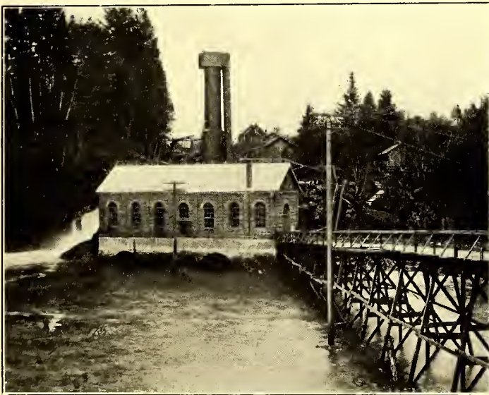
POWER HOUSE AND TUMWATER FALLS
