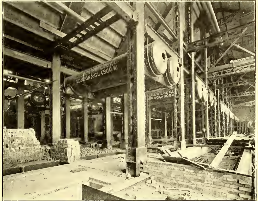
FIG. 14.—BOILERS AND ECONOMIZERS IN PROCESS OF ERECTION
