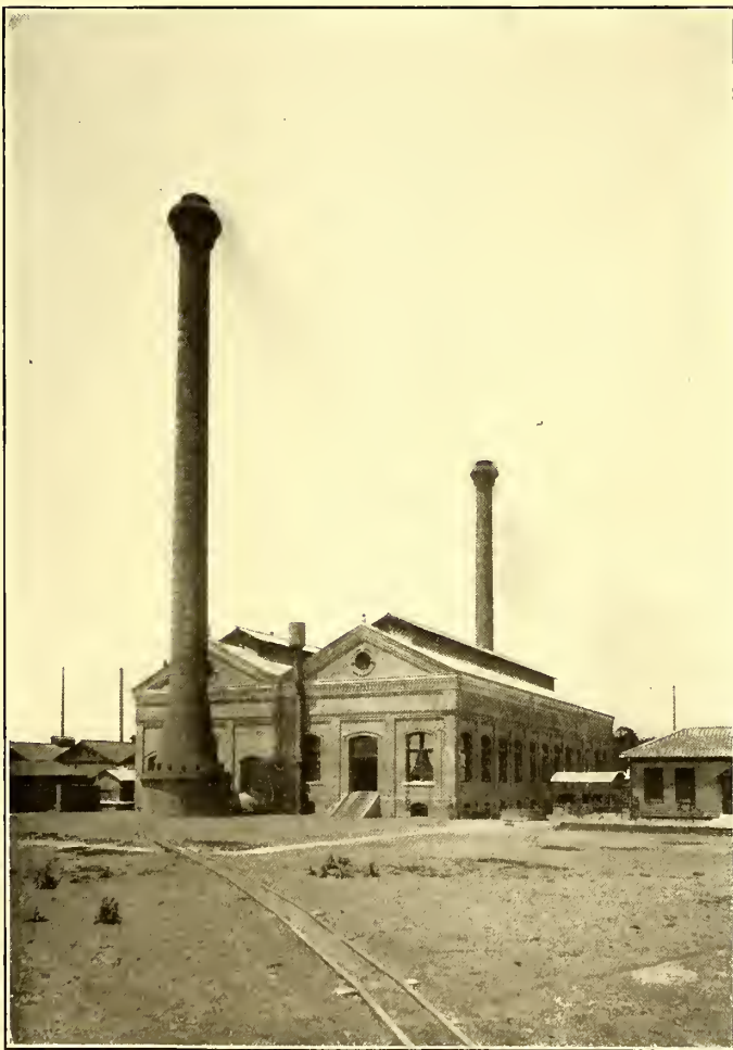
AN EXTERIOR VIEW OF THE POWER STATION
