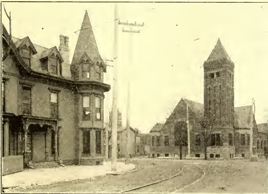
CURVE AT CORNER OF THIRD STREET AND MORGAN STREET, RUSHVILLE, IND.
