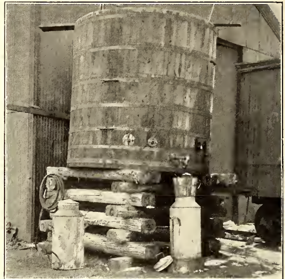
FIG. 4.—MIXING TANK FOR CALCIUM CHLORIDE AT THE CAR HOUSE
