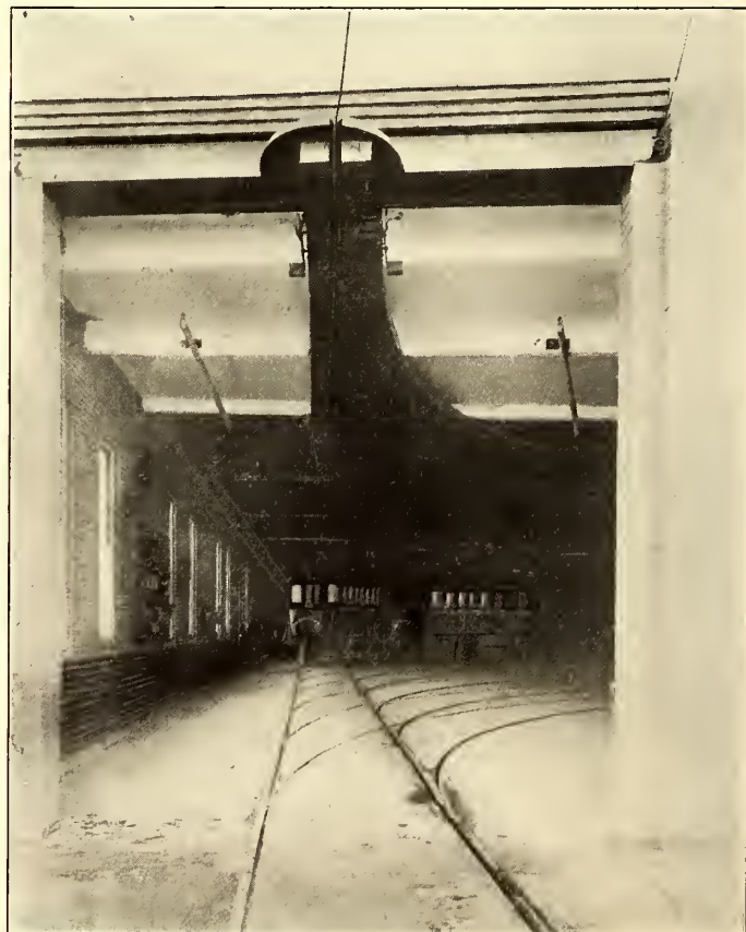
ENTRANCE DOOR, WETHERSFIELD CAR HOUSE, SHOWING LADDER TRACKS INSIDE THE HOUSE
