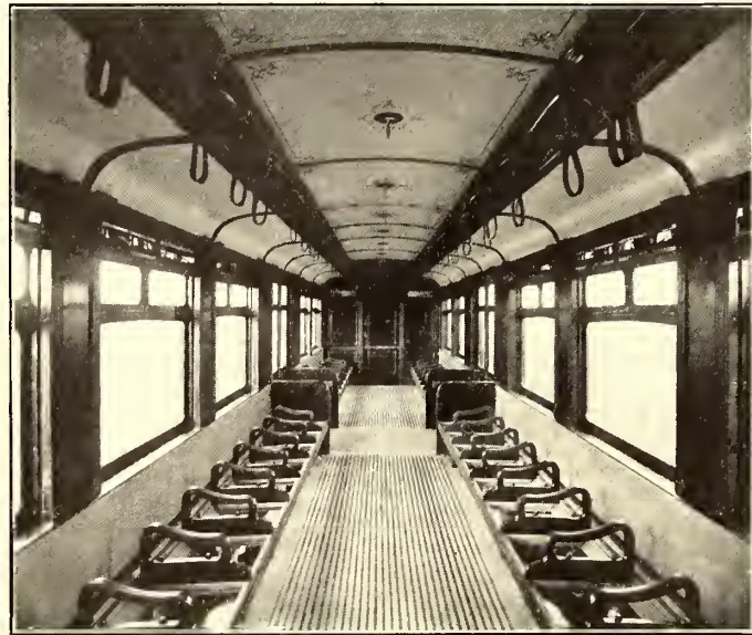
FIG. 71.—INTERIOR OF MOTOR CAR WITHOUT BAGGAGE COMPARTMENT FOR DISTRICT RAILWAY
