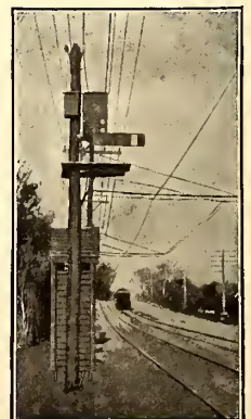
Boston & Worcester St. Ry. using Blake Signals
