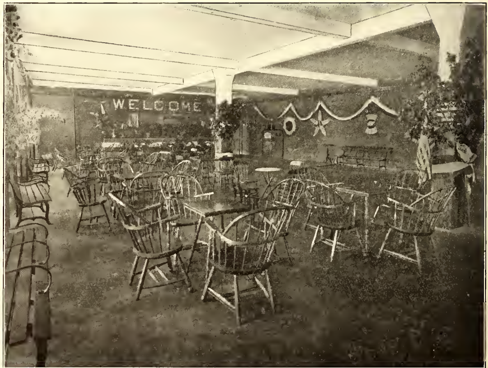
EMPLOYEES' ENTERTAINMENT ROOM, SHOWING PAINTED SPACE AROUND HYDRANT TO THE RIGHT OF THE CENTER POST
