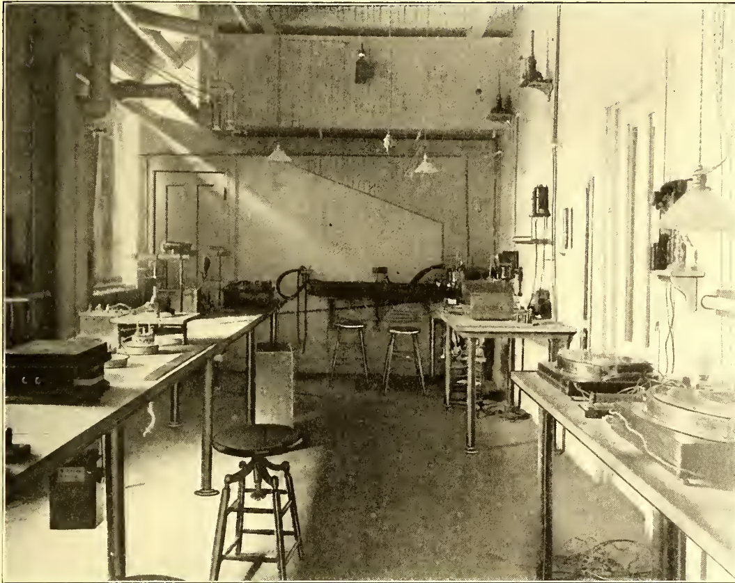
THE STANDARDIZING LABORATORY WHERE HIGH PRECISION TESTS OF RESISTANCE, CONDUCTIVITY, ETC., ARE CARRIED OUT
