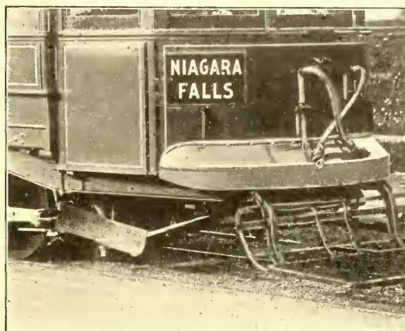
BUFFER ARRANGED WITH INCLINED TOP
