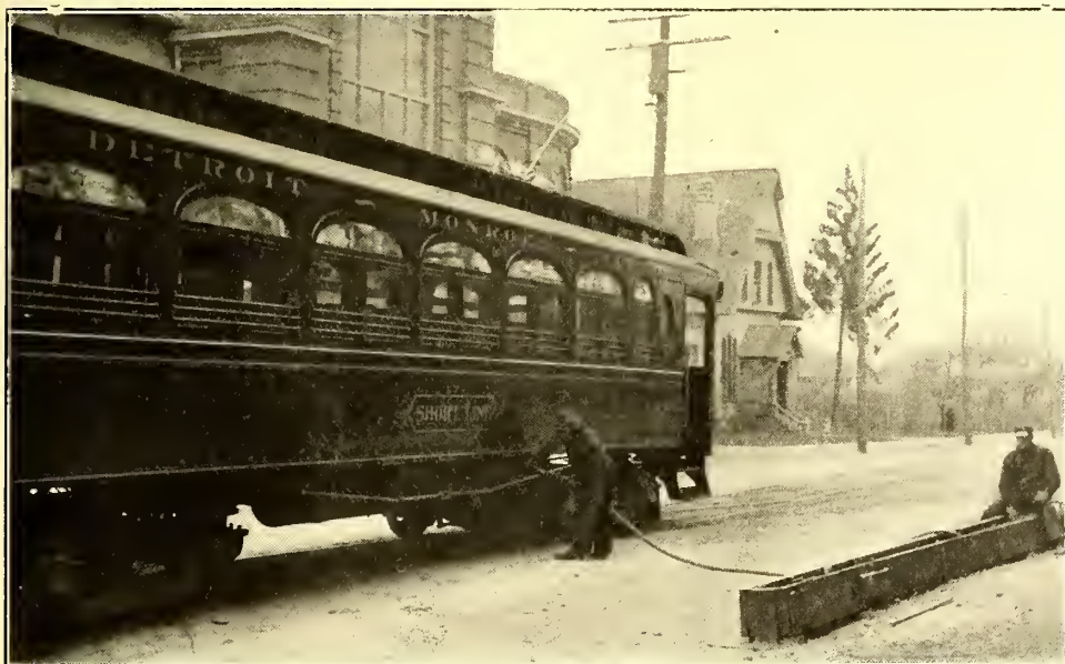
VIEW OF CAR AT THE STORAGE-AIR SYSTEM STATION AT THE MAIN POWER STATION IN MONROE, SHOWING METHOD OF CHARGING THE CAR RESERVOIRS WITH THE HIGH-PRESSURE AIR
