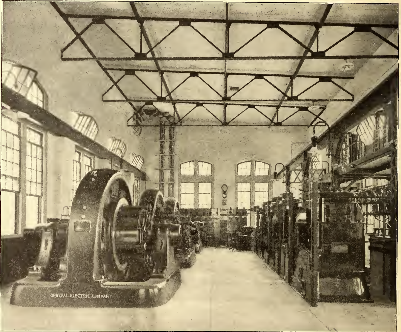
BROCKTON SUBSTATION—OLD COLONY STREET RAILWAY CO. THREE 750 Kw. ROTARY CONVERTERS.
