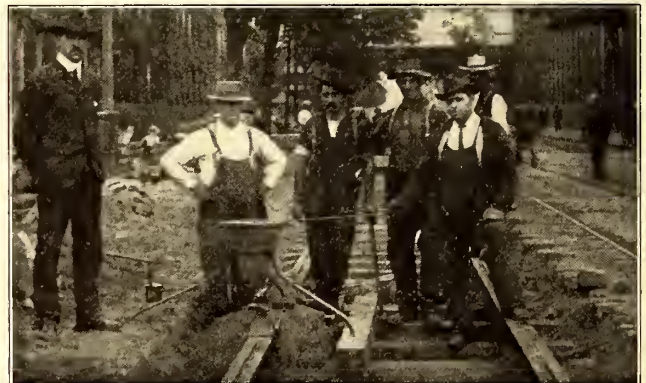
THERMIT RAIL WELDING, HOLYOKE, MASS.
