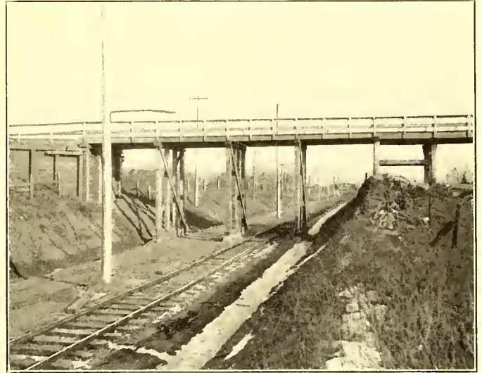
OVERHEAD CROSSING NEAR JULIETTA, IND.
