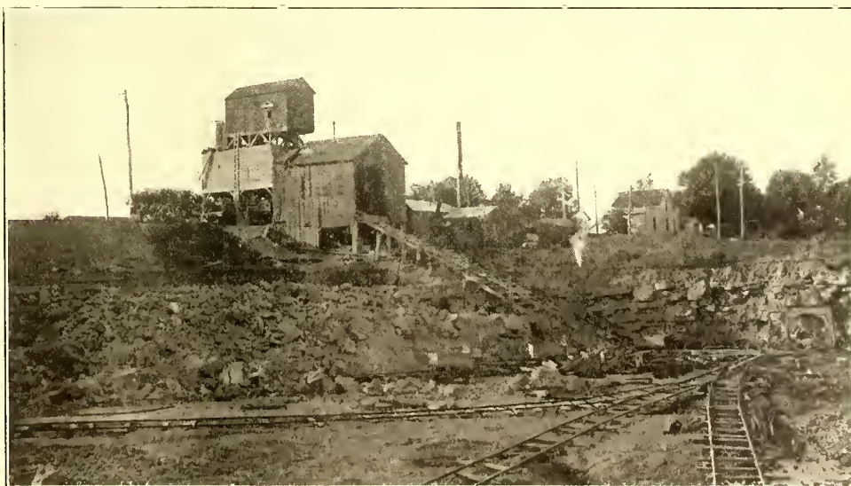
THE QUARRY AND STONE-CRUSHER PLANT AT NEWPORT, OPERATED BY THE RAILROAD COMPANY, FROM WHICH 60,000 CU. YDS. OF STONE BALLAST HAS BEEN REMOVED FOR TRACK BALLASTING
