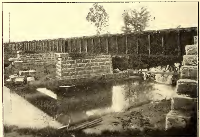
BRIDGE OVER BLUE RIVER, NEAR MORRISTOWN, IND.
