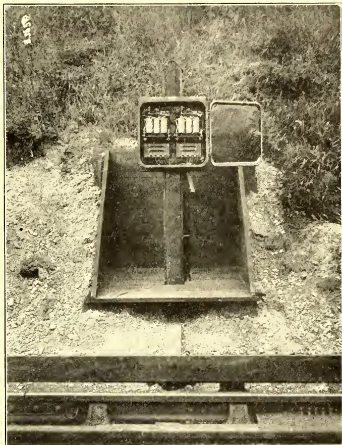
FIG. 66.—MOUNTING OF SIGNAL RELAYS
