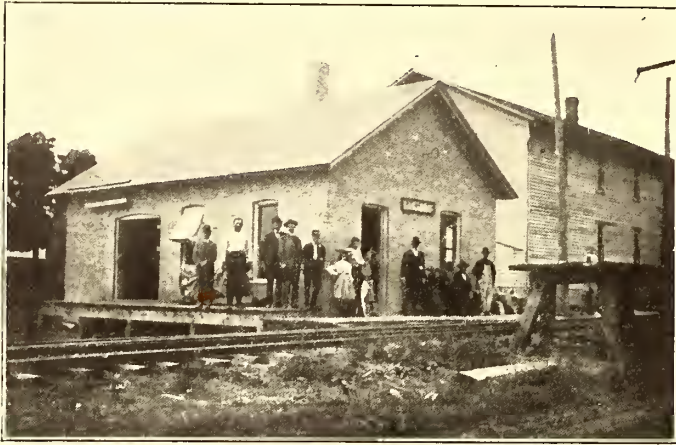
THE SUB-STATION AND DEPOT AT DEWITT, UPON THE INTERURBAN LINE
