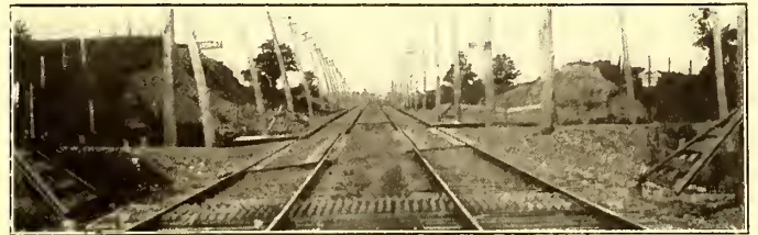
PROTECTING HIGHWAY CROSSINGS, UTICA & MOHAWK
