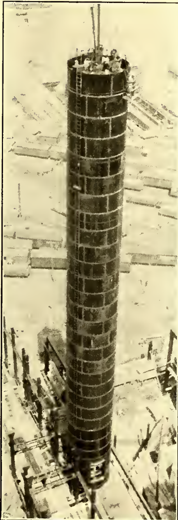
VIEW OF STACK DURING ERECTION
