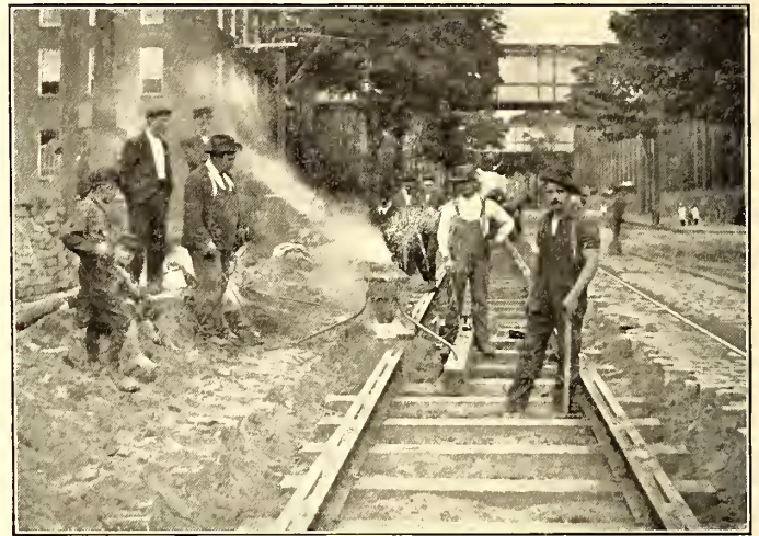
THERMIT REACTION IN PROGRESS
