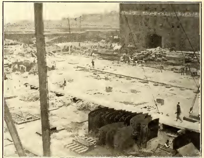
LAYING THE CONCRETE FOR THE STATION FOUNDATION
