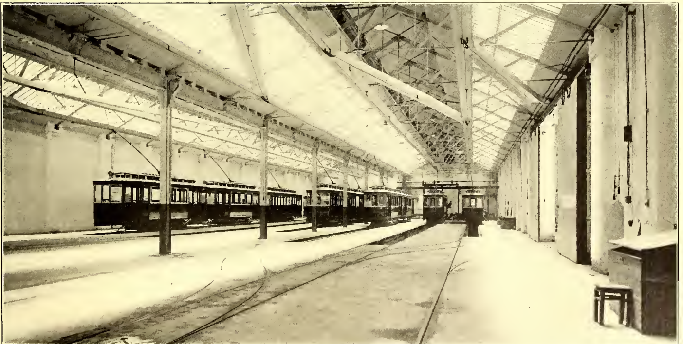
SIX-TRACK CAR SHED OF THE HONG KONG TRAMWAYS, 220 FT. LONG, AND ACCOMMODATING THIRTY-FIVE 29-FT. CARS
