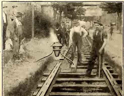
(THERMIT RAIL WELDING, HOLYOKE, MASS.)
