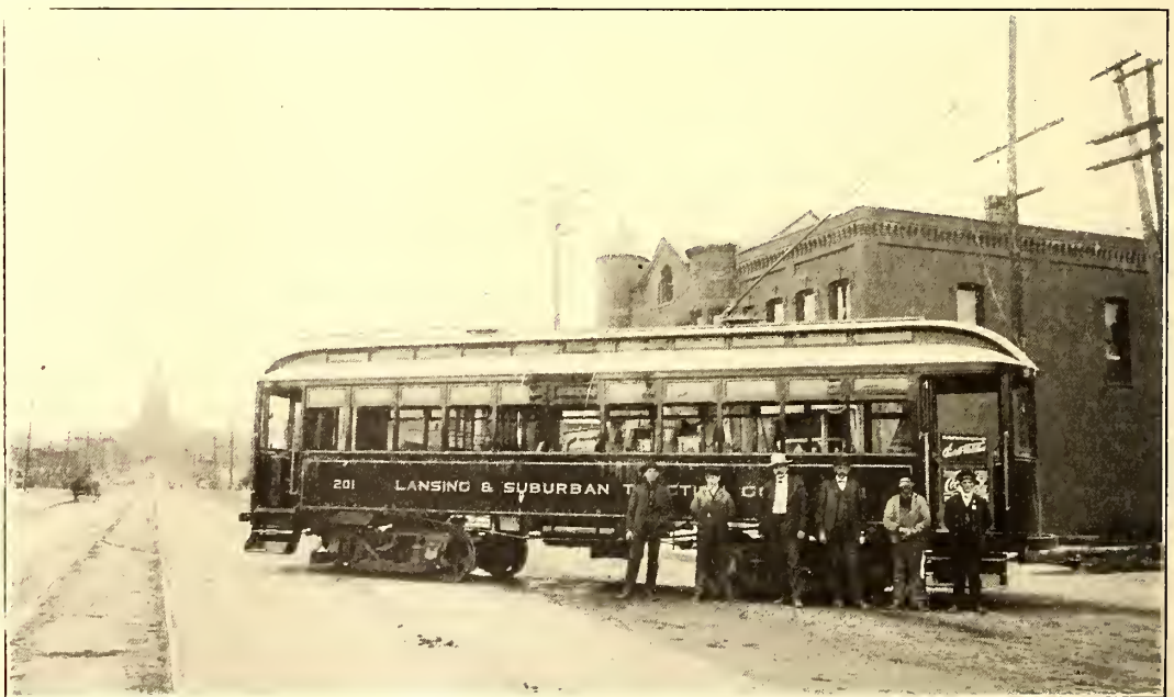
ONE OF THE STANDARD DOUBLE-TRUCK CARS IN USE UPON THE INTERURBAN DIVISION, TURNING INTO THE CITY TRACKS TO ENTER LANSING
