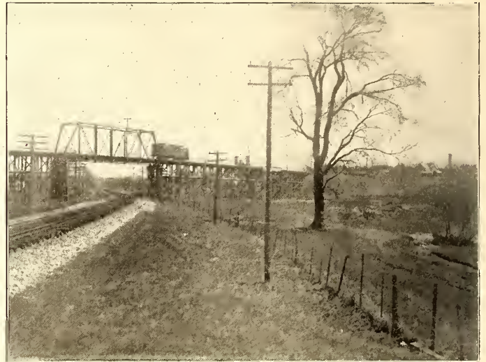
CROSSING ABOVE THE PENNSYLVANIA RAILROAD AT LOUISVILLE
