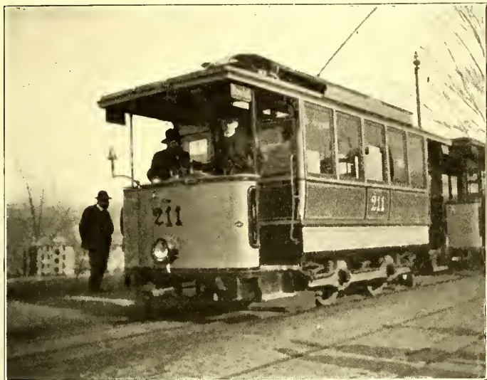
FIG. 3.—STUTTGART MOTOR CAR AND TRAILER EQUIPPED WITH HYDRO-ELECTRIC BRAKE
