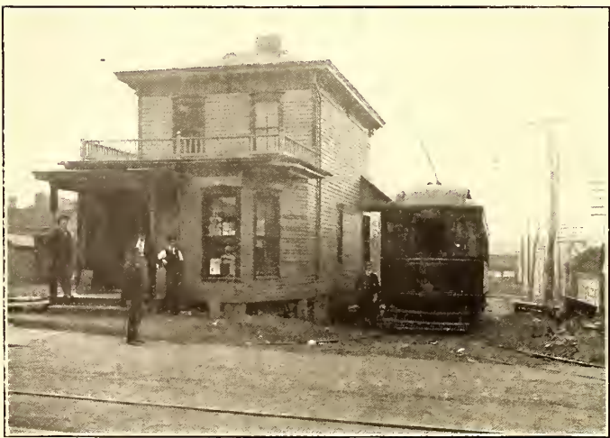
THE SALEM TERMINAL OF THE STARK ELECTRIC RAILWAY
