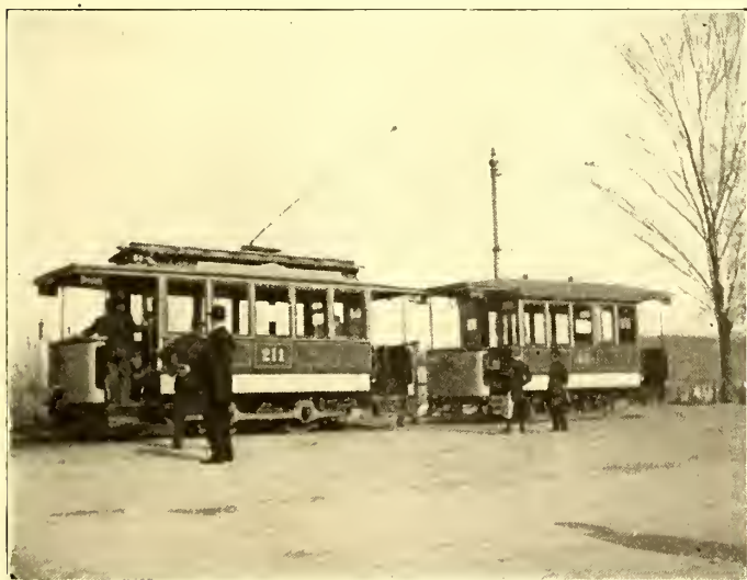
FIG. 4.—ANOTHER VIEW OF THE STUTTGART EQUIPMENT
