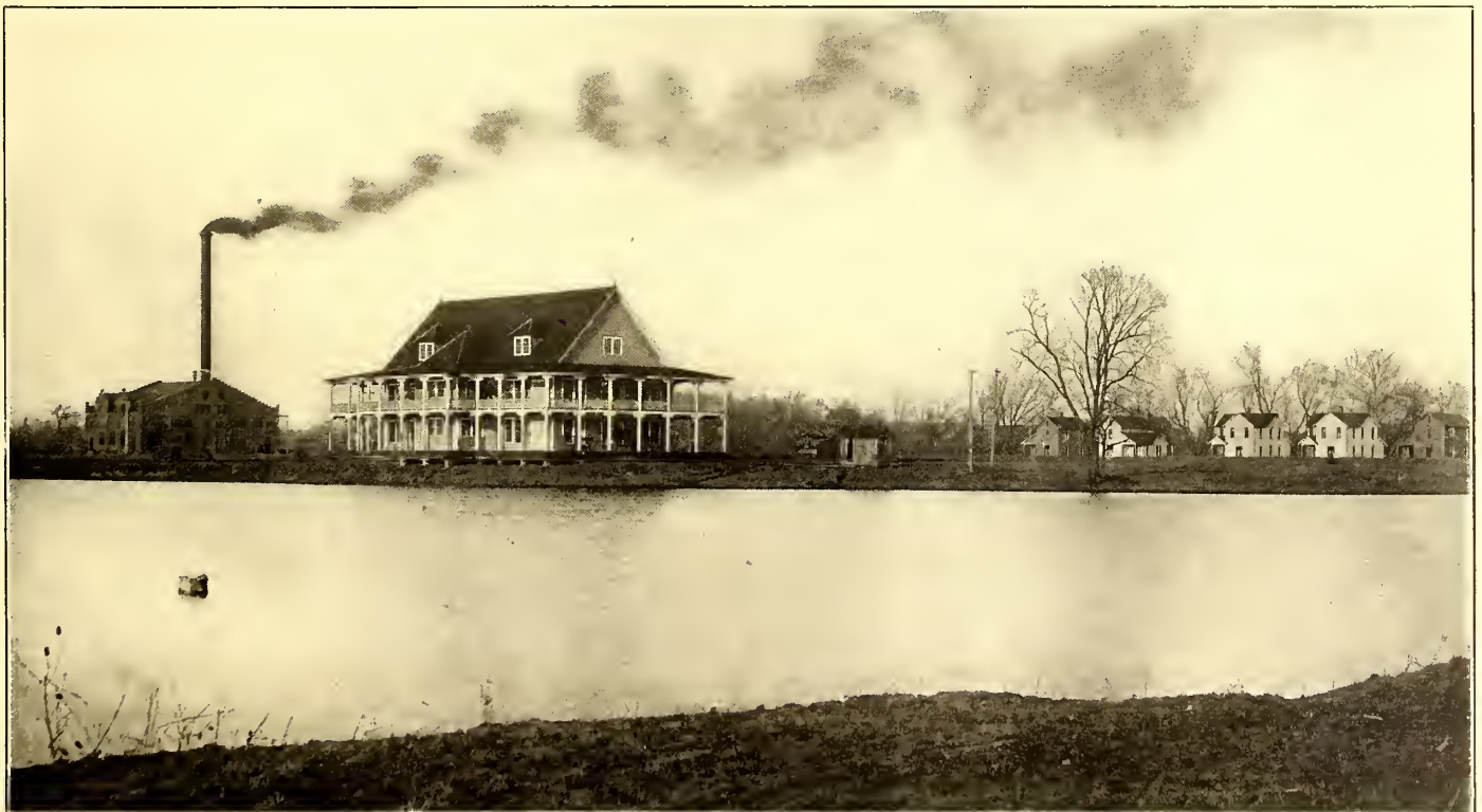
PART OF PANORAMIC VIEW OF LAKE, SHOWING THE POWER HOUSE AND PAVILION
