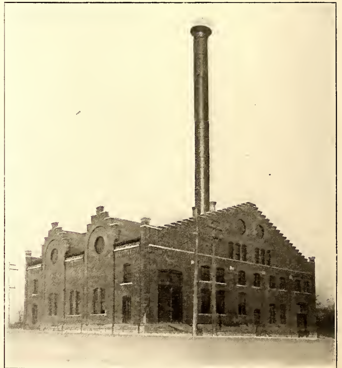
EXTERIOR OF POWER HOUSE
