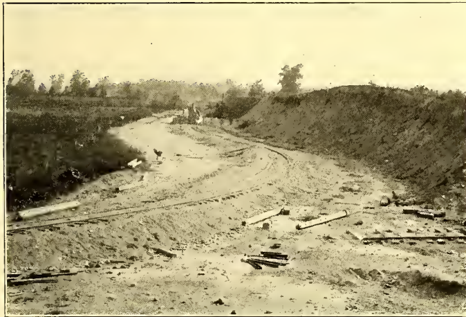
STEAM SHOVEL WORKING IN GRAVEL PIT
