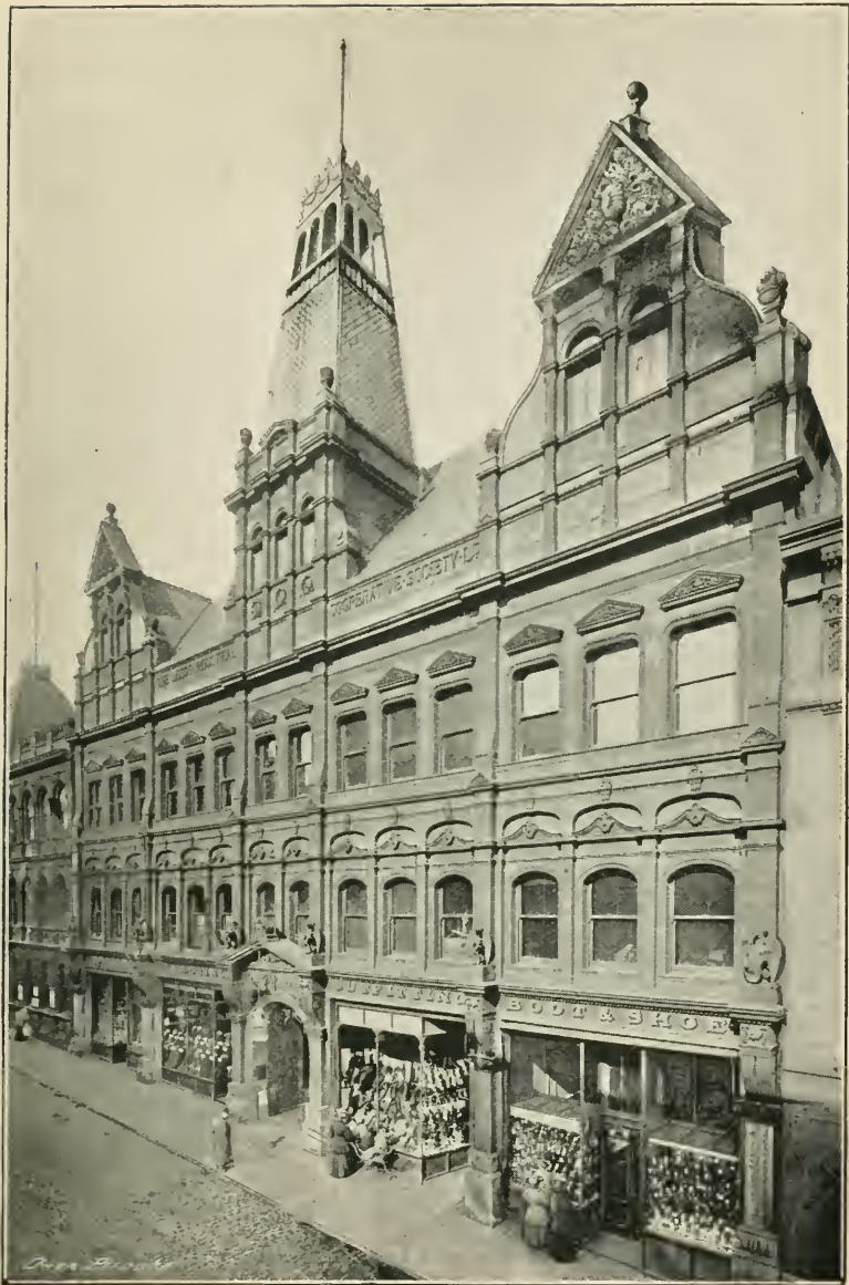
CENTRAL PREMISES, ALBION STREET (EAST SIDE).
