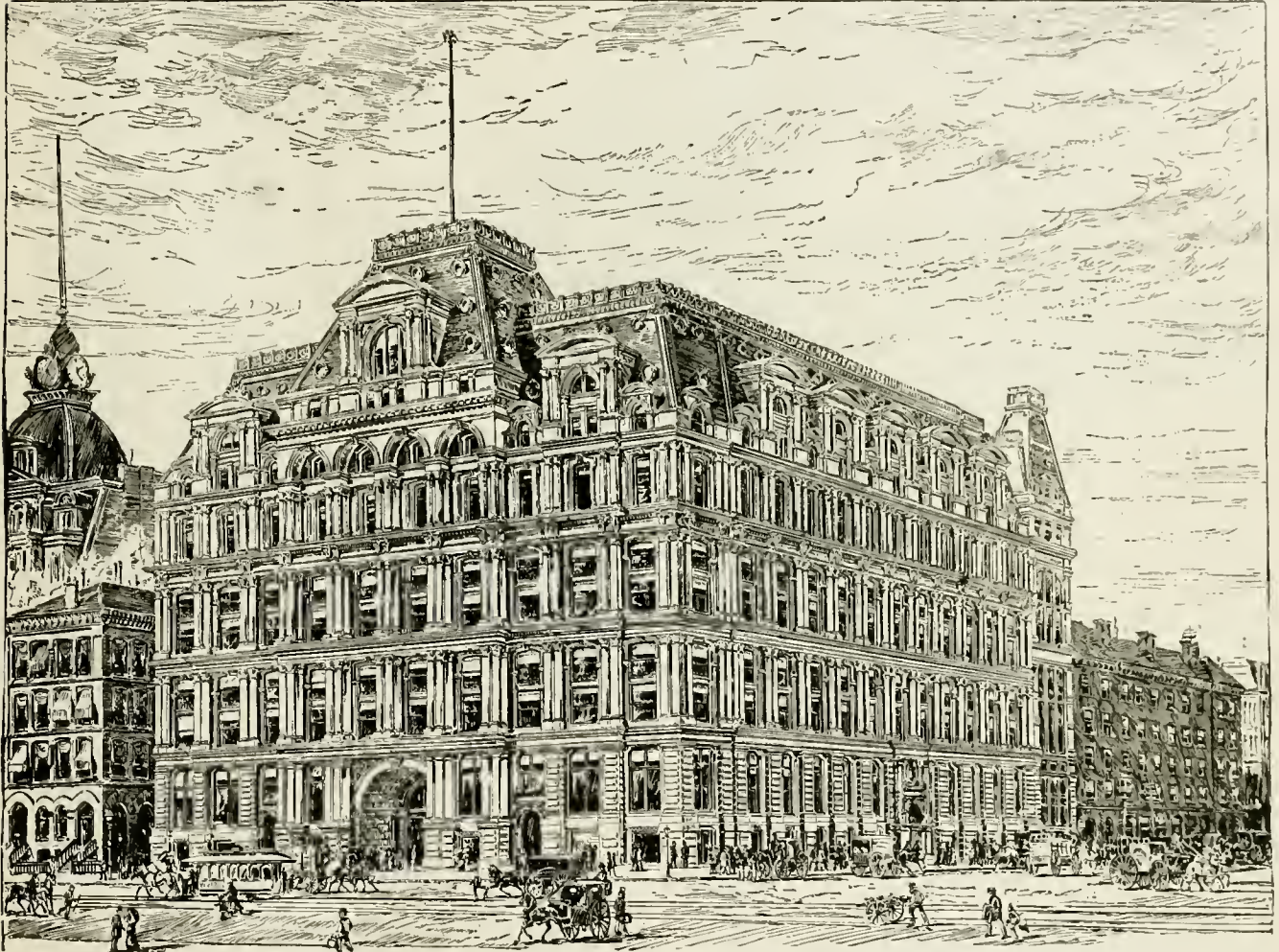
EQUITABLE LIFE ASSURANCE BUILDING, NEW YORK.
