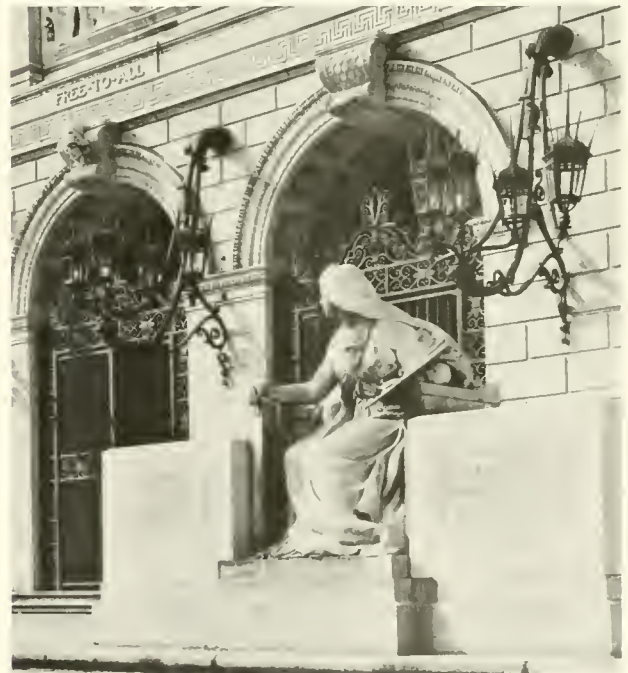
The facade of the McKim building showing sculptor Bela L. Pratt's heroic figure, Art.
