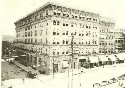
WASHINGTON TRUST BUILDING
