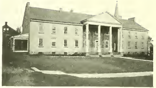
OLD WASHINGTON ACADEMY BUILDING, 1793
