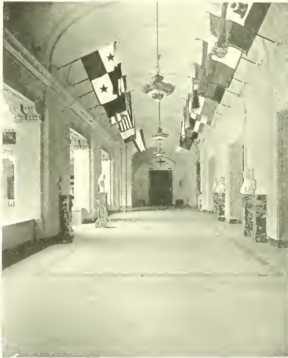
CORRIDOR, PAN-AMERICAN UNION BUILDING
