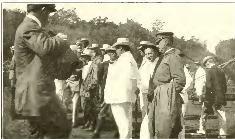
AT THE PACIFIC DIVISION OF THE PANAMA CANAL President Taft talking to Division Engineer Williamson.
