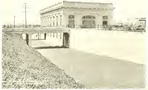
VIEW OF STATION FROM SOUTHEAST, SHOWING ELEVATED BAGGAGE AND EXPRESS DELIVERY AND CONCRETE PLATFORMS
