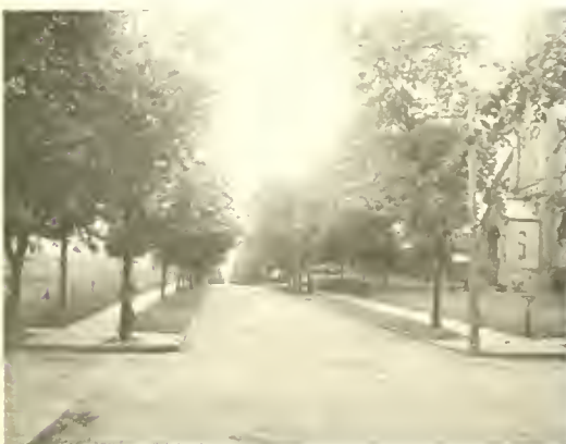
EAST WHEELING STREET
