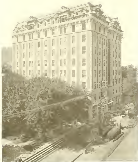
NEW GOFF BUILDING, CLARKSBURG
