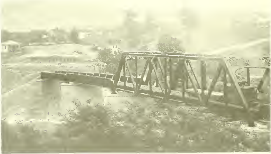
NEW BRIDGE ACROSS MONONGAHELA RIVER, NEAR CLARKSBURG, W. VA.
