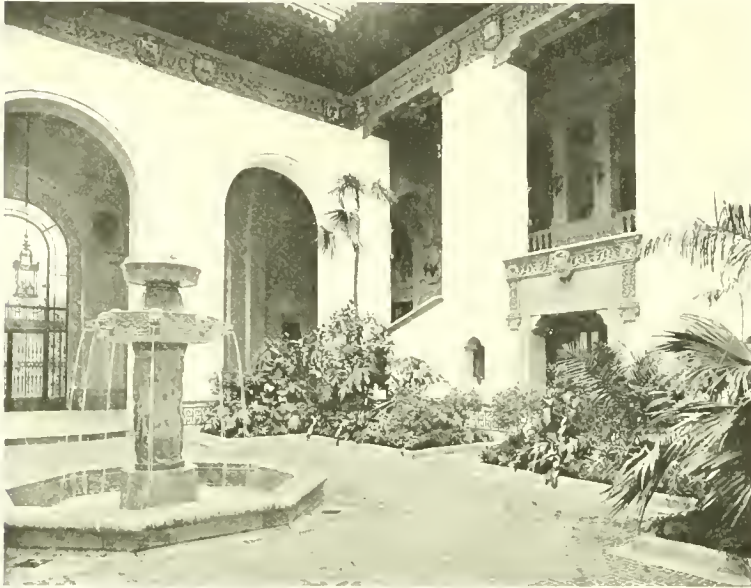
THE PATIO, PAN-AMERICAN UNION BUILDING, WASHINGTON, D. C.
