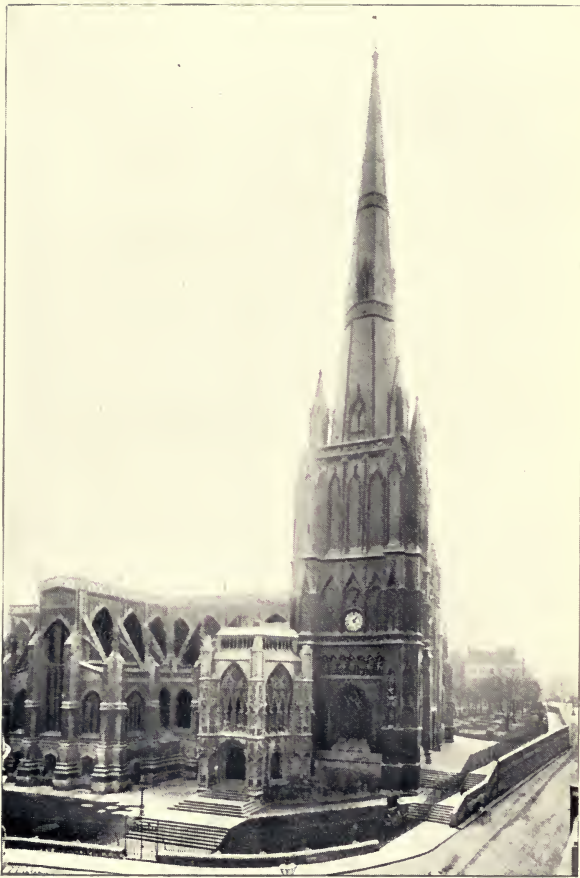
ST. MARY REDCLIFF CHURCH, BRISTOL (NORTH VIEW)
