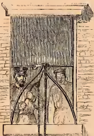
A "BREAK," THROUGH WHICH THE ROPES PASS, USED BY THE POMPER CORPS TO REGULATE THE RAPIDITY OF THE DESCENT FROM ABOVE.
