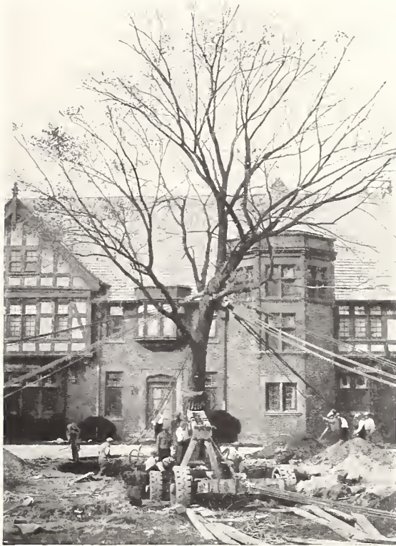
Large Elm being planted at home of Mr. Donald Geddes, Glen Cove, L. I.
