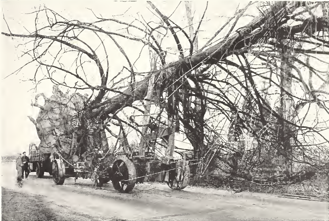
Large Linden being moved to estate of Mr. Marshall Field, Huntington, L. I. Two such trees were successfully transplanted. Note the Hicks' way of digging with large balls of earth and saving all extending roots by carefully wrapping, to prevent drying out.
