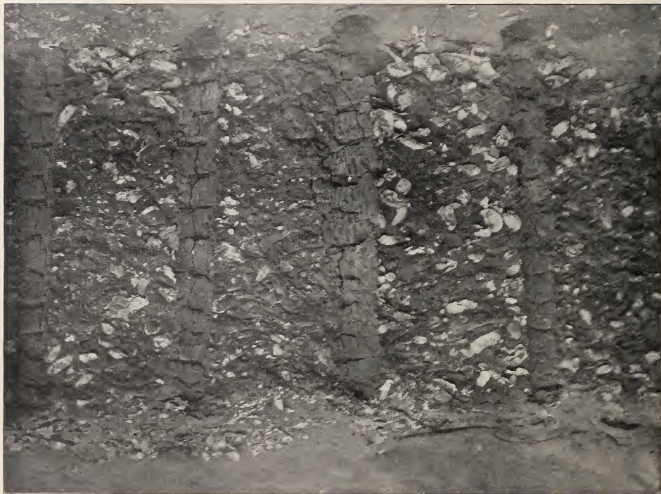
Fig. 4.—Portion of wall showing molds of uprights and cross-pieces. Aboriginal structure. Mound on Little island, S. C.
