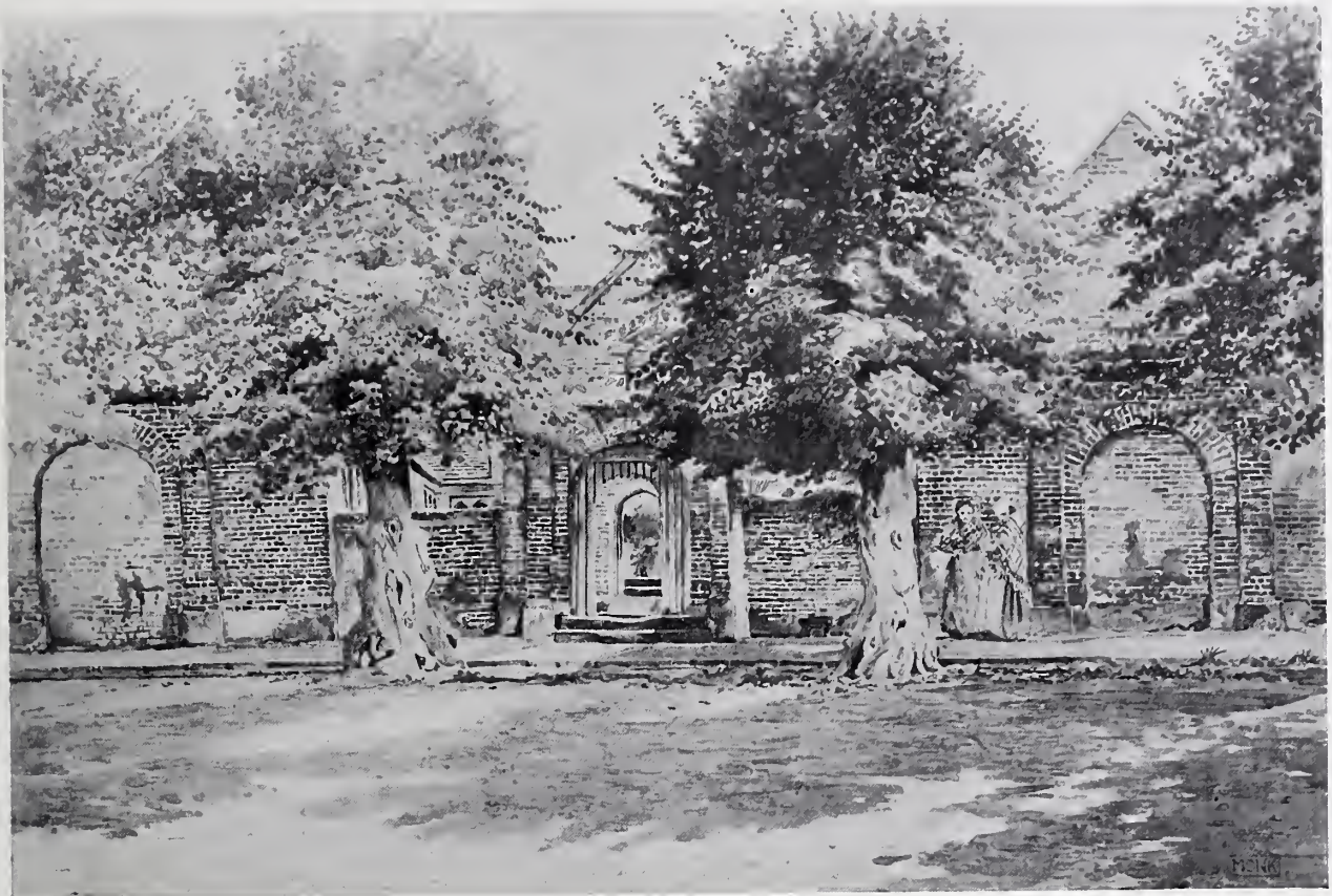
Entrance to Almshouses from the High Street.
