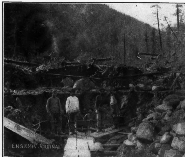
HAND WORK IN THE GRAVEL
