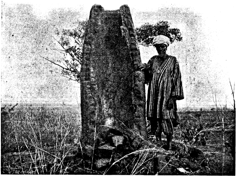
SECTION OF NATIVE IRON-SMELTING FURNACE, NEAR BANJELI, WEST-CENTRAL TOGO.
