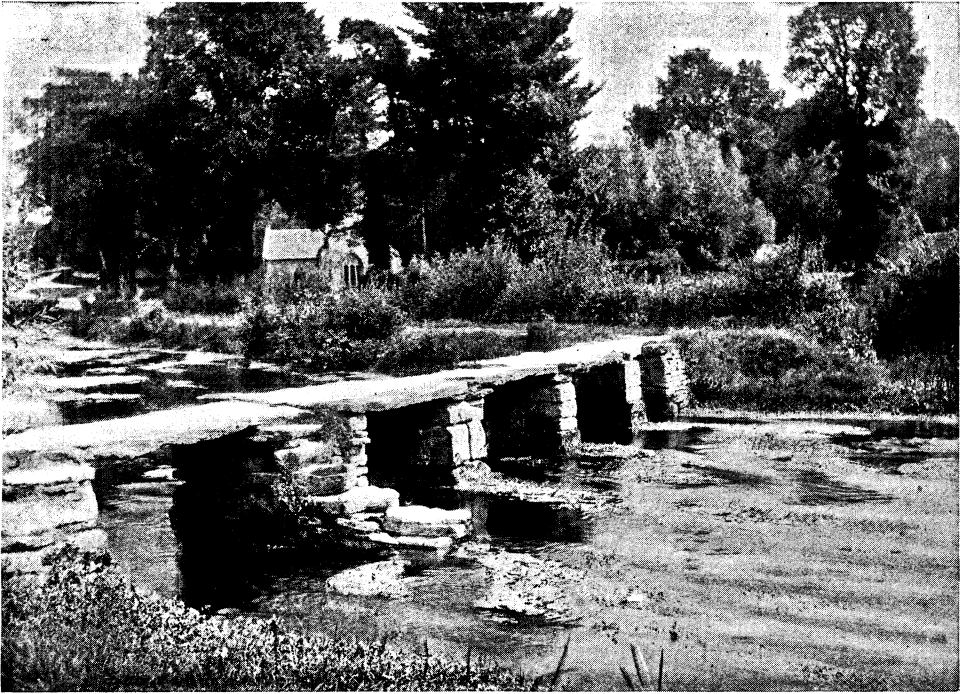
THE LEACH : THE BRIDGE AT EASTLEACH.
