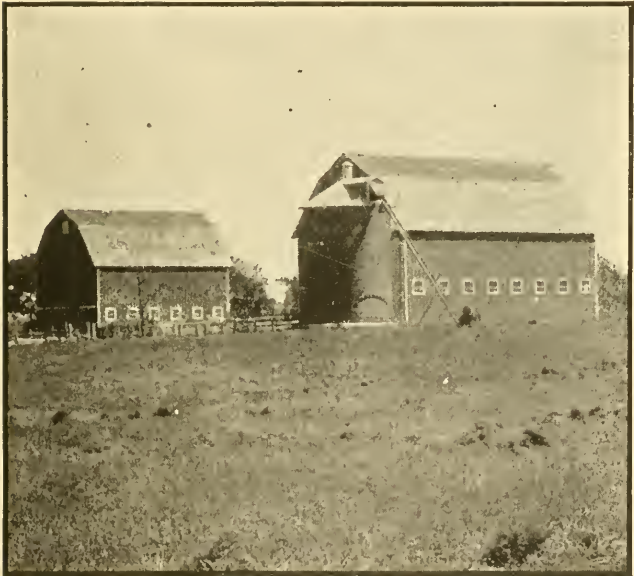
Fig 36—Silo Attached to Barn
