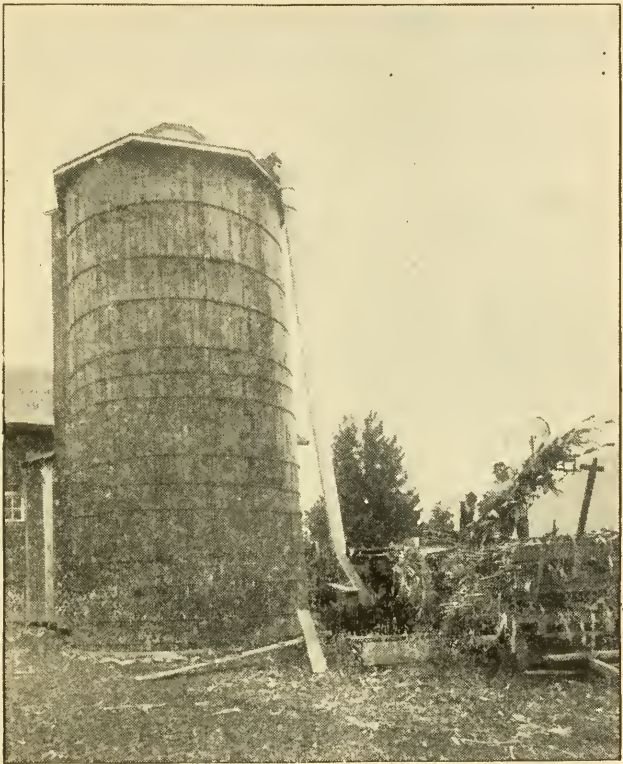
Fig 43—Filling Silo with Blower
