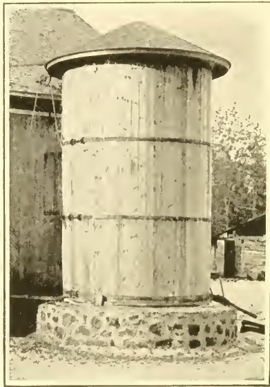
Fig 35—Cheap Stave Silo
