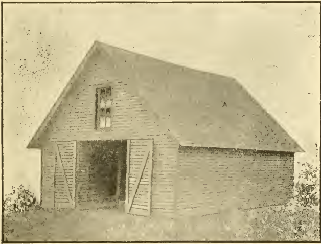
Fig 28—Modern Corn Crib At Minnesota experiment station
