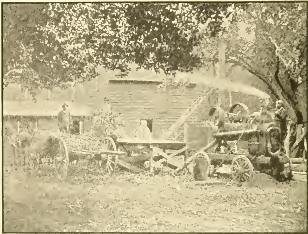
Fig 39—Filling the Silo
