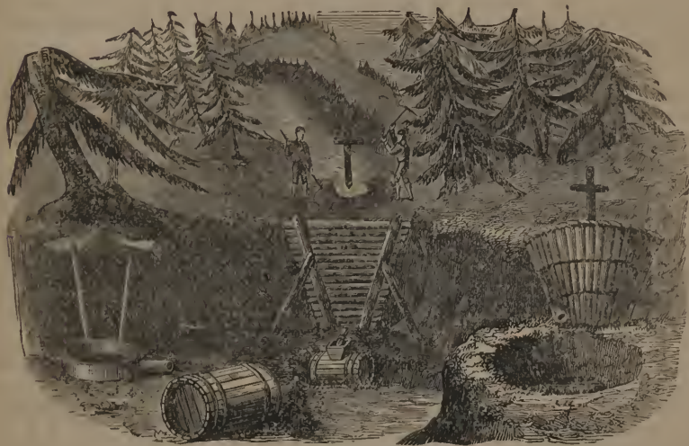
Preparation of Tar.
