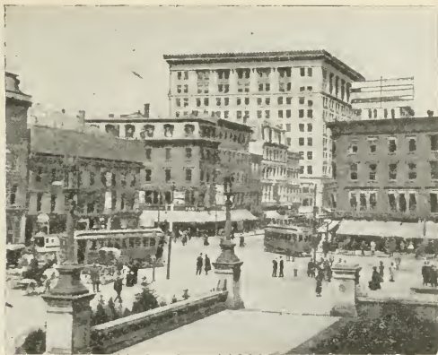
WORCESTER—CITY HALL SQUARE AND "BUSY CORNER"
