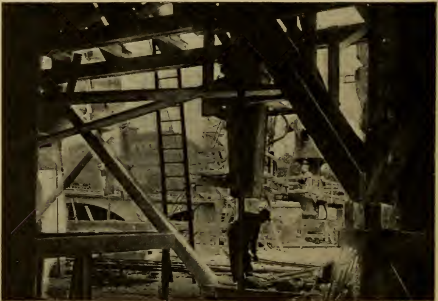
The Paris Métropolitain under Construction
