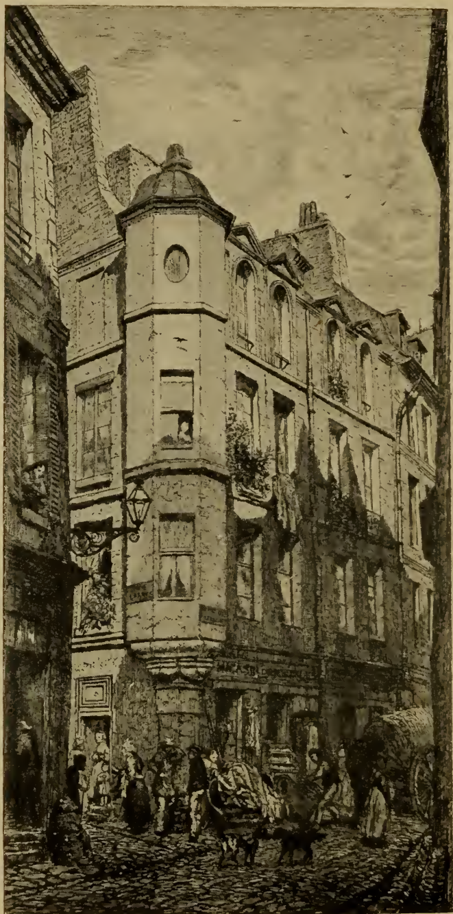
House with corner turret in the Rue des Cordeliers
