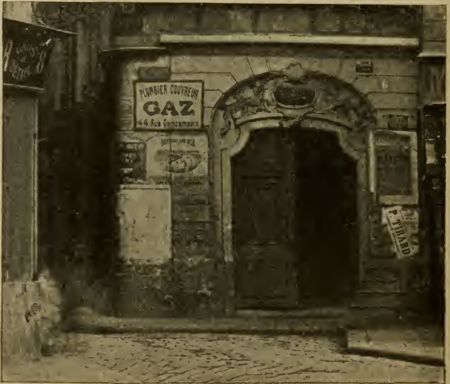
The old Bureau des Lingères , Rue Courtalon (now demolished), former Entrance Gateway
