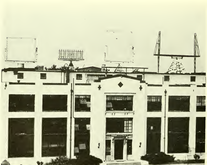
2. Penthouse roof, Bldg. 12, showing (right to left) pre-XAF, XAF, 400-Mc, and CXAM antennas. Pre-XAF is hand driven; all others are motor driven with remote control. Summer 1940.
