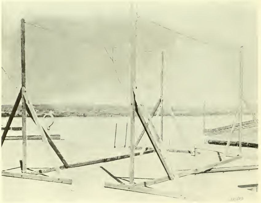
2. Original 28-Mc radar receiving antenna; \lambda/2 dipole with \lambda/2 reflector. April 1936.
