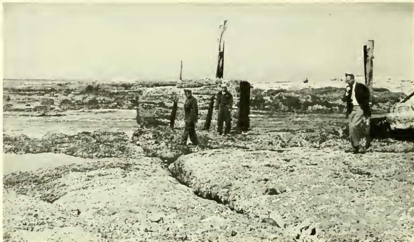
1. Dock at Isla Mocha destroyed by tsunami and former shoreline raised 2\frac{1}{2} meters. Before, top of concrete was awash at low tide. Picture taken at high tide.
