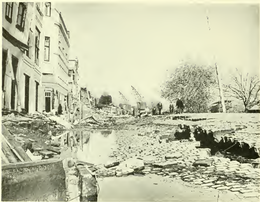
1. Ship-loading equipment and buildings along Valdivia waterfront severely damaged, caused by slumping.
