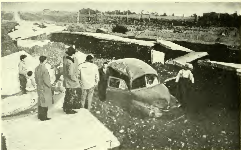
2. Road construction in swampy area near Puerto Varas. The undamaged road can be seen in upper left.
