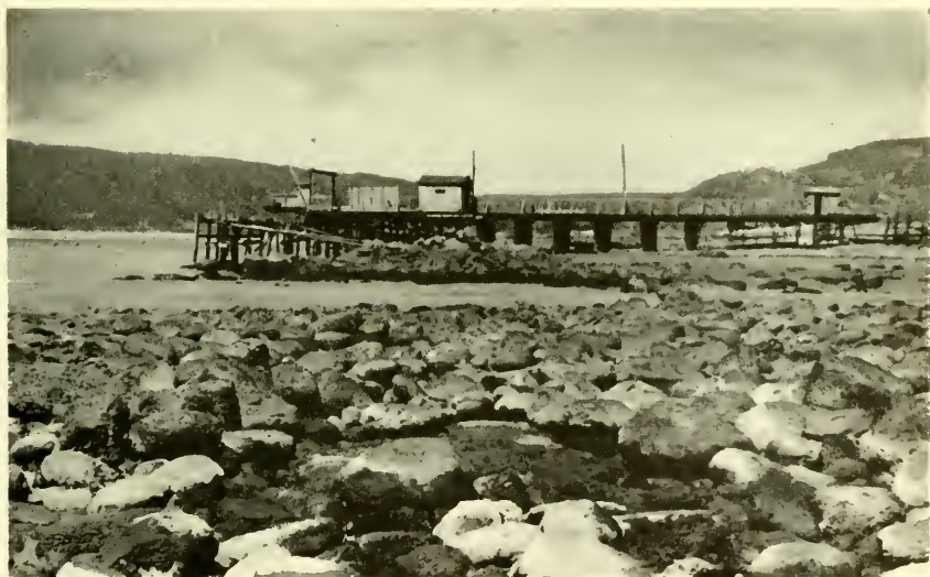
2. Dock at Lebu, here 1\frac{1}{2} meters out of water, decreased to about \frac{1}{2} meter in 5 months.
