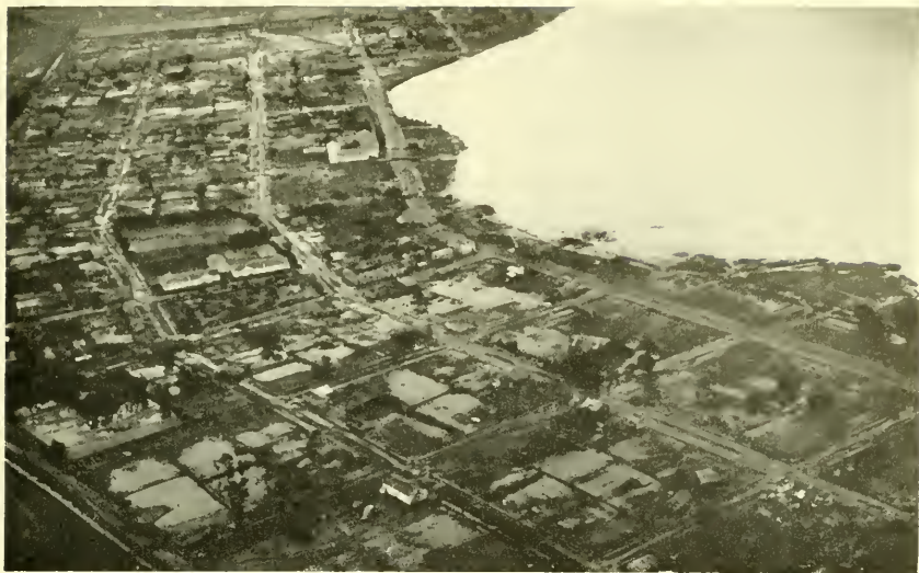
1. The tsunami washed away many houses in Puerto Saavedra. The shoreline is now 1\frac{1}{2} meters higher than before, inundating some streets.
