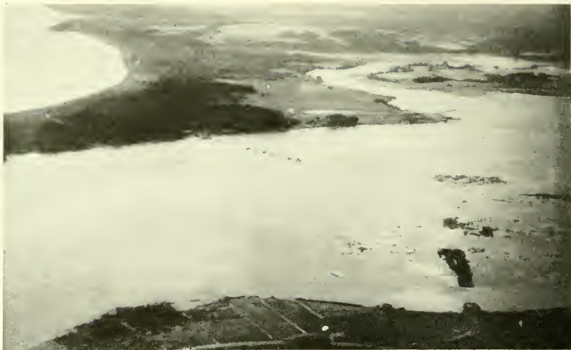
1. Mouth of the Río Pudeto, showing the effects of inundation. Note remains of bridge, the deck of which was washed away by the tidal wave, the submerged road, and the farmlands.
