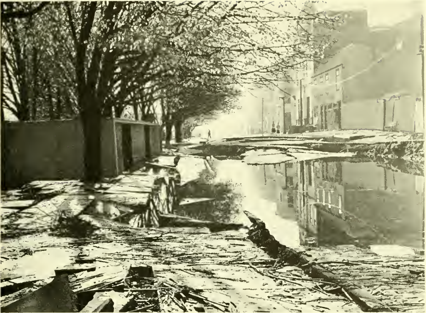
1. Damage to Malecón and park in Valdivia resulting from failure of retaining wall and artificial fill.
