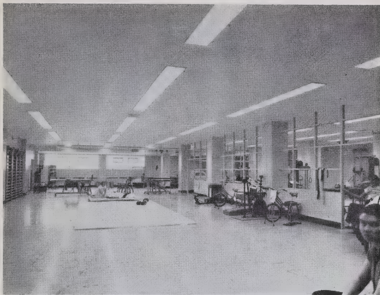
Interior of the Polio Hospital Addition, University of Alberta—Edmonton
