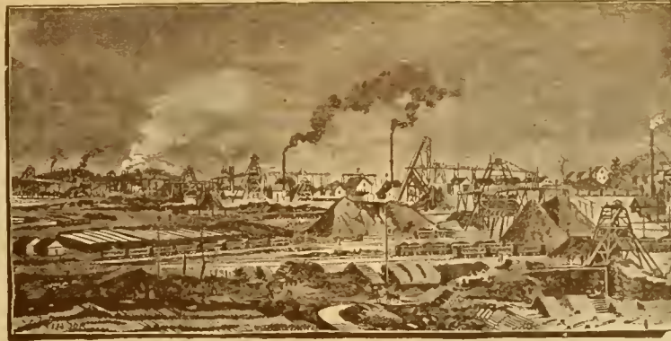
VIEW OF THE ASHLAND MINE.
