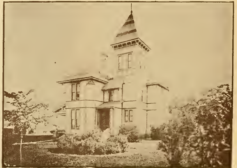
"EVERGREEN COTTAGE" RESIDENCE OF GOV. SAM S. FIFIELD.
