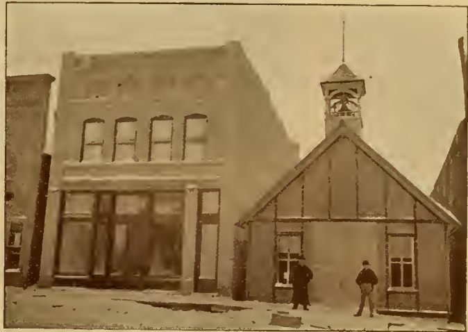
PETTINGILL BLOCK AND HOSE HOUSE.
