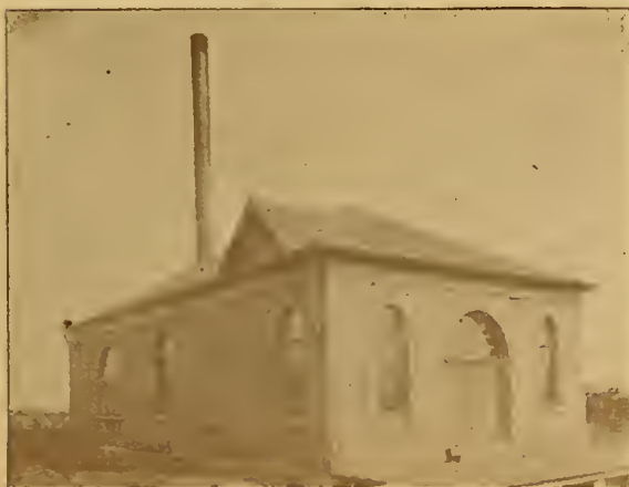
ELECTRIC LIGHTING CO. POWER HOUSE.
