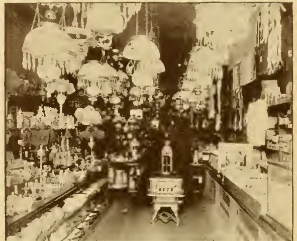
INTERIOR VIEW OF "THE RACKET," SCHUTT BROS.
