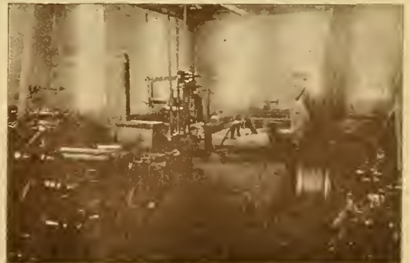
INTERIOR BEEMAN & BOWMAN'S MACHINE SHOPS.
