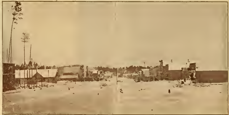
VIEW FROM DEPOT, LOOKING NORTH.
