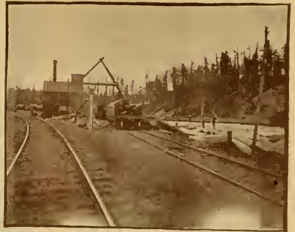
LOG HOISTING MACHINE AT BAD AND IRON RIVERS.
