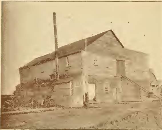
PLANING AND EXCELSIOR MILL—H. KRUSCHKE & CO.
