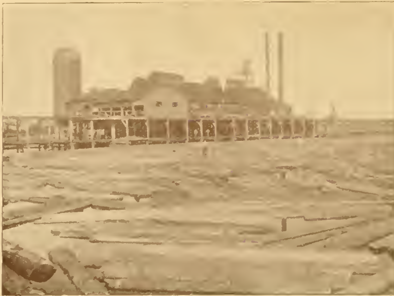
MILL OF C. C. THOMPSON LUMBER CO., WASHBURN, WIS.
