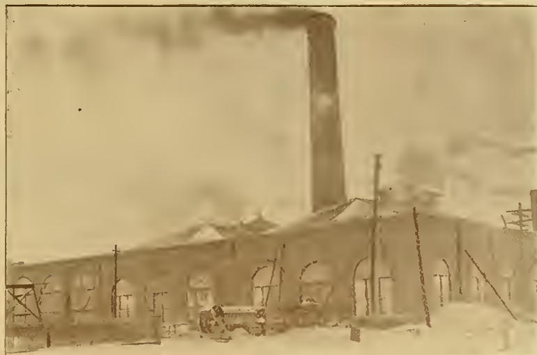
ELECTRIC POWER HOUSE—ASHLAND LIGHTING AND STREET RY. CO.
