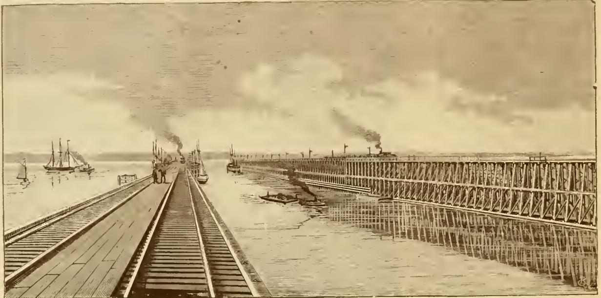
MILWAUKEE, LAKE SHORE & WESTERN ORE DOCKS, 2,521 AND 2,272 FEET IN LENGTH RESPECTIVELY.
