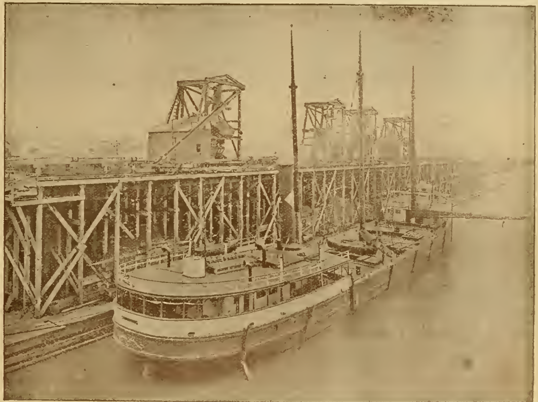
UNLOADING COAL AT THE L. S. COAL CO.'S DOCKS.
