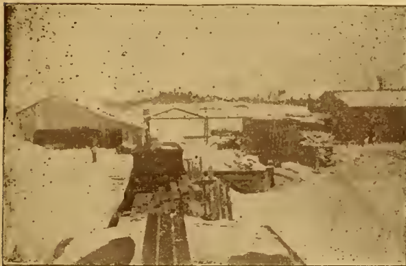
EXTERIOR BOHN MANUFACTURING CO., IRON RIVER, WIS.
