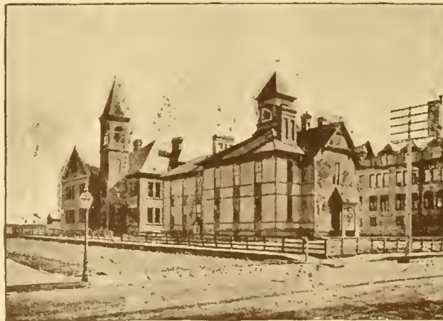
THE HIGH SCHOOL BUILDINGS.
