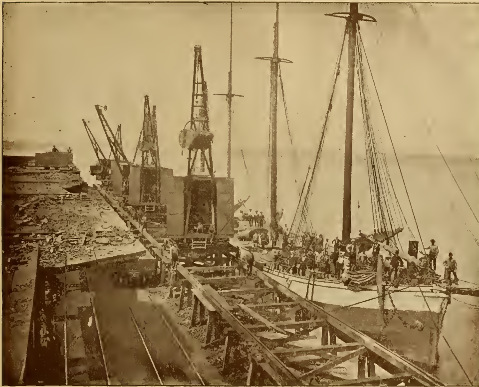
UNLOADING COAL AT THE OHIO COAL CO. DOCK, ASHLAND, WIS.
