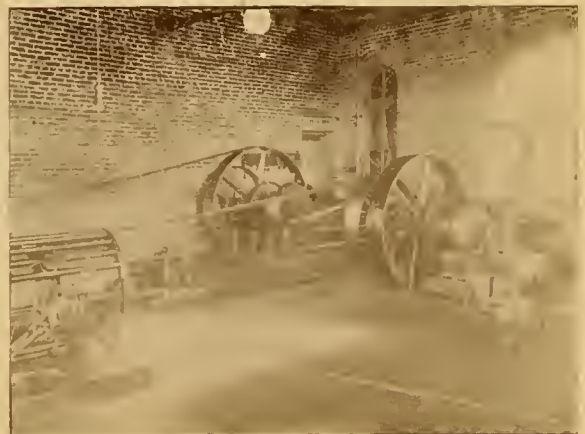
INTERIOR ELECTRIC LIGHTING CO. POWER HOUSE.
