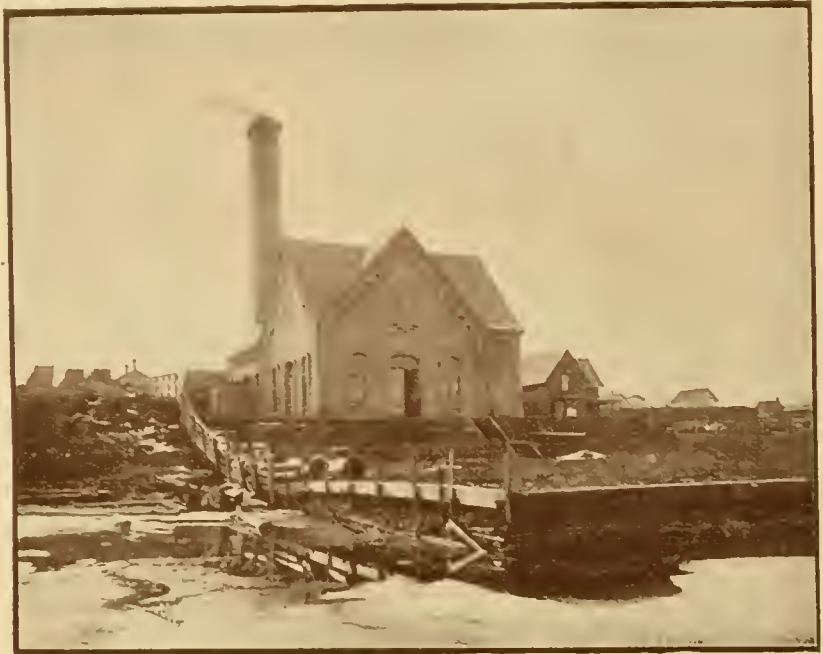
PUMPING STATION—ASHLAND WATER CO.
