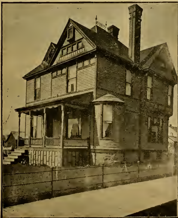
RESIDENCE OF J. SCOTT ELLIS.
