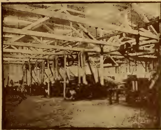
INTERIOR OF PLANING MILL.
