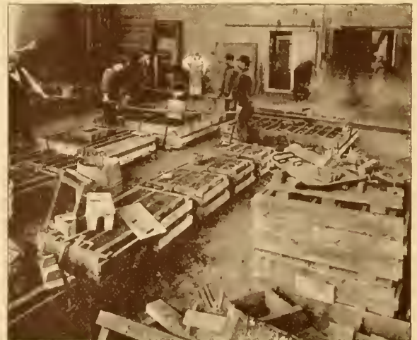
INTERIOR OF CASTING ROOM.
