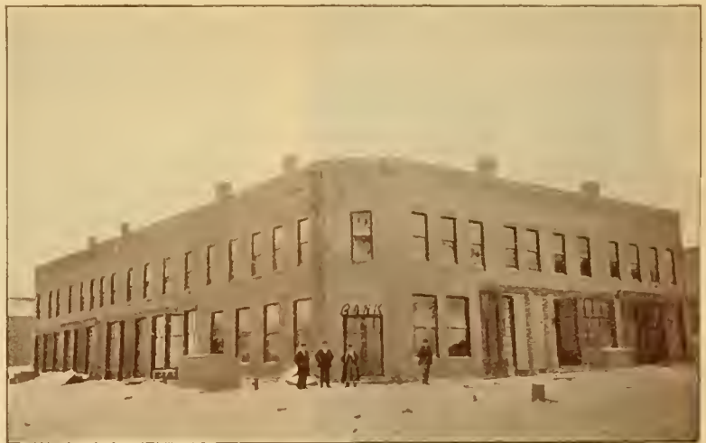
MCCORD BLOCK—BANK OF IRON RIVER.
