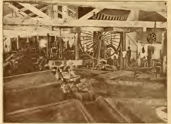
INTERIOR MILL—SHORES LUMBER CO.
