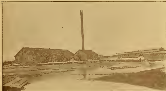
MILL AND ENGINE HOUSE, NORTH WISCONSIN LUMBER CO.
