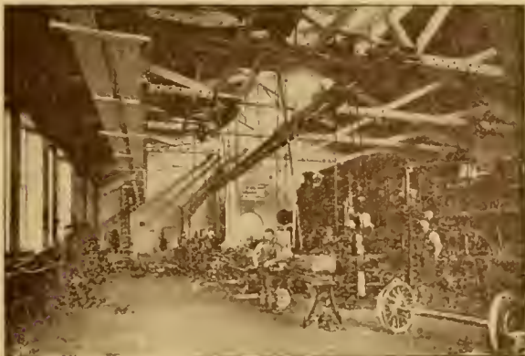
INTERIOR VIEW OF THE MACHINE SHOPS.
