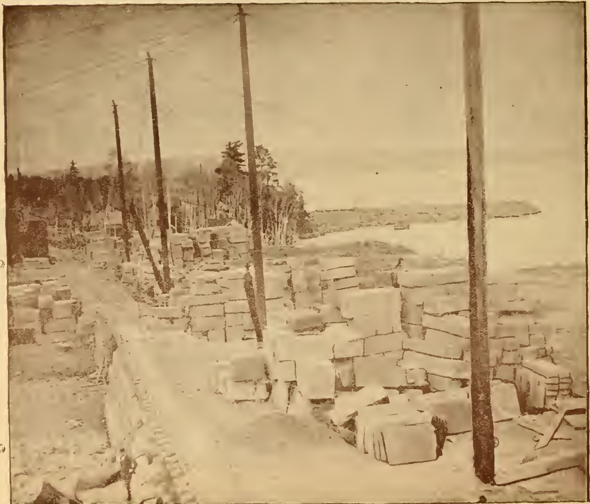
QUARRY NO. 2, PRENTICE BROWNSTONE COMPANY.
