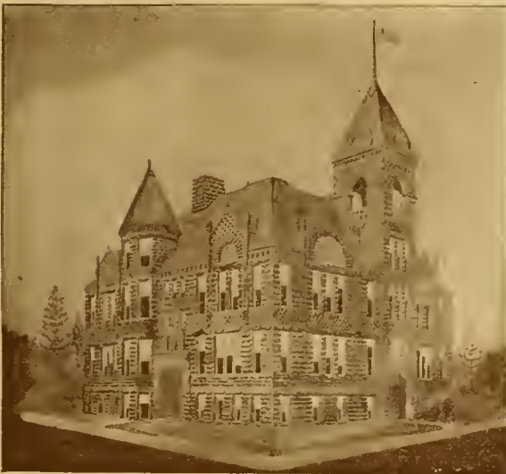
NEW BROWNSTONE PUBLIC SCHOOL BUILDING
