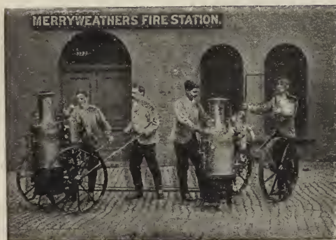
Showing Engine in transit and off Carriage for Work.
