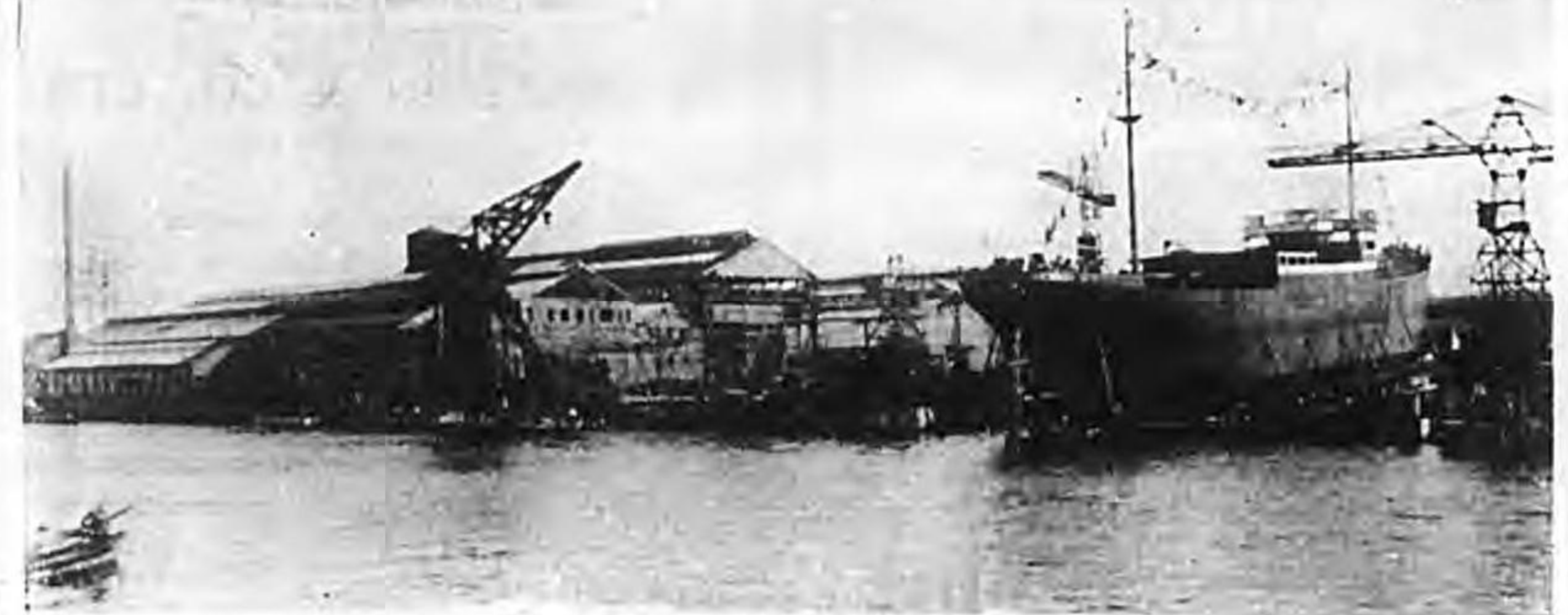
General View of Head Works, Tokyo
