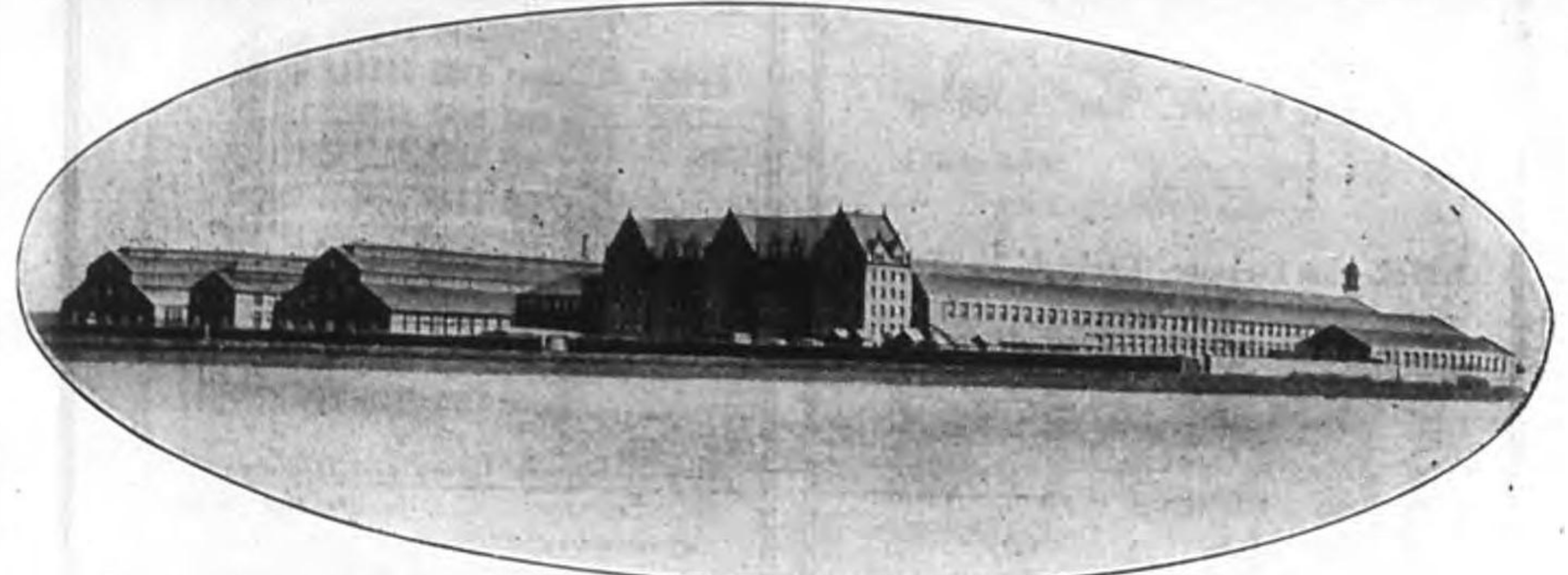
TRAFFORD PARK WORKS
