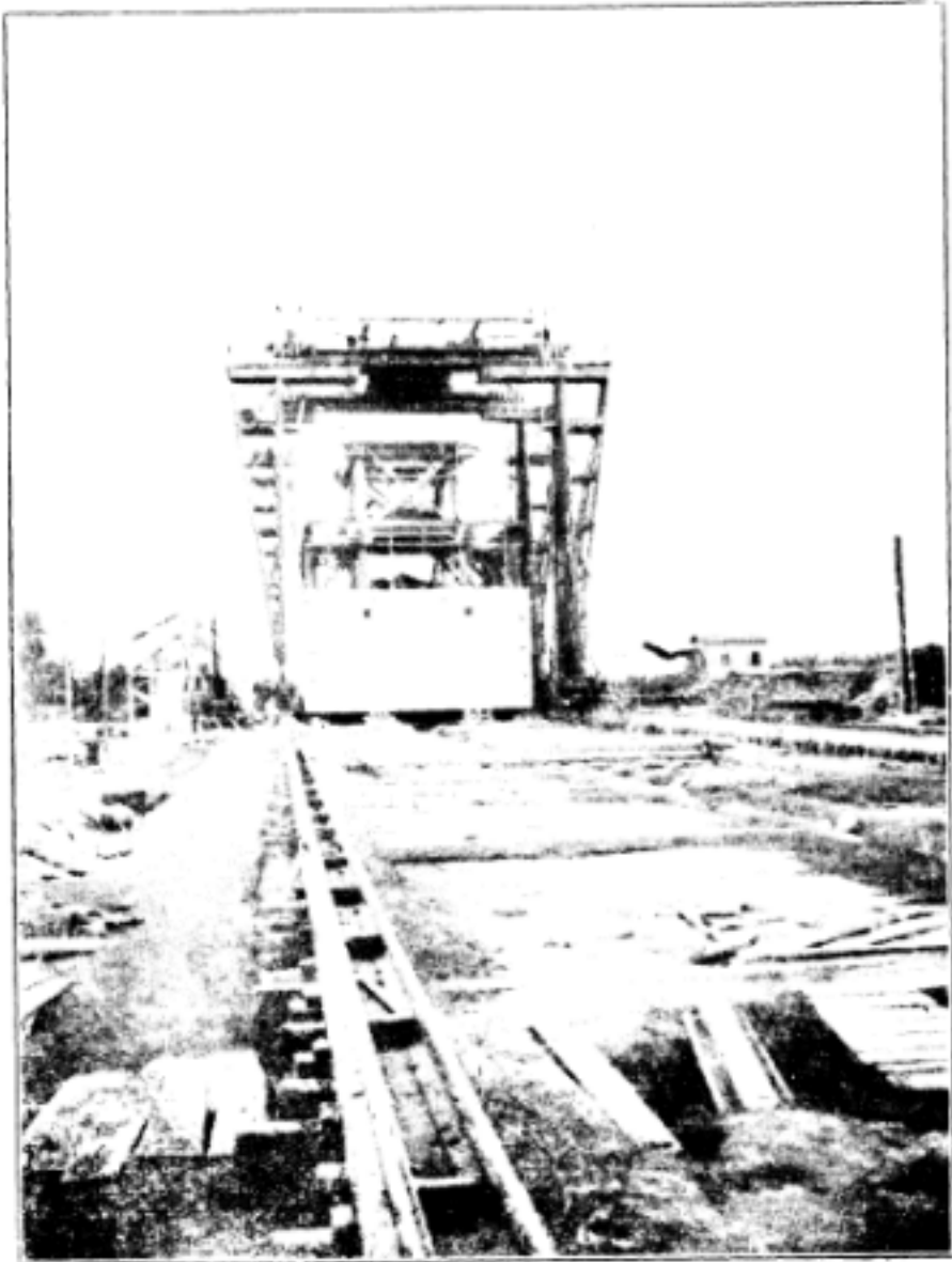
CAISSON WITH HIGH CRIB WALLS.
