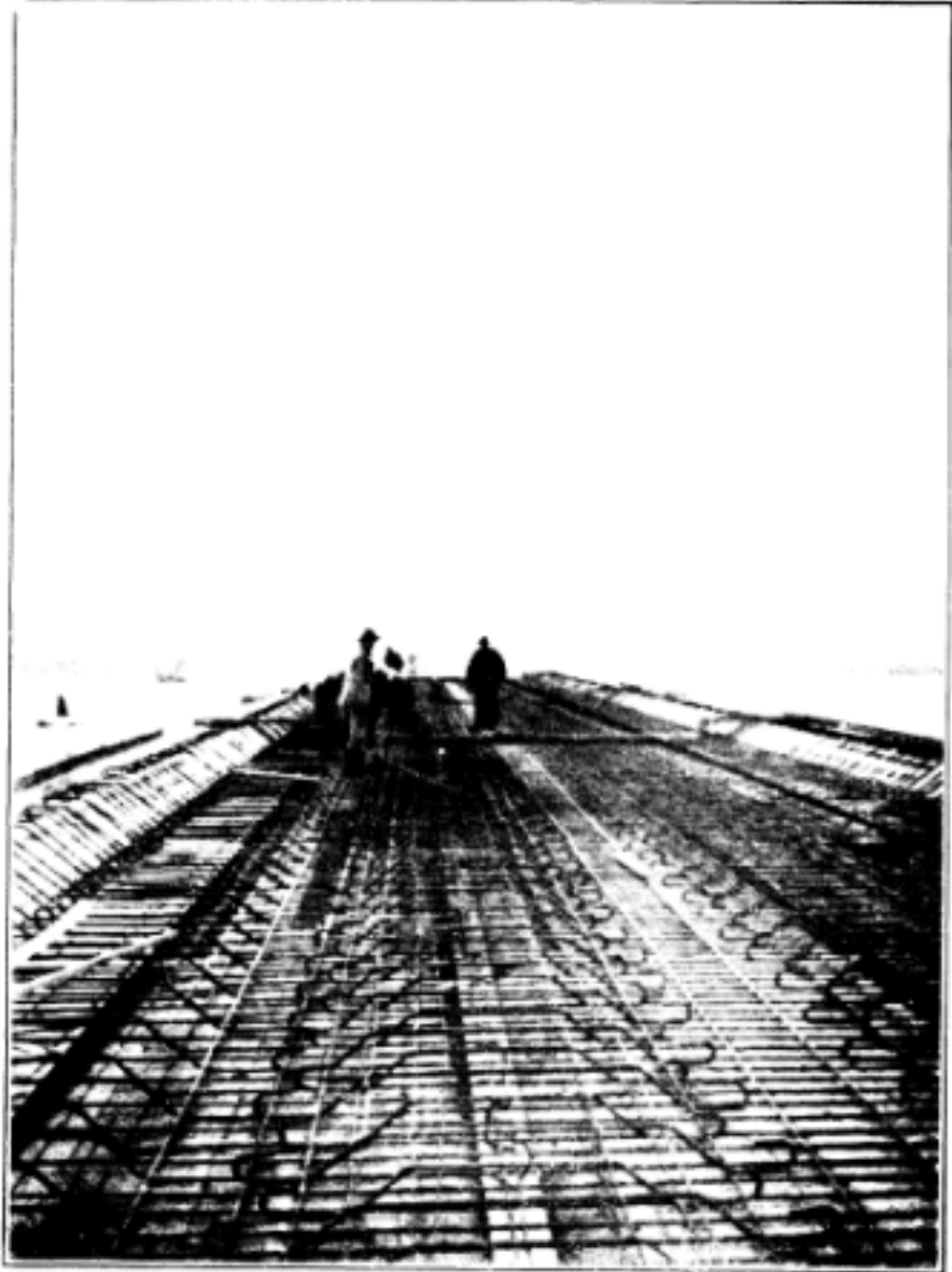
ROADWAY DECK OVER MAIN SPAN.
