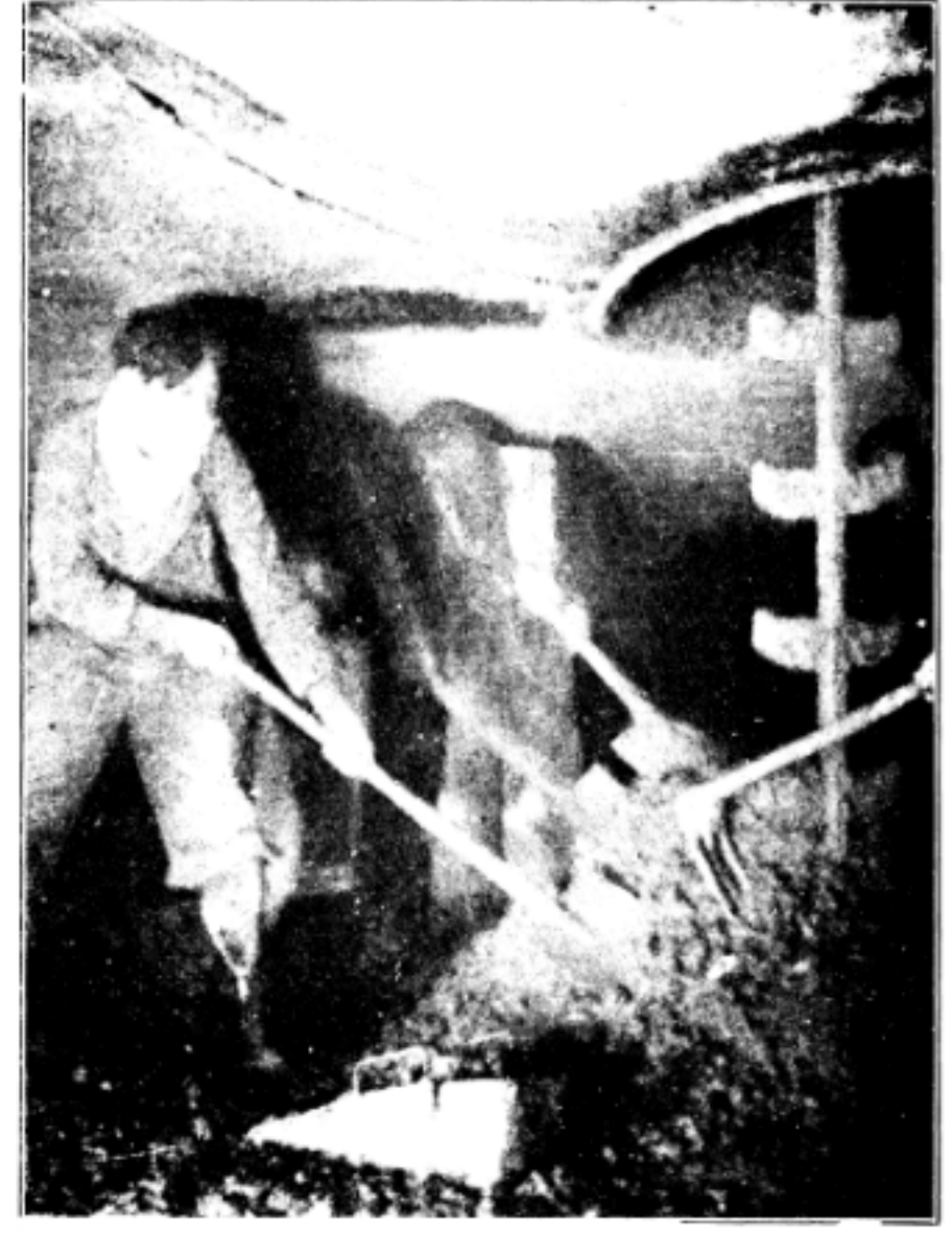
REMIXING CONCRETE IN WORKING CHAMBER
