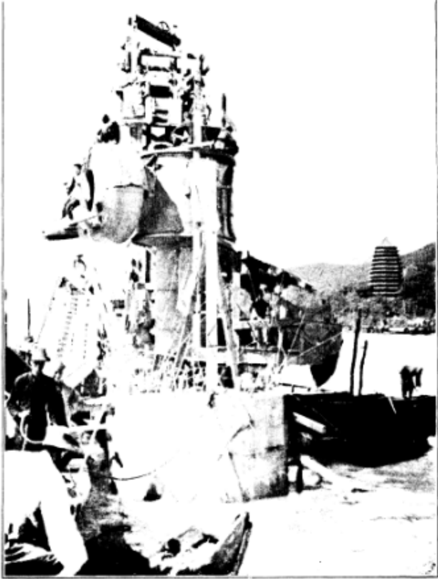
SEALING WORKING CHAMBER OF CAISSON.
