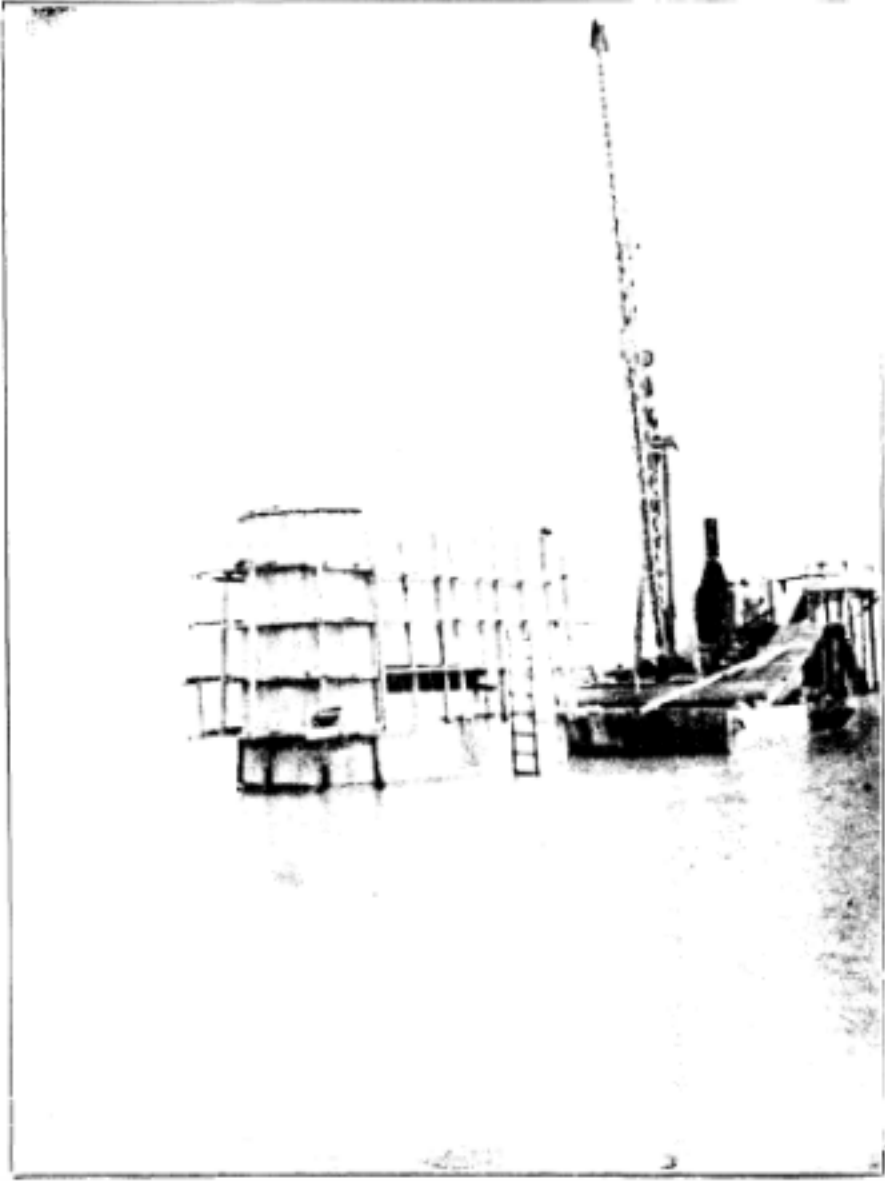
CASTING LAST SECTION OF PIER SHAFT.
