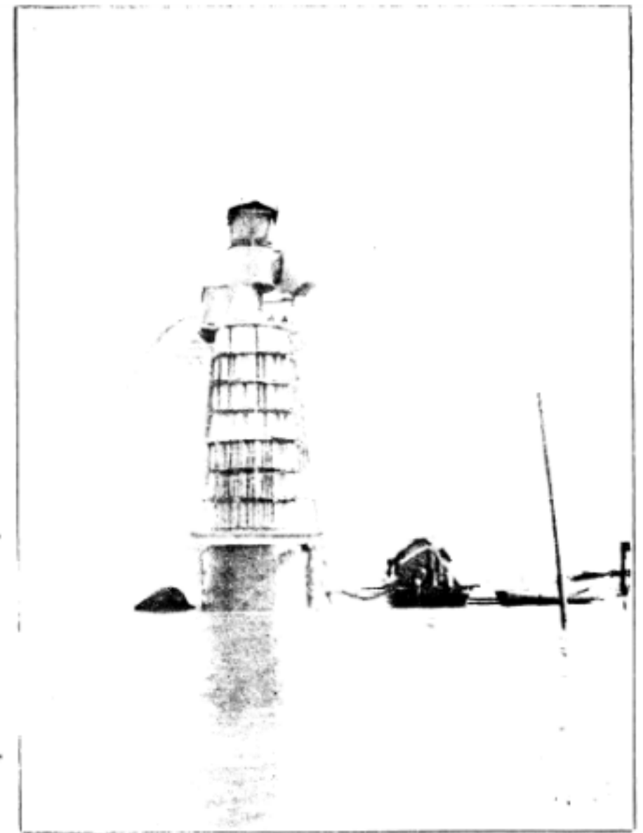
EXCAVATION BY HYDRAULIC EJECTING PROCESS.
