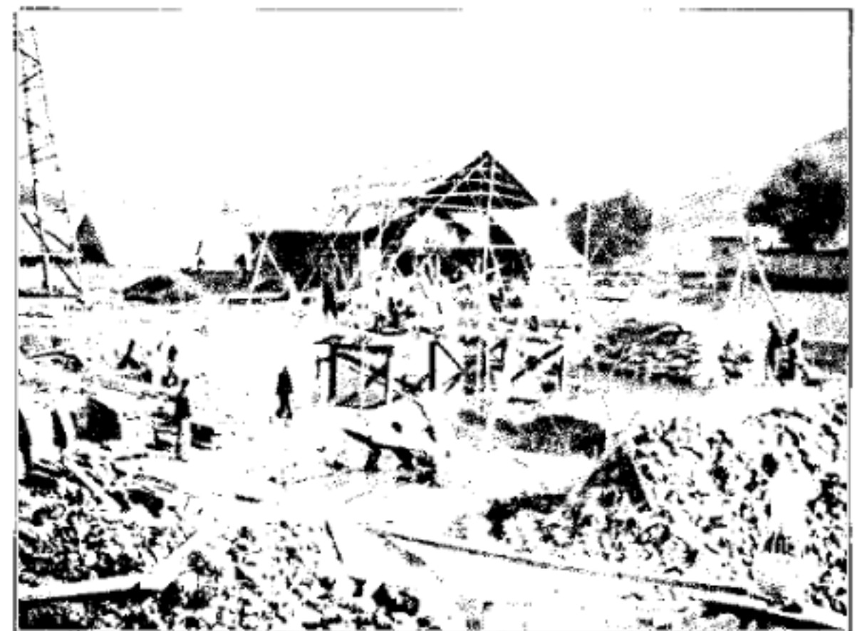
OPEN CAISSONS OF NORTH ABUTMENT.
