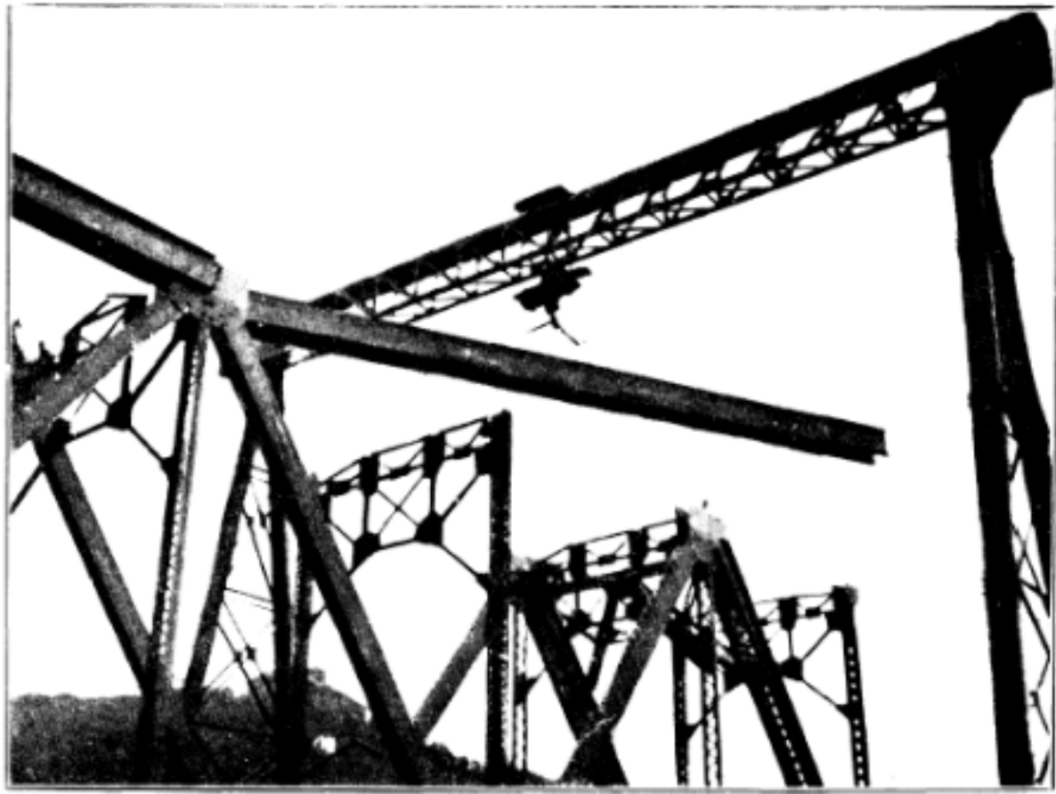
HOISTING TOP CHORD.
