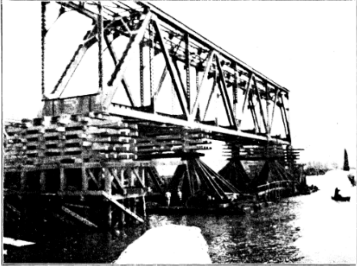
BARGES UNDER STEEL SPAN.
