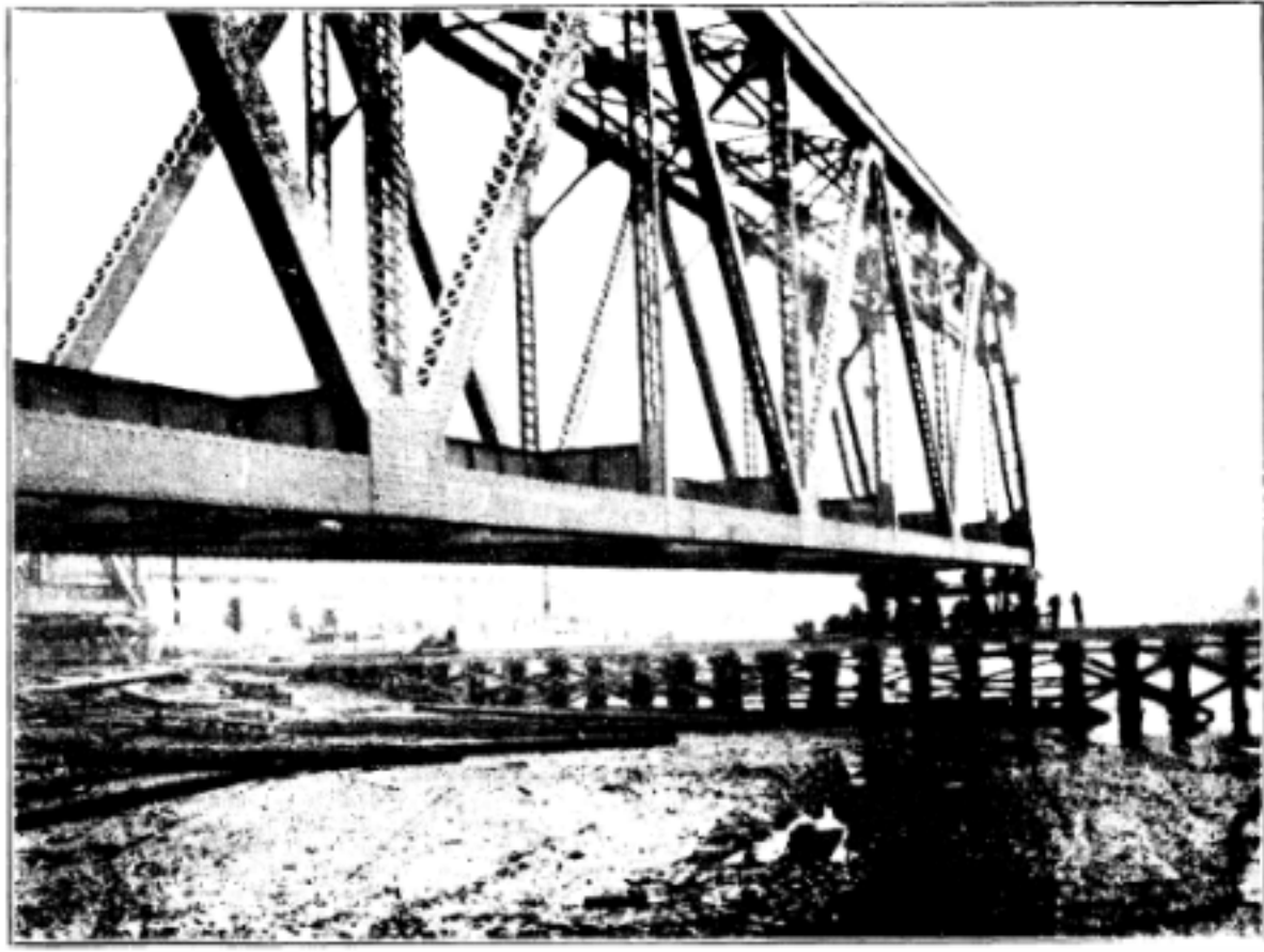
STEEL SPAN DURING TRANSPORT.
