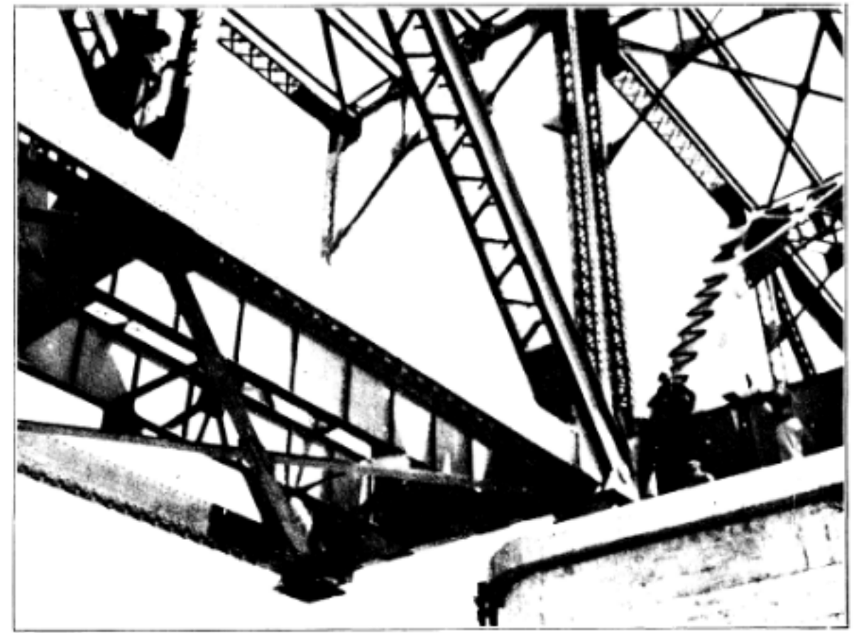
"SANDWICHING" A STEEL SPAN BETWEEN ERECTED ONES.
