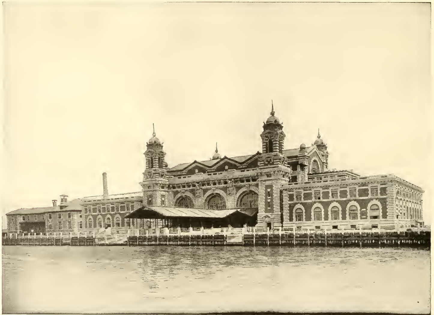
IMMIGRANT STATION. These fine buildings of brick, stone and terra cotta are located on Ellis Island, a small island between the Liberty Statue and the Communipaw shore. Here thousands of immigrants are received daily and passed into the United States. All steerage passengers are transferred from the steamers in which they arrive, and before they can land, must be examined as to their eligibility as citizens and be fully recorded. The Government never ceases to protect the immigrant until he is prepared to face the new conditions. Over 11,000,000 immigrants have entered the port of New York since 1880, and the annual average is about 600,000.
