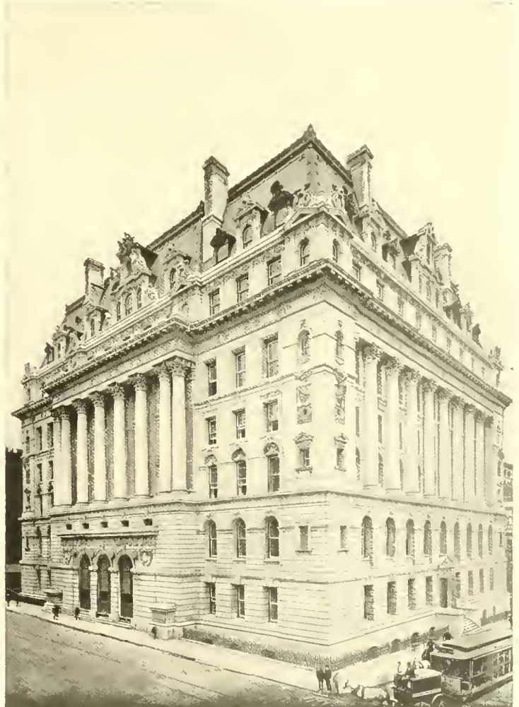
HALL OF RECORDS. Chambers, Reade and Center Streets. A splendid fire-proof structure built of steel and Maine granite, for the safe-keeping of real estate deeds, mortgages, etc., of Manhattan Borough, also for Surrogates' Courts and City Offices. Erected 1904, and cost $5,000,000.
