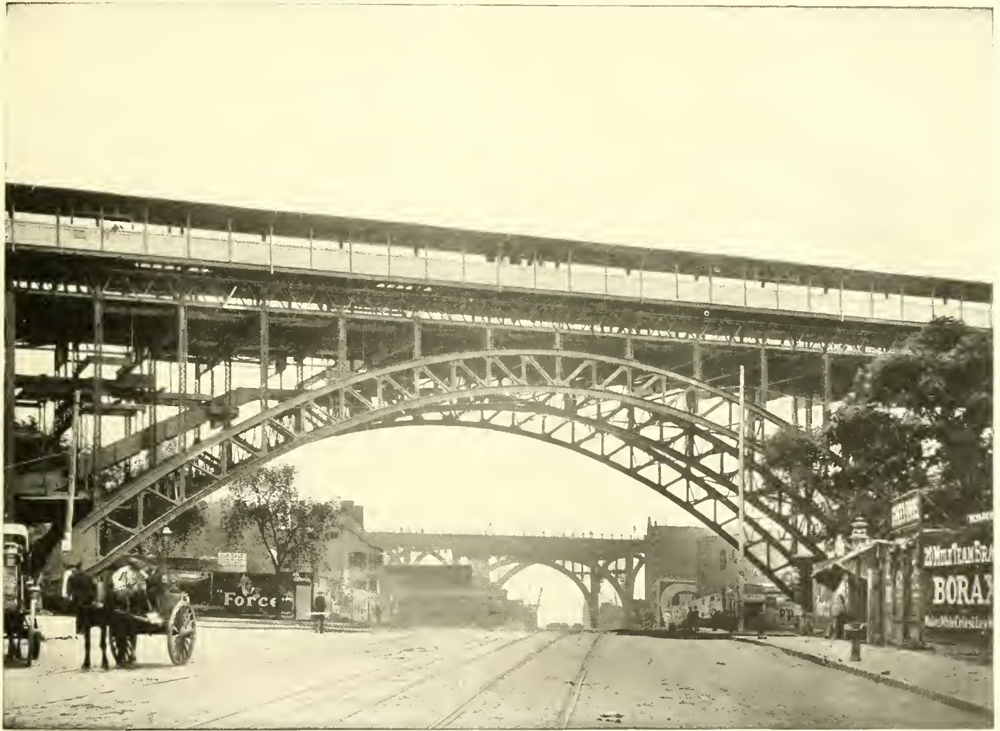
MANHATTAN VIADUCT, Manhattanville. At 125th Street the West Side line of the underground rapid transit system emerges from the subway and crosses the Manhattan valley on a great flying-arch steel viaduct to 135th Street, where it again enters the tunnel, and at 190th Street is more than 100 feet below the surface. The Manhattan Viaduct is a splendid example of American bridgework, and in common with all sections of this greatest engineering feat of the new century, is built to last for all time under the severest strains.
