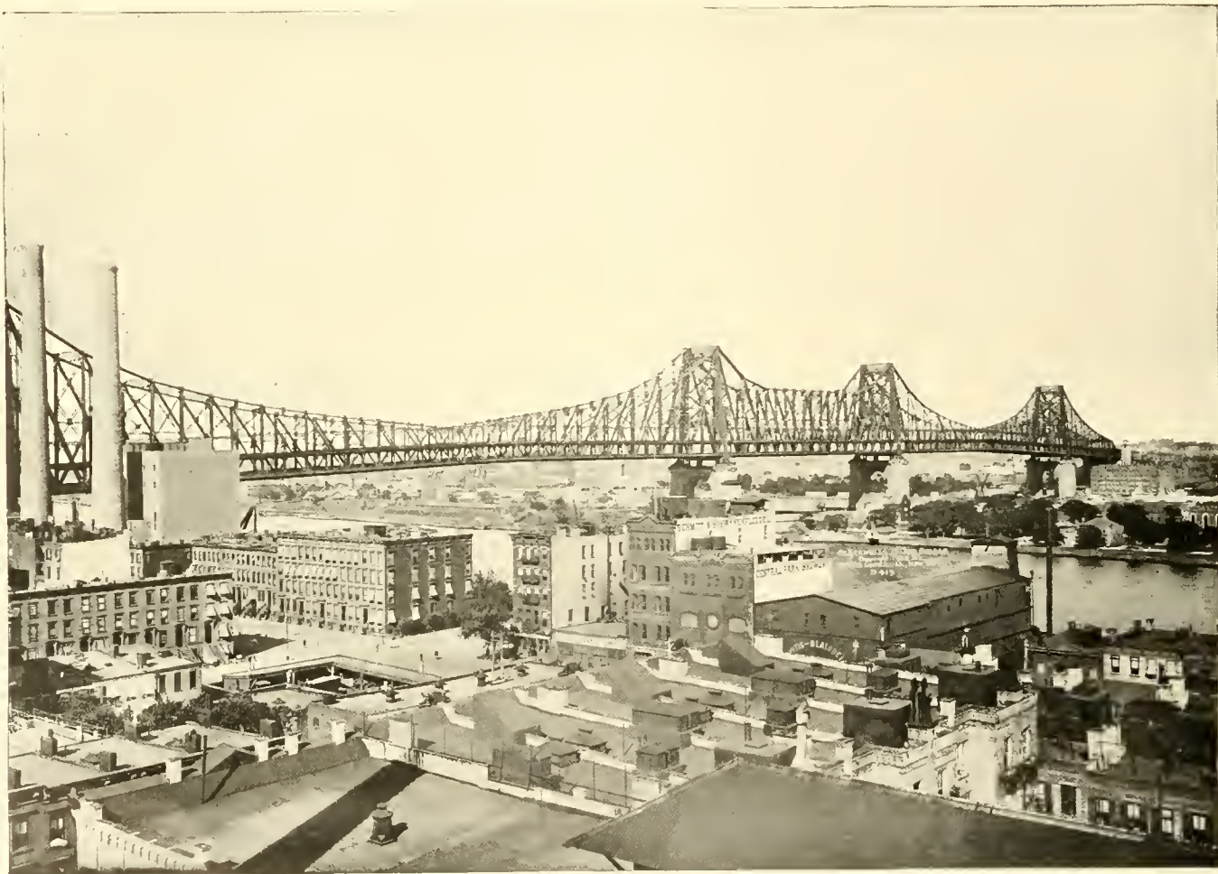
BLACKWELL'S ISLAND BRIDGE. This splendid example of cantilever bridge construction spans the East River from East 59th Street and 2d Avenue to Jane and Academy Streets, Long Island City. The bridge is supported by six masonry piers with a clear height over channels of 135 feet. Longest span 1182 feet. The entire structure is nearly 7700 feet in length—the longest bridge spanning the East River. It is provided with a roadway 53 feet wide, 4 trolley lines, 2 railroad tracks and 2 promenades. The bridge was completed in 1908 at a cost of over $25,000,000.
