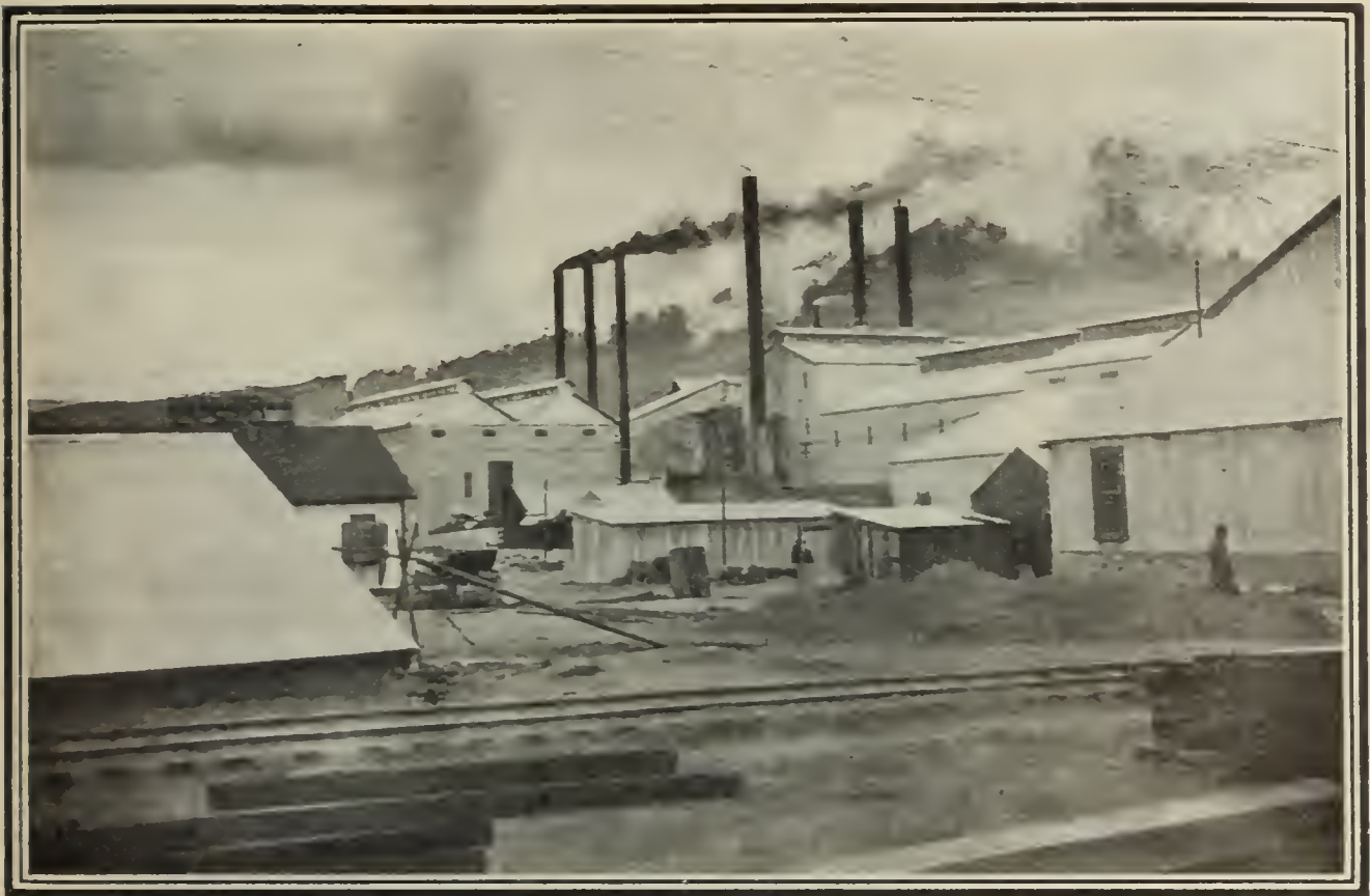
AQUEDUCT CONCRETE PLANT BUILT BY THE CITY OF LOS ANGELES
