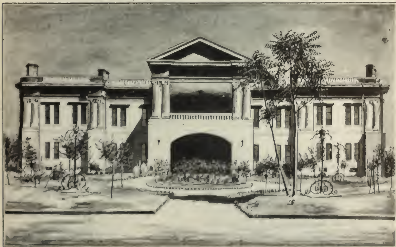
HOME OF CHINA'S STATE DEPARTMENT THE NEW WAIWUPU BUILDING, AT PEKING
