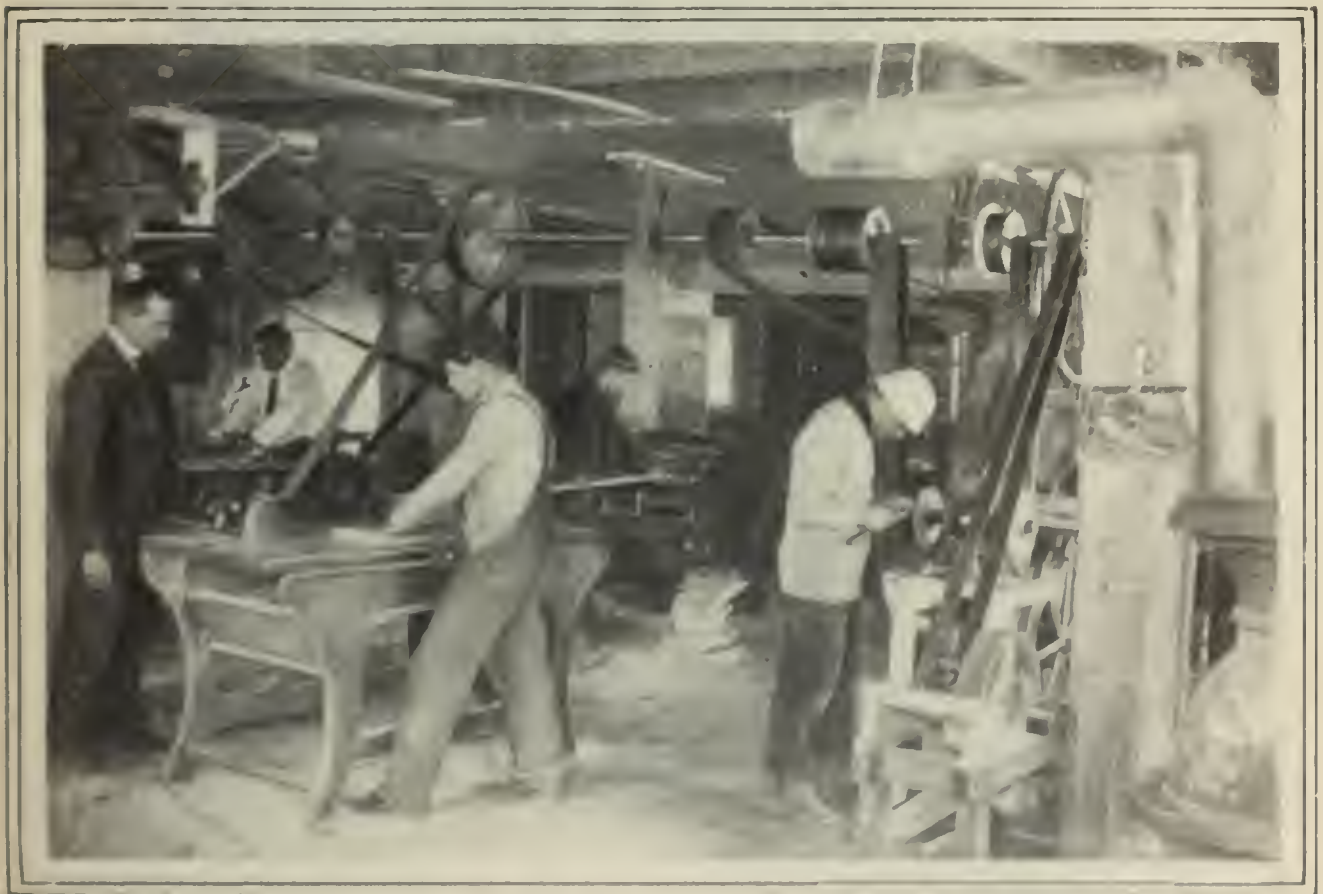
IN THE WORKING SHOP
