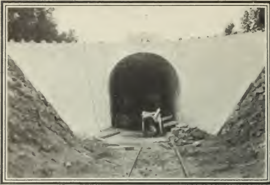
OUTLET OF THE AQUEDUCT INTO DRY CANYON RESERVOIR
