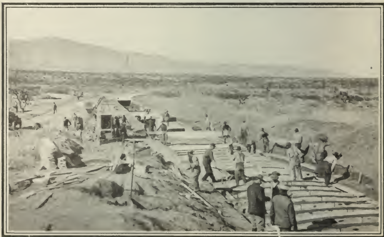
PUTTING THE CONCRETE COVER ON THE CONDUIT IN THE MOJAVE DESERT
