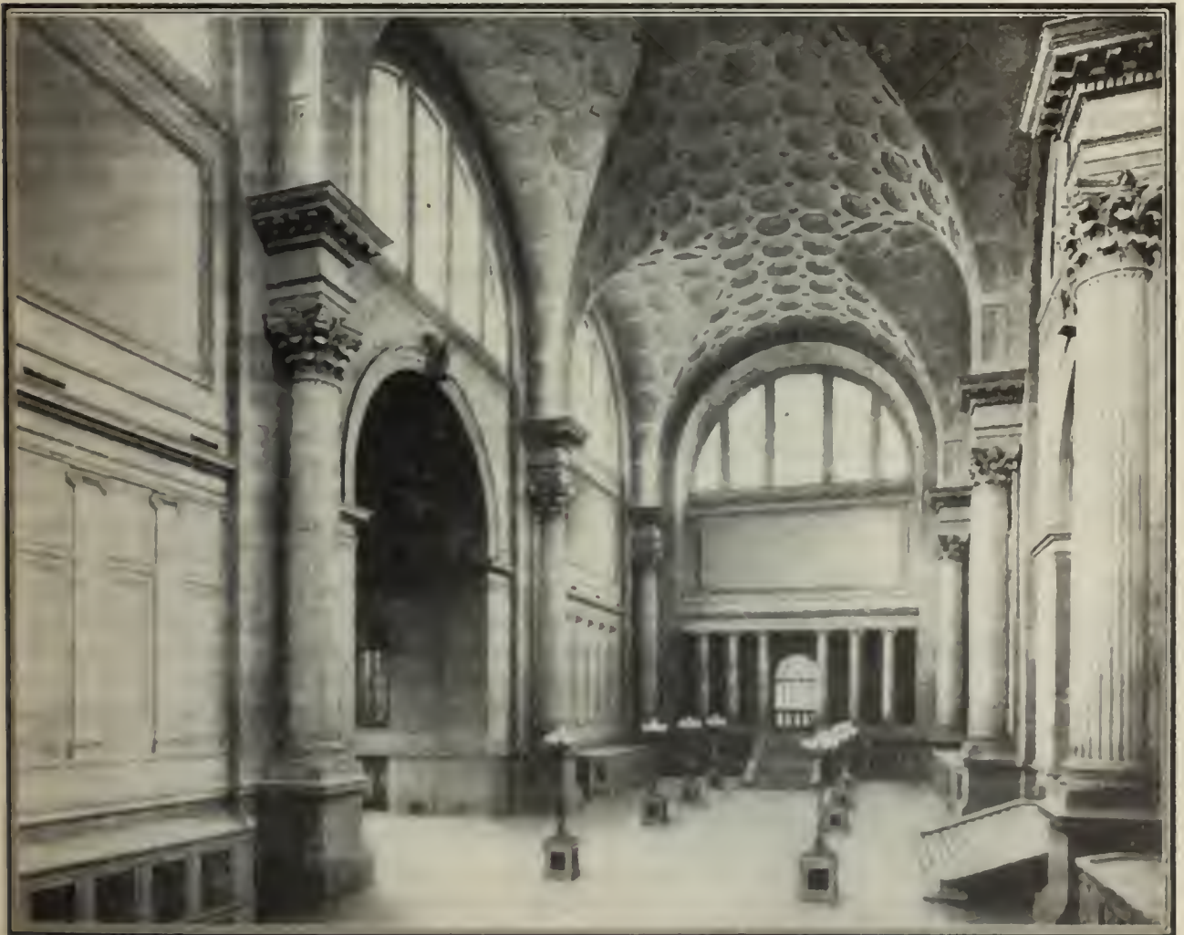
THE SPACIOUS PENNSYLVANIA WAITING ROOM
