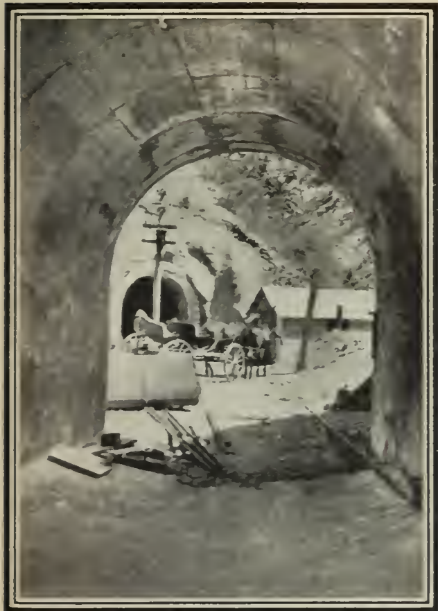
TWO OF THE FINISHED TUNNELS IN THE SAUGUS DIVISION
