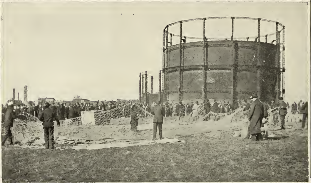
STRETCHING THE NETTING OVER THE BIG BAG. THE GAS TO FILL THE BALLOON IS TO BE FED FROM THE GAS-RESERVOIR NEAR BY.
