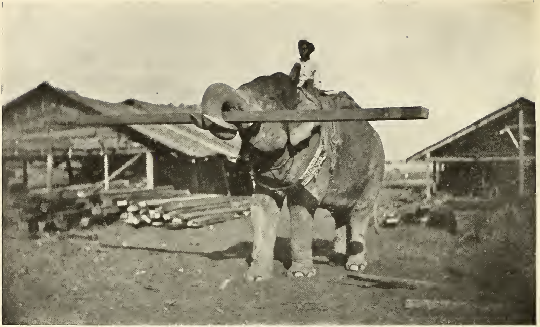
AN INDEPENDENT WORKER CARRYING A BEAM TO THE STACK.
