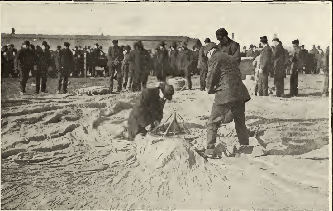
SCREWING THE VALVE-RINGS TOGETHER ON THE FABRIC.
