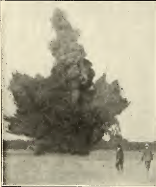
EXPLOSIVES APPLIED TO A HUGE STUMP AND ROOTS OF A TREE.
