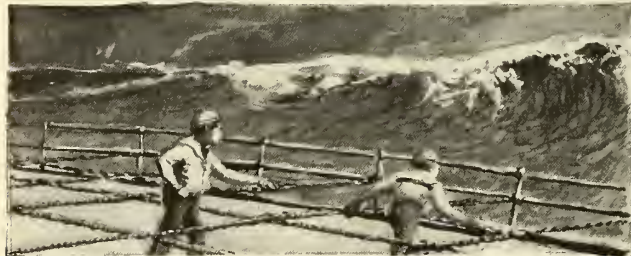
"THE LIFE-LINES WERE WOVE FROM RAIL TO STANCHIONS."
