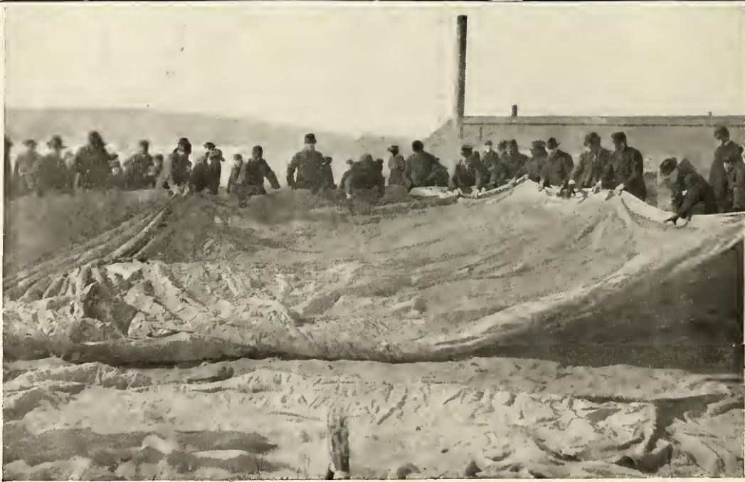
STRETCHING THE FABRIC OUTWARD FROM THE VALVE-HOLE IN THE CENTER.
