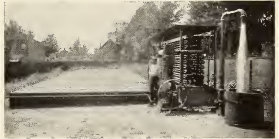
PUMPING WATER BY POWER FROM THE HEAT OF THE SUN.
