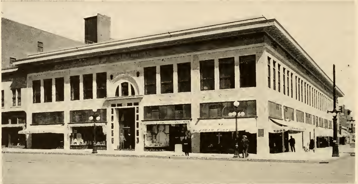
STRATTON STORE BUILDING, COLORADO SPRINGS, COLORADO
