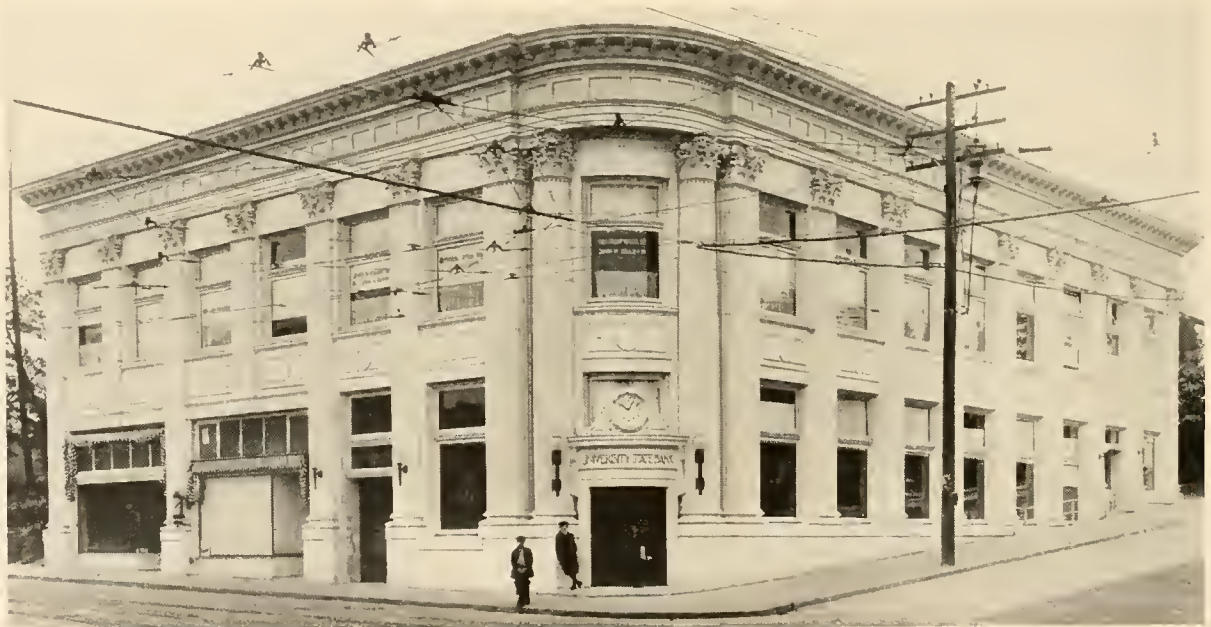
UNIVERSITY STATE BANK BUILDING, SEATTLE, WASH.
