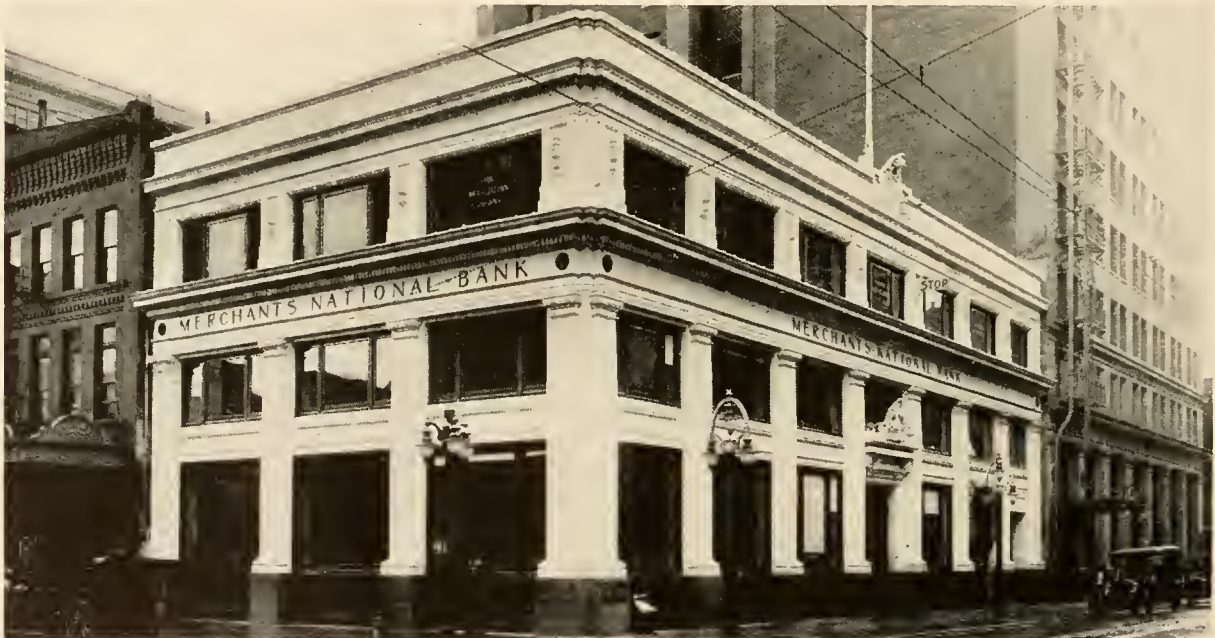
MERCHANTS NATIONAL BANK, PORTLAND, ORE.
