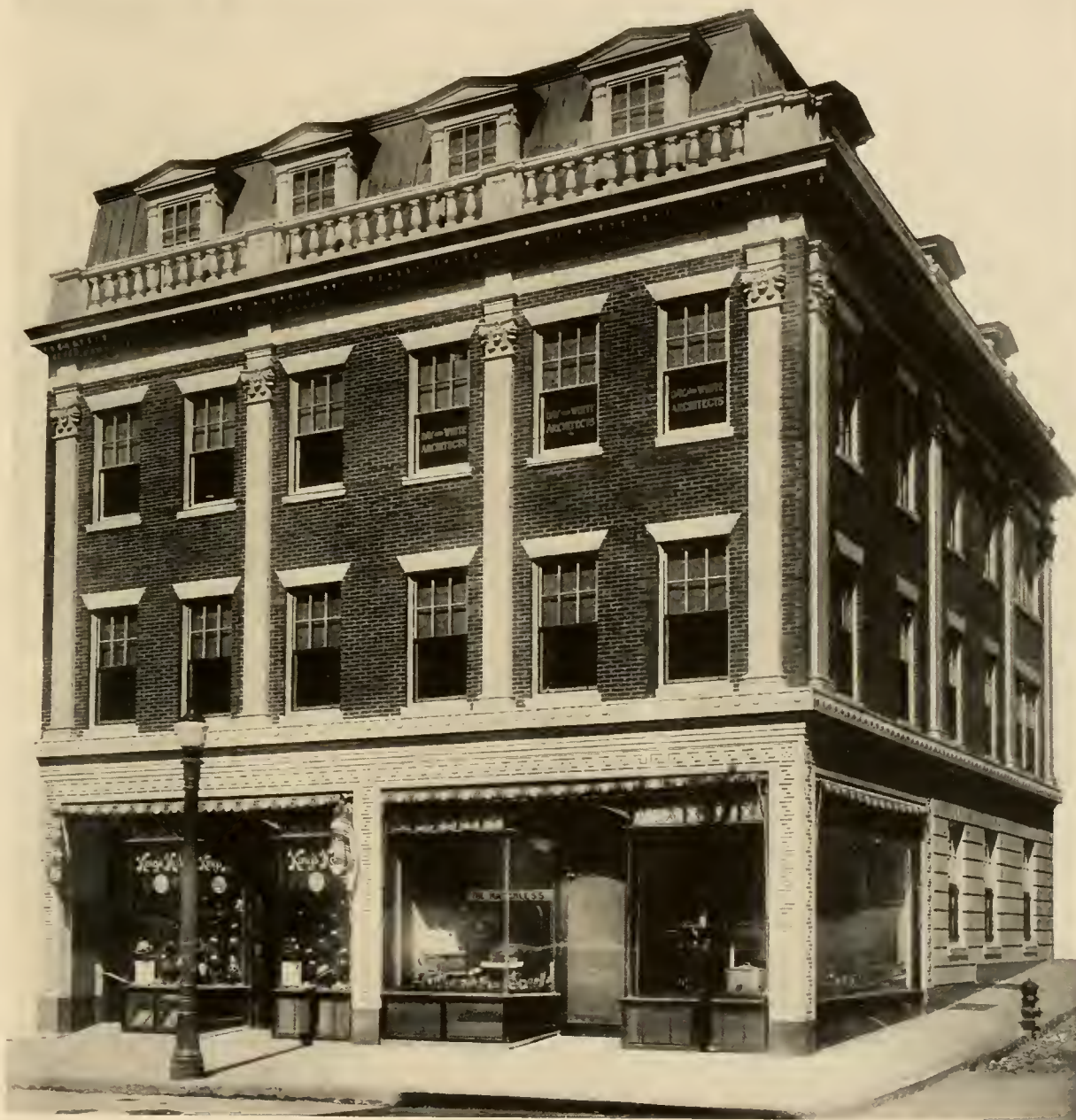
HAVERHILL ELECTRIC COMPANY BUILDING, HAVERHILL, MASS. (After rebuilding with Terra Cotta)
