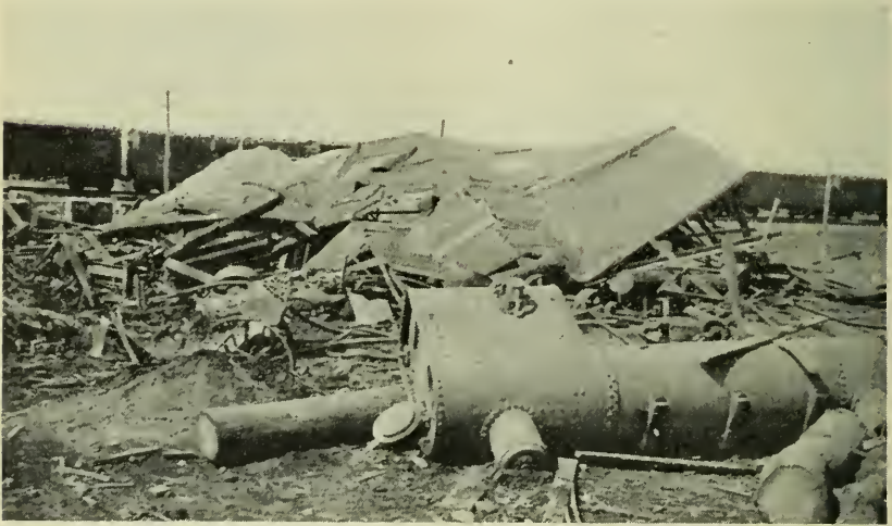
Complete destruction of a southern mill by a boiler explosion.
