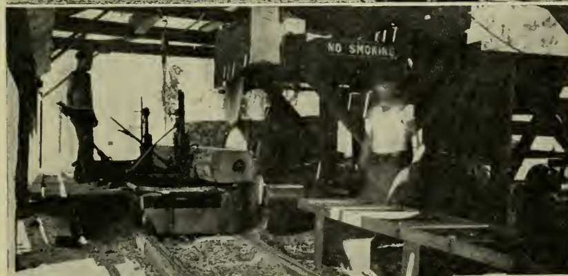
Top—The “crowning glory”—The sawmill locomotive made from parts of this and that. Center—Boiler with its open air setting and sawdust bin. Bottom—The saw carriage, showing the arrangement of two saws for extra large logs.
