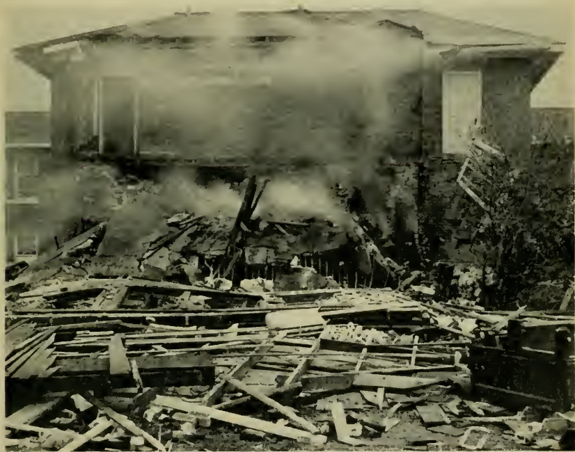
Wreckage of music room and boiler room after explosion.
