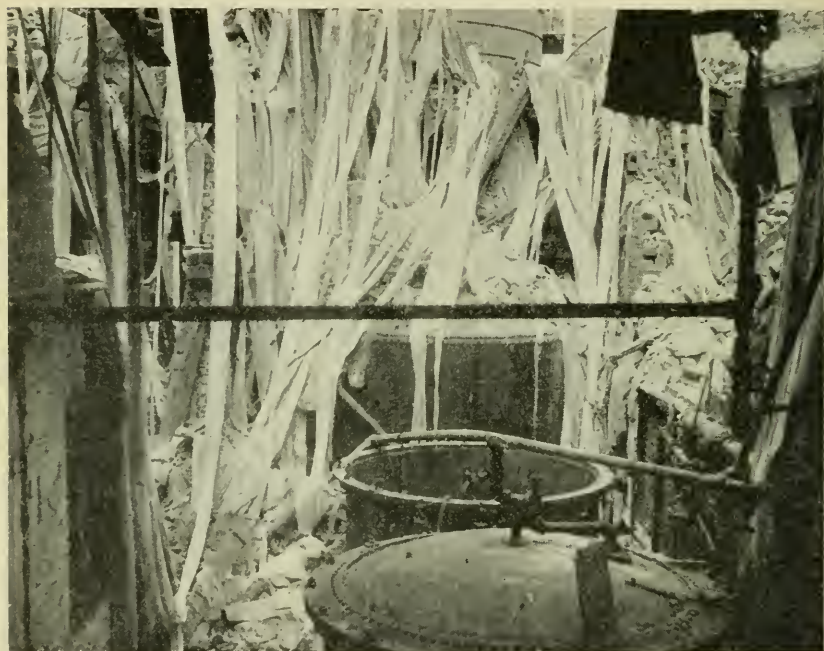
Empty kier and contents. The head landed in a nearby street.
