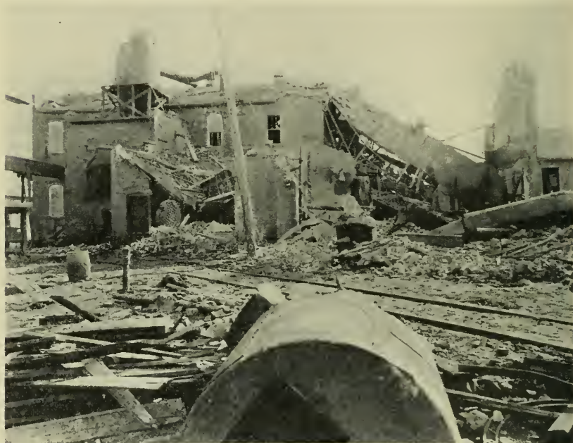
Wreckage at Hertford, North Carolina. A one-story boiler room formerly stood at the right just beyond the tracks at about the spot where the steel smokestack is lying. Near the left center of the mill building is No. 1 boiler beneath which is the engine. On the roof of the mill building at the extreme left is the rear course of the No. 2 boiler which exploded. The breeching is in the foreground.
