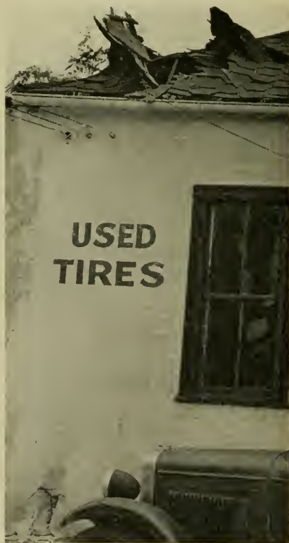
The air tank happened to go upward.
