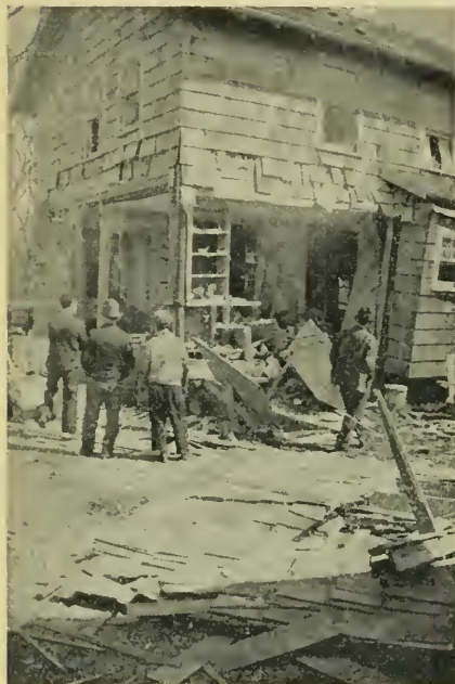
After a hot water tank exploded.
