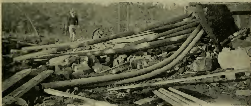
Parts of mine boiler following its explosion.
