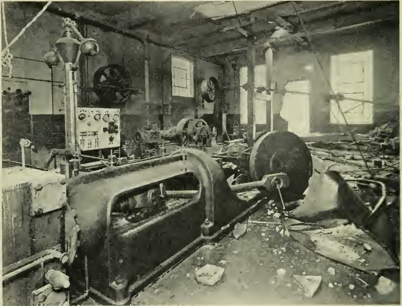
Engine room after the flywheel exploded and wrecked the engine.
