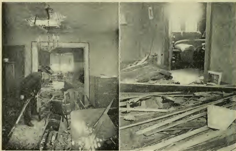
After hot water tanks hurtled upward.
