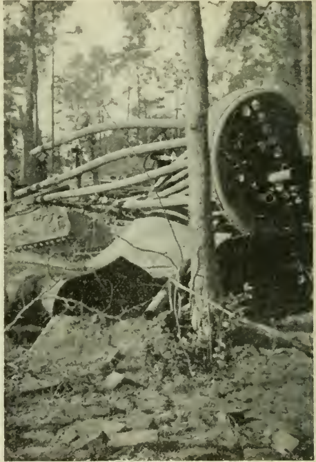
Part of exploded sawmill boiler in Georgia forest.
