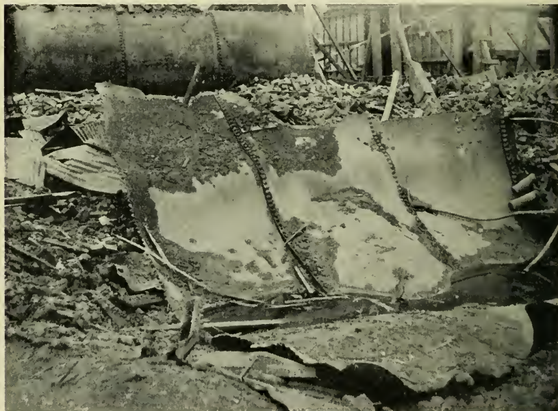
Partial view of wreckage from Georgia boiler blast.
