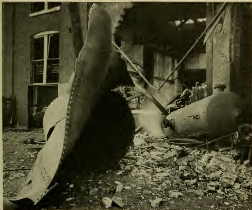
Following the ignition of lubricating oil vapor.
