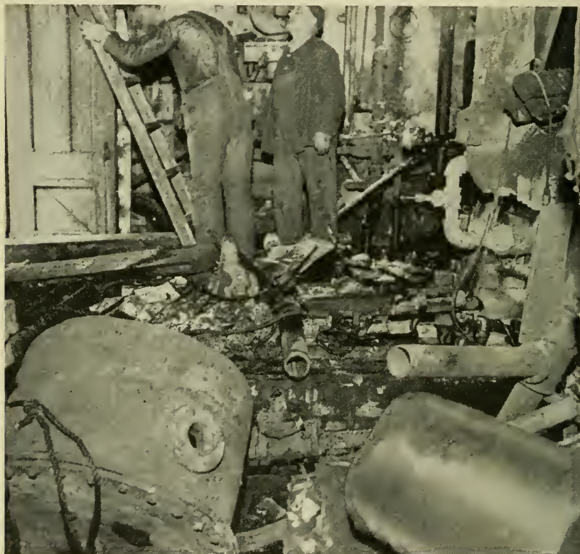
Result of cast iron blow-off tank explosion.
