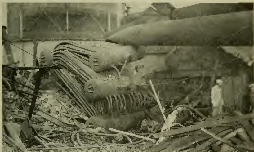
Wreckage after failure of concealed mud drum head.
