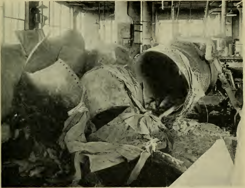
Figure 1. Remains of the vulcanizer after its explosion.
