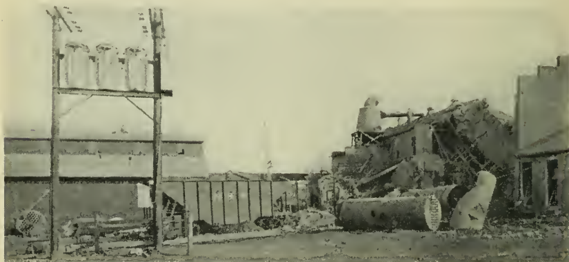
Another view of the mill at Hertford. In the foreground is No. 3 boiler and part of the stack. The front course of No. 2 boiler is shown at the extreme left where it fell after the explosion.
