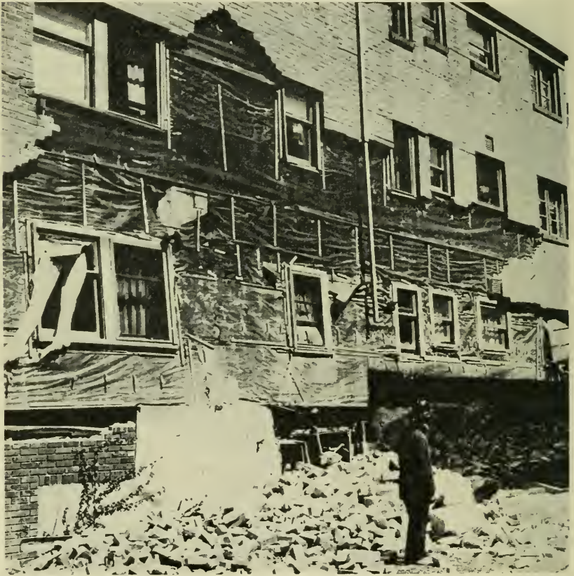
Part of $30,000 damage after heating boiler exploded in Seattle apartment.
