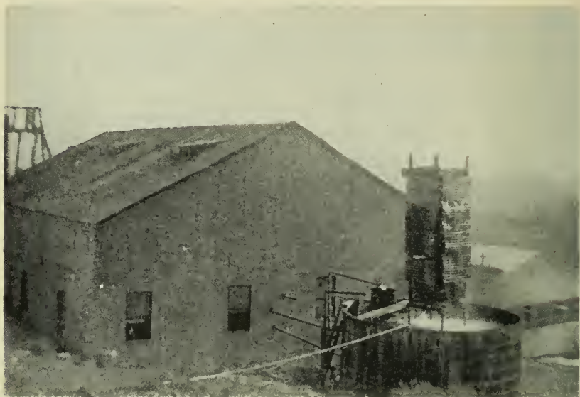
One of the mine buildings and the circulating water cooling tower. Water is carefully conserved. Even water for shower baths is saved and used in process work.
