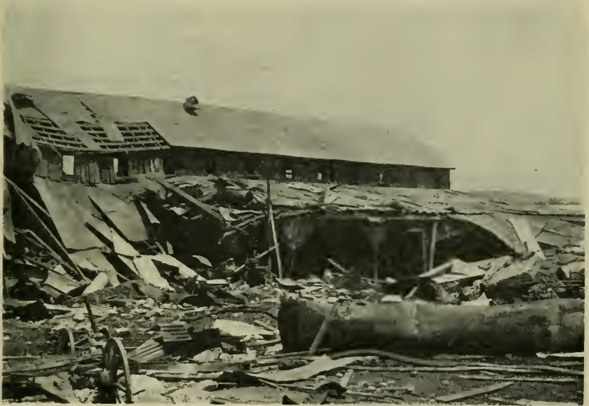
Figure 1. Result of a lap seam failure early in June.
