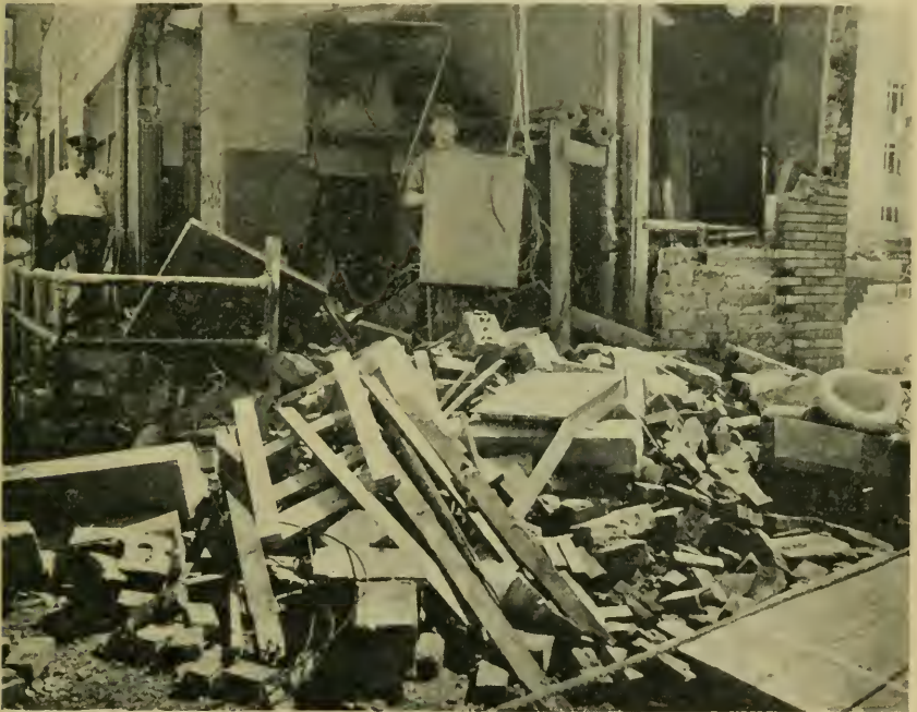
An Indiana automobile service station after a hot water heater burst.
