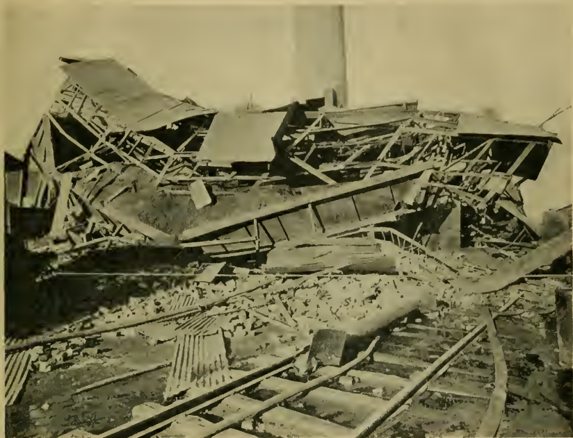
A bunker of coal collapses into the debris to complicate the search for a fireman's body.
