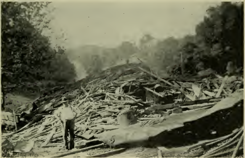
After a sawmill boiler explosion in West Virginia. The scene is typical of wreckage following this type of accident.
