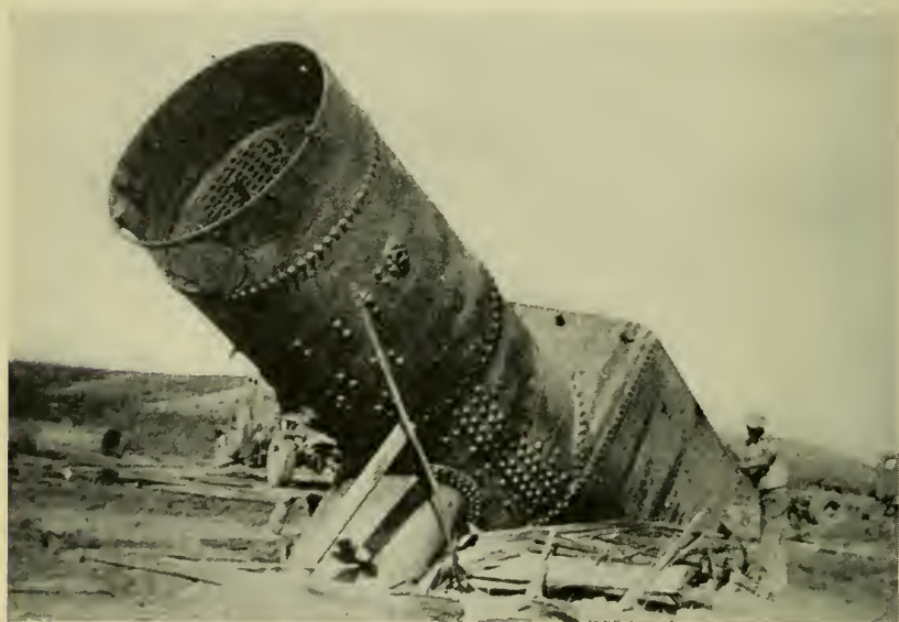
After the crown sheet pulled off its stays.
