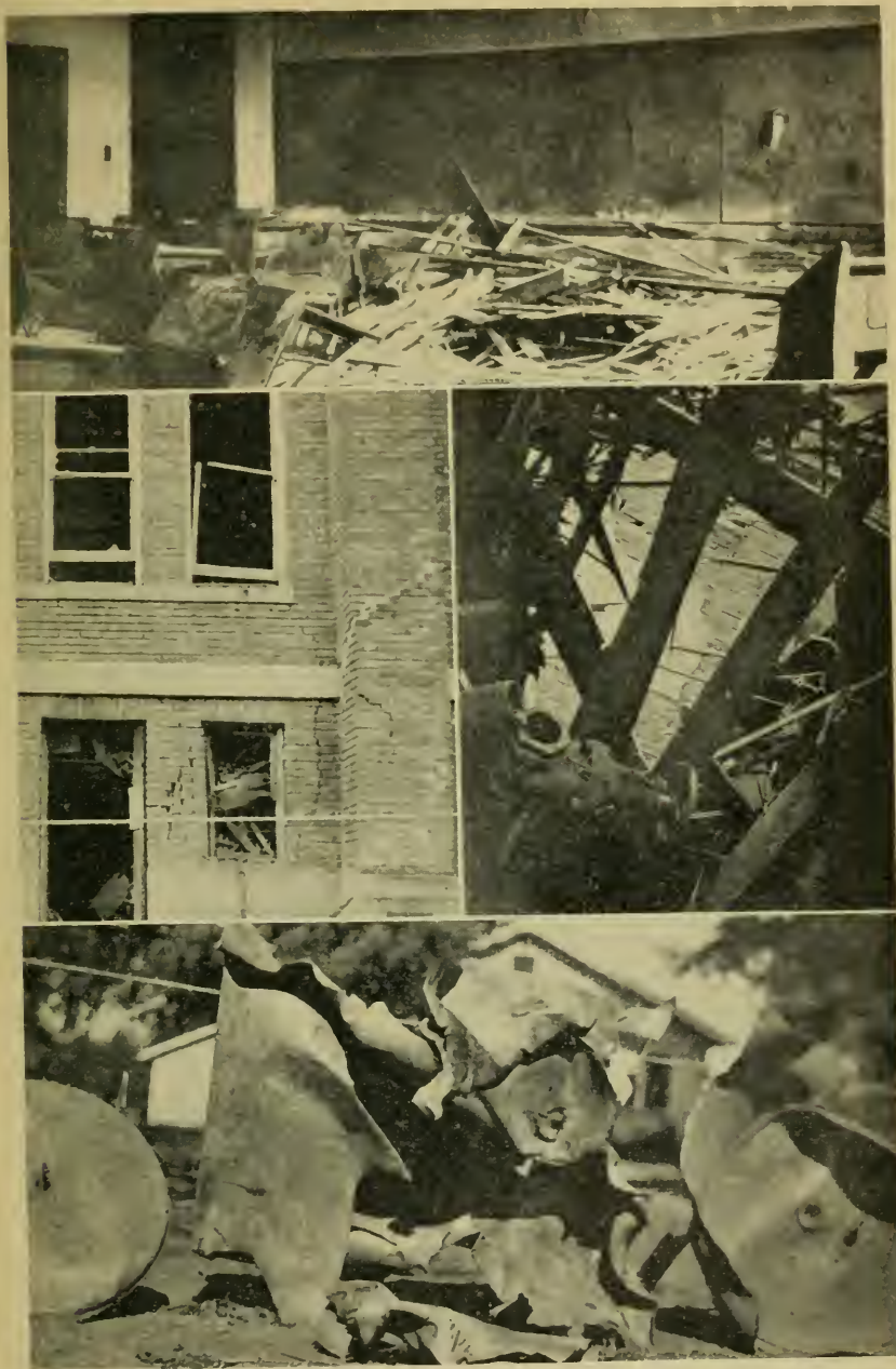
Scenes at Forest, Mississippi. Top and right center—views of the school-room floor. Left center—cracks in the building. Bottom—pieces of the tank.
