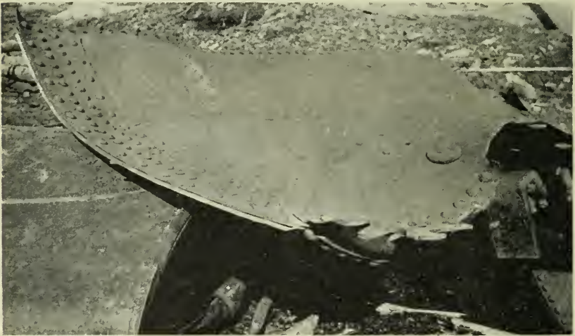
Part of the boiler plate after an explosion which killed three.
