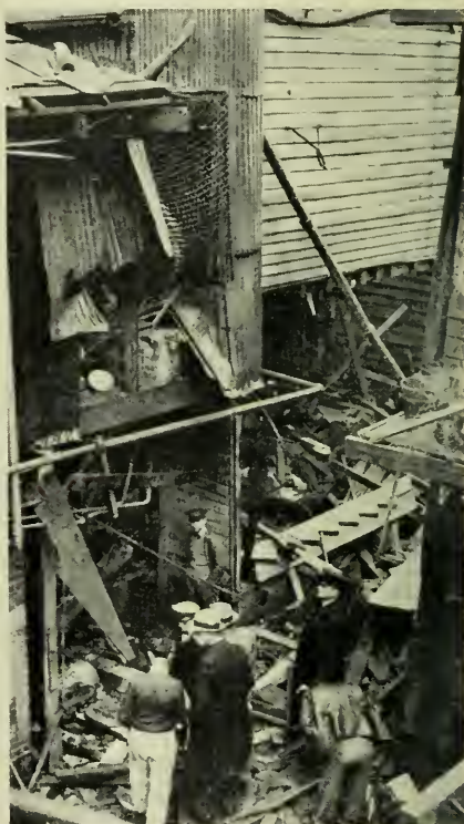
Damage following explosion of vertical tubular boiler.
