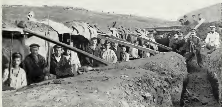
A COMPANY IN THE TRENCHES.
