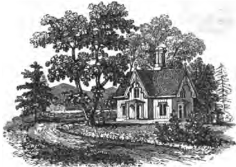
[Fig. 60. The Gardener's House, Blithewood.]
