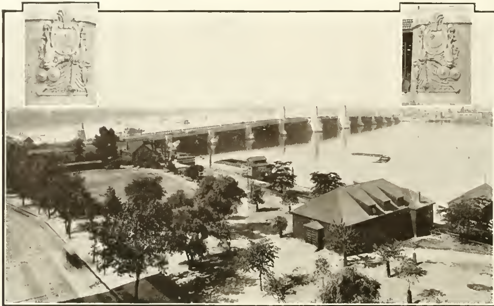
THE NEW CAMBRIDGE BRIDGE
