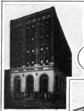
Ottawa National Bank and First National Bank, Miami, Okla. Merged shortly after construction commenced.
