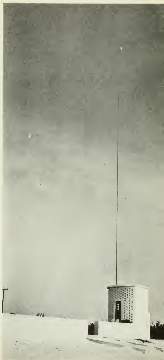
FIG. 3. The radio telephone receiving station at Tampa, Fla., for coastal and harbor service
