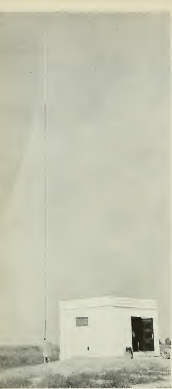
FIG. 2. The radio telephone transmitting station at Wilmington, Del., for coastal and harbor service
