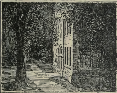
ENTRANCE, RAND HALL, NIGHT
