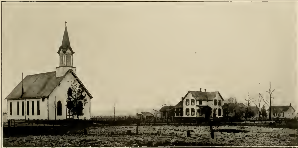
GERMAN LUTHERAN CHURCH, PARSONAGE, TEACHER'S RESIDENCE AND SCHOOL, SUGAR CREEK TOWNSHIP
