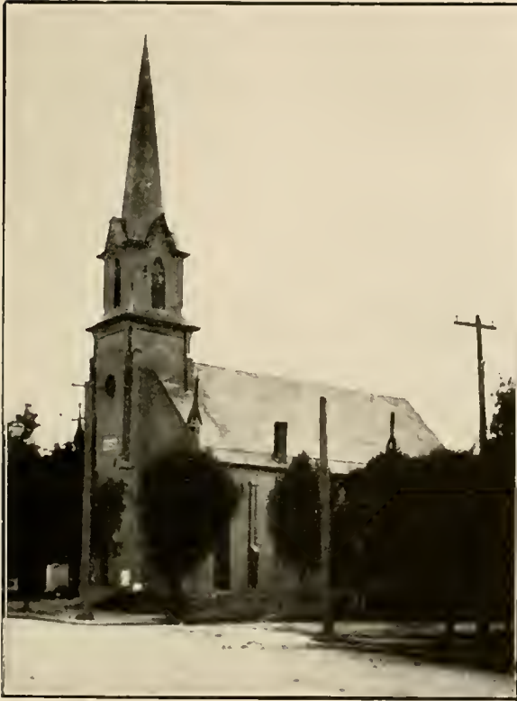
OLD PRESBYTERIAN CHURCH, GREENFIELD
