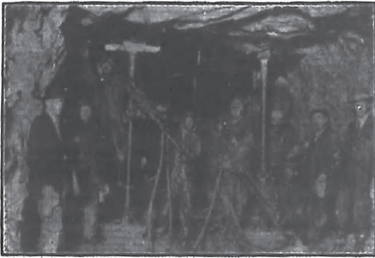
(43) Leyner-Ingersoll Drills in Rogers Pass Tunnel of Canadian Pacific R. R., at Glacier, British Columbia. A new American Tunneling Record, 932 feet per Month, was established here during January, 1915.
