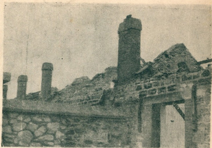
(4) 被毀之張家莊站員司住宅 The destroyed Staff Quarters at Chang Chia Chuang Station
